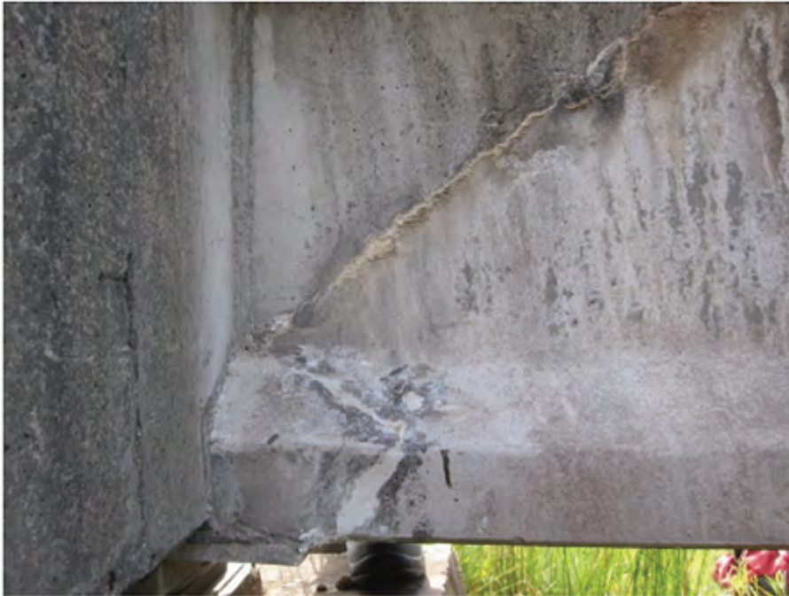
Figure 2-7 Crack repair at pier 9 (refer defect 1)
