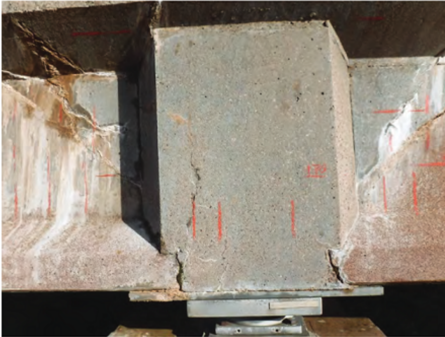
Plate 8 – General view of surface markings to Pier 9 Right Beam up/down.
