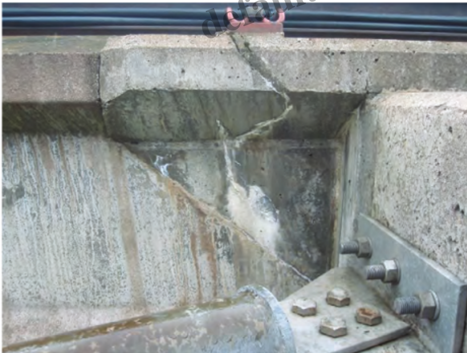
Figure 2-6 Cracking at a pier 9 (refer defect 1)
