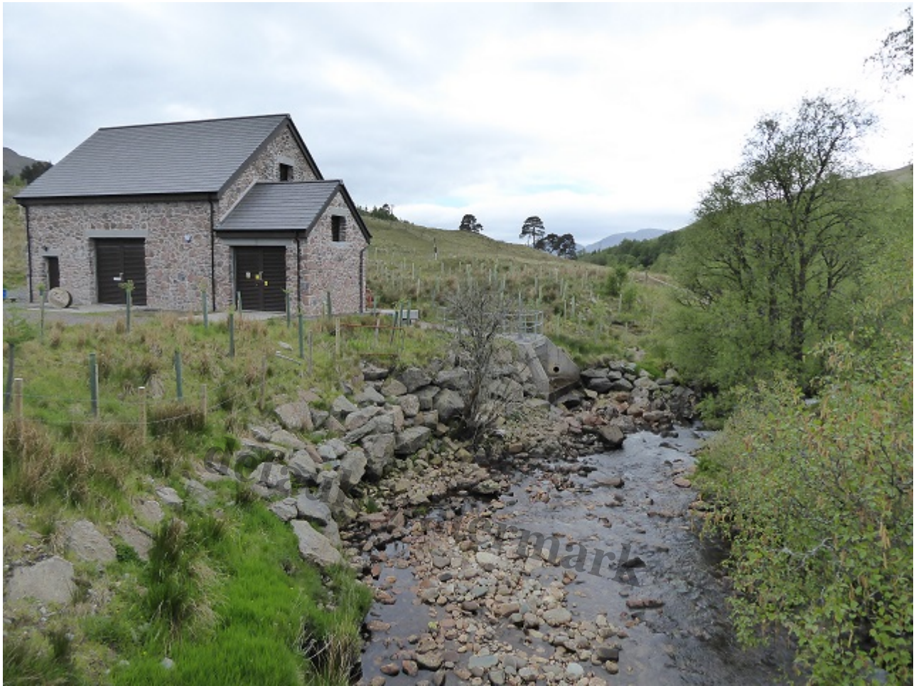
Upper Glen Falloch hydro scheme turbine house, surrounded by plastic tree tubes next to the river
