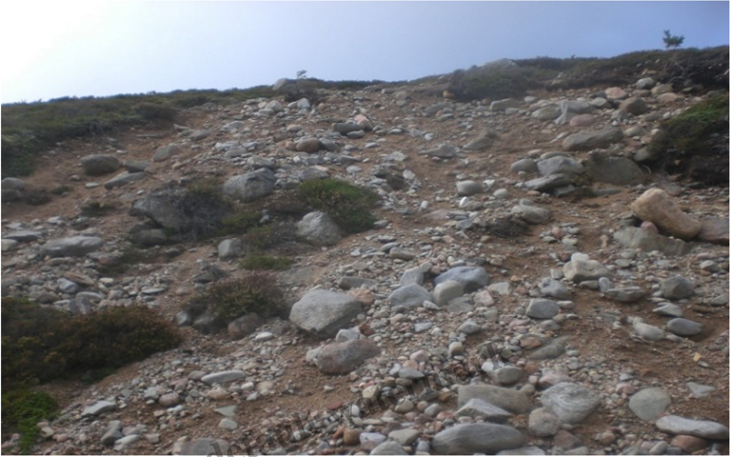
Collapsing hillside above the path.
