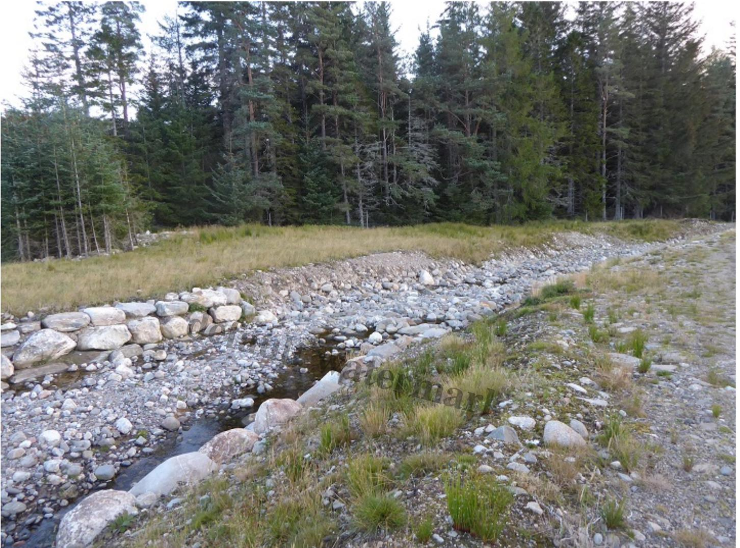
The design flaws and the problems they have caused are only two apparent as soon as you look beyond the rip rap bouldering below the entrance to the overflow. A shortish section of bank has collapsed, leaving earth vulnerable to erosion.
