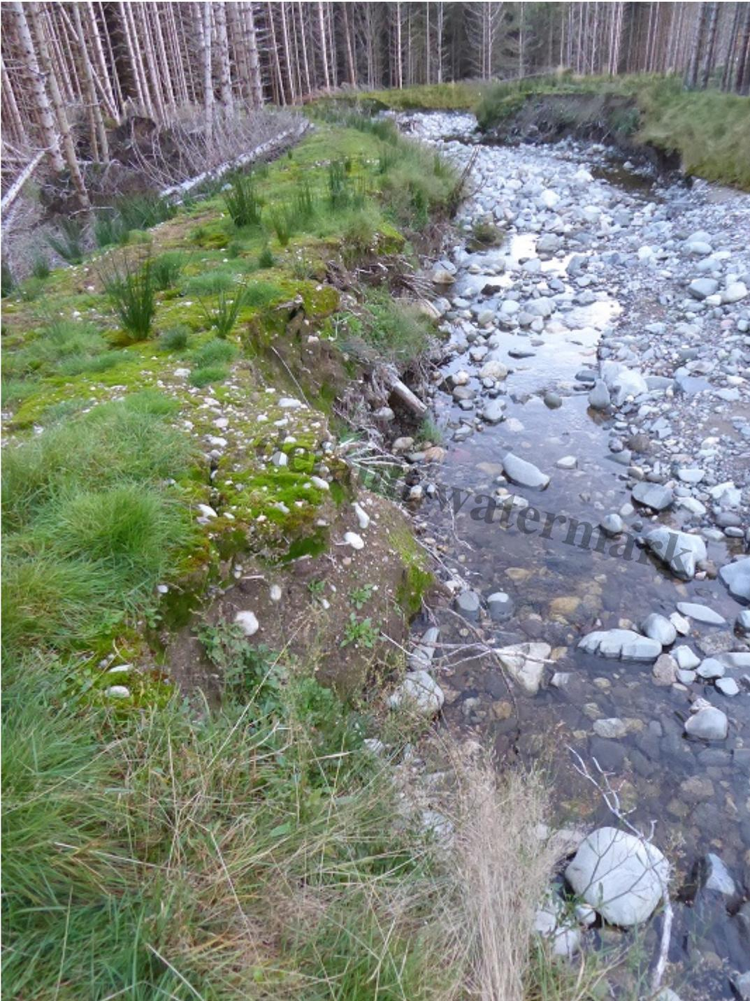
Lower down, what were bare earth banks have greened up slightly. But take a careful look and you can see how they are continuing to erode. If any volume of water was to run down the overflow, these banks would be swept away in no time at all.
