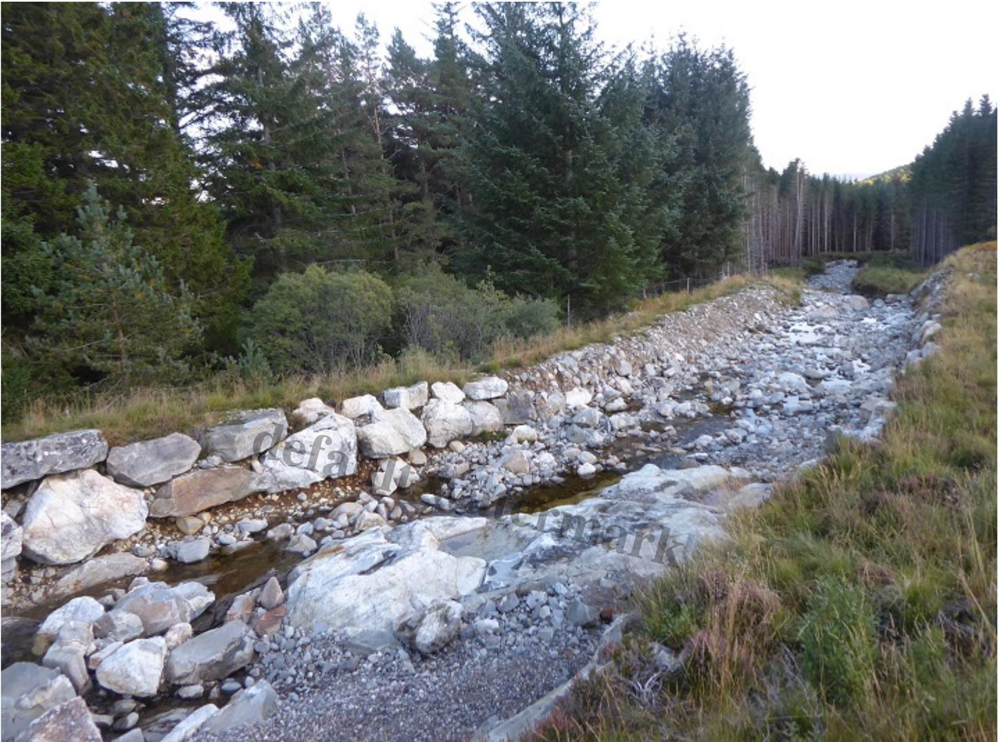
Some sections of rip rap bouldering appear poorly designed, with giant boulders sitting on earth vulnerable to erosion. It seems that almost the entire overflow channel will, if it is ever to function properly, require to be re-built. Highland Council contributed Â£135k to this project â?? for what?
