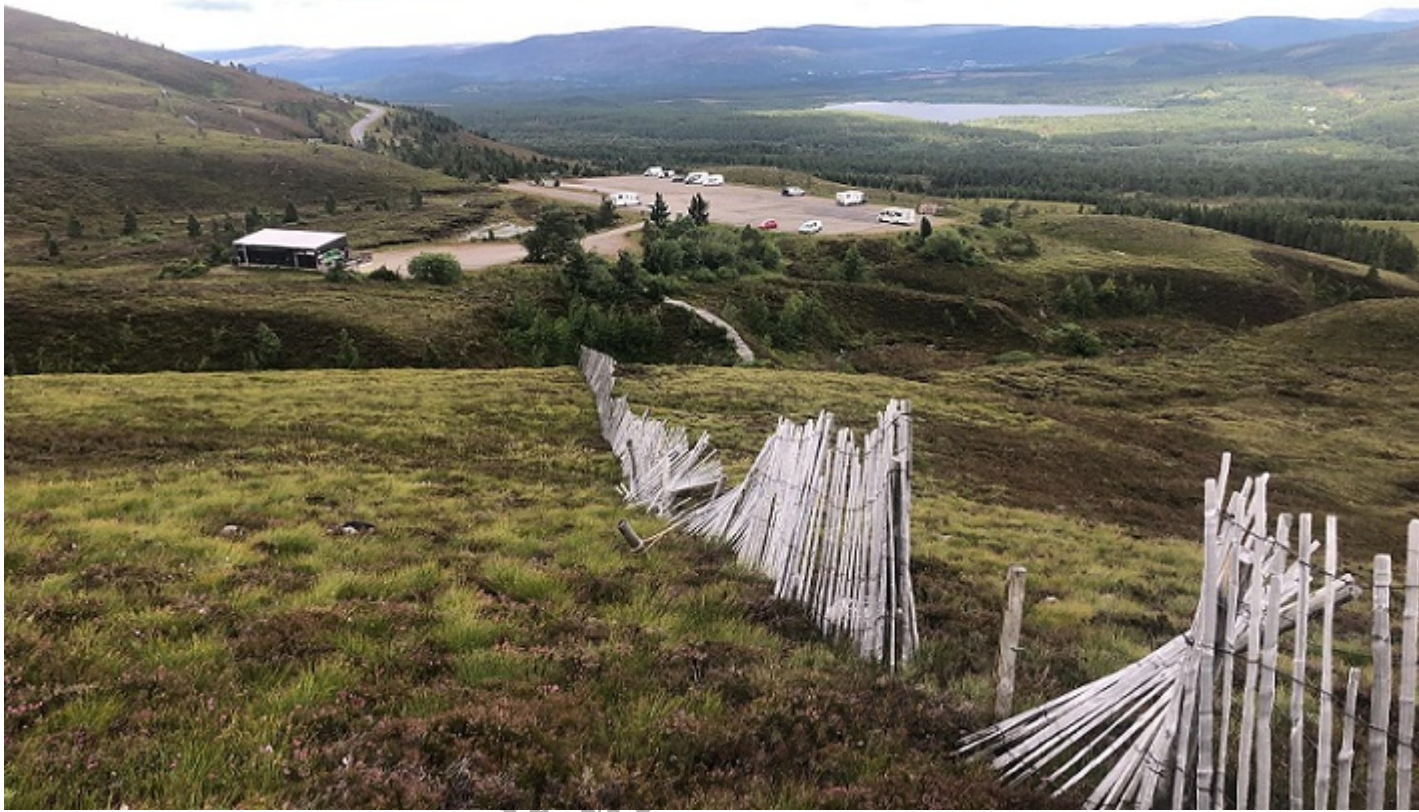
The Laogh Mor Return fencing in a state of disrepair as it is further into the Coire. Photo credit Alan Bratney Autumn 2020
