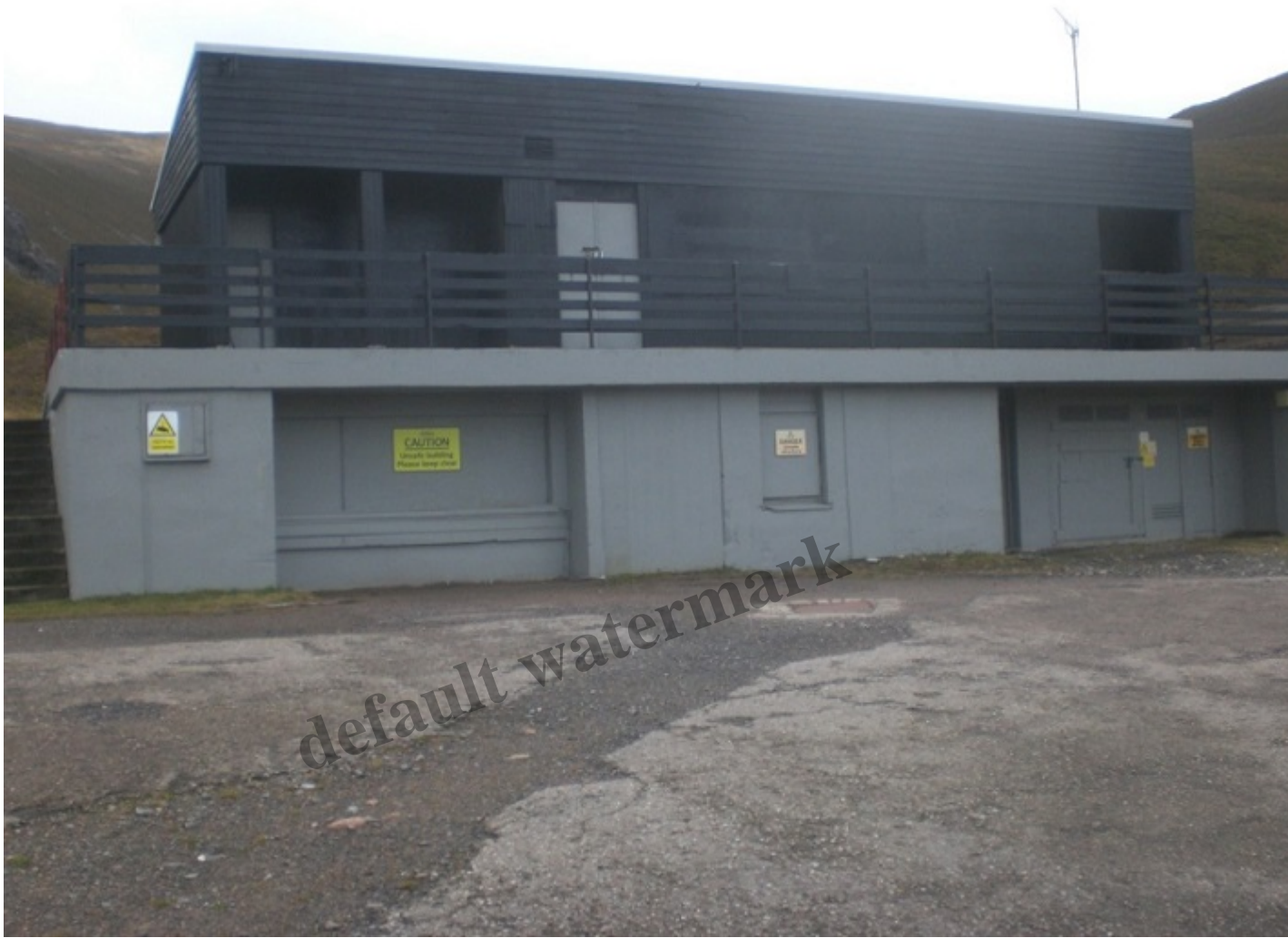
The Ciste base station building. Photo credit Alan Bratley Autumn 2020
