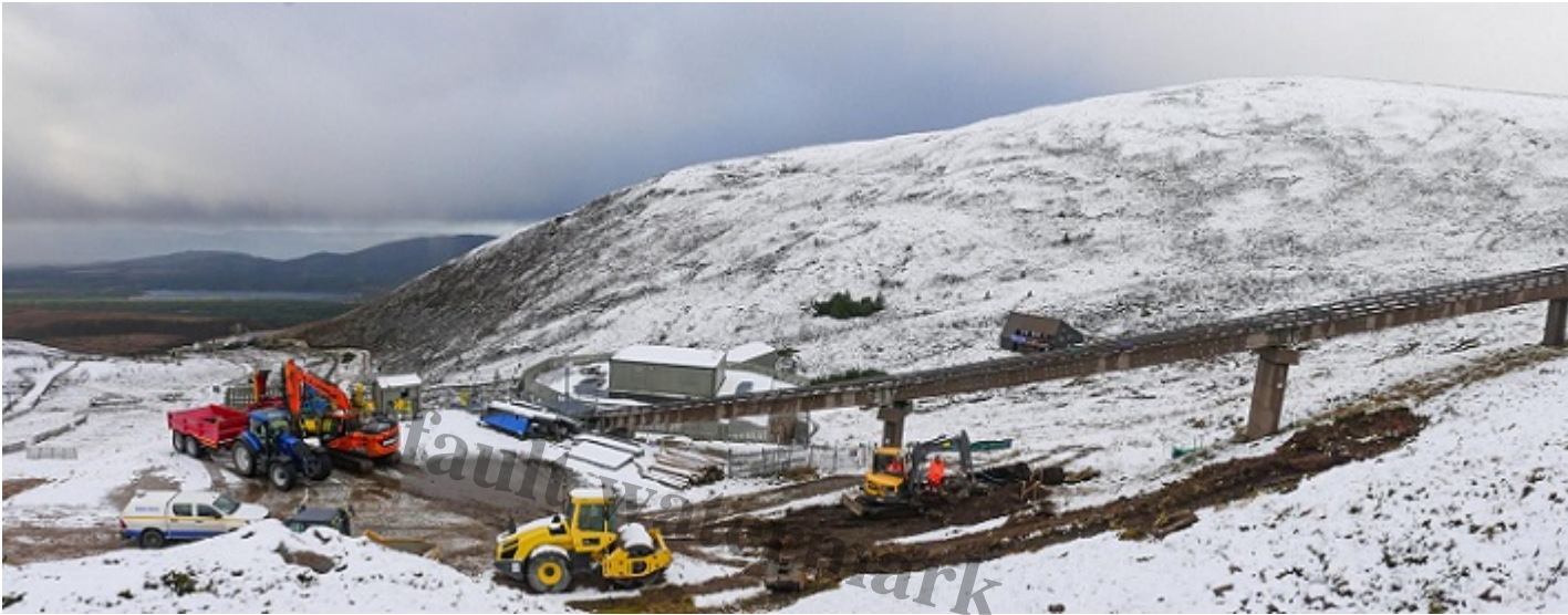
View of the repair works from above the mid-station, with compound on left and pillars 51,52 and 53 visible
