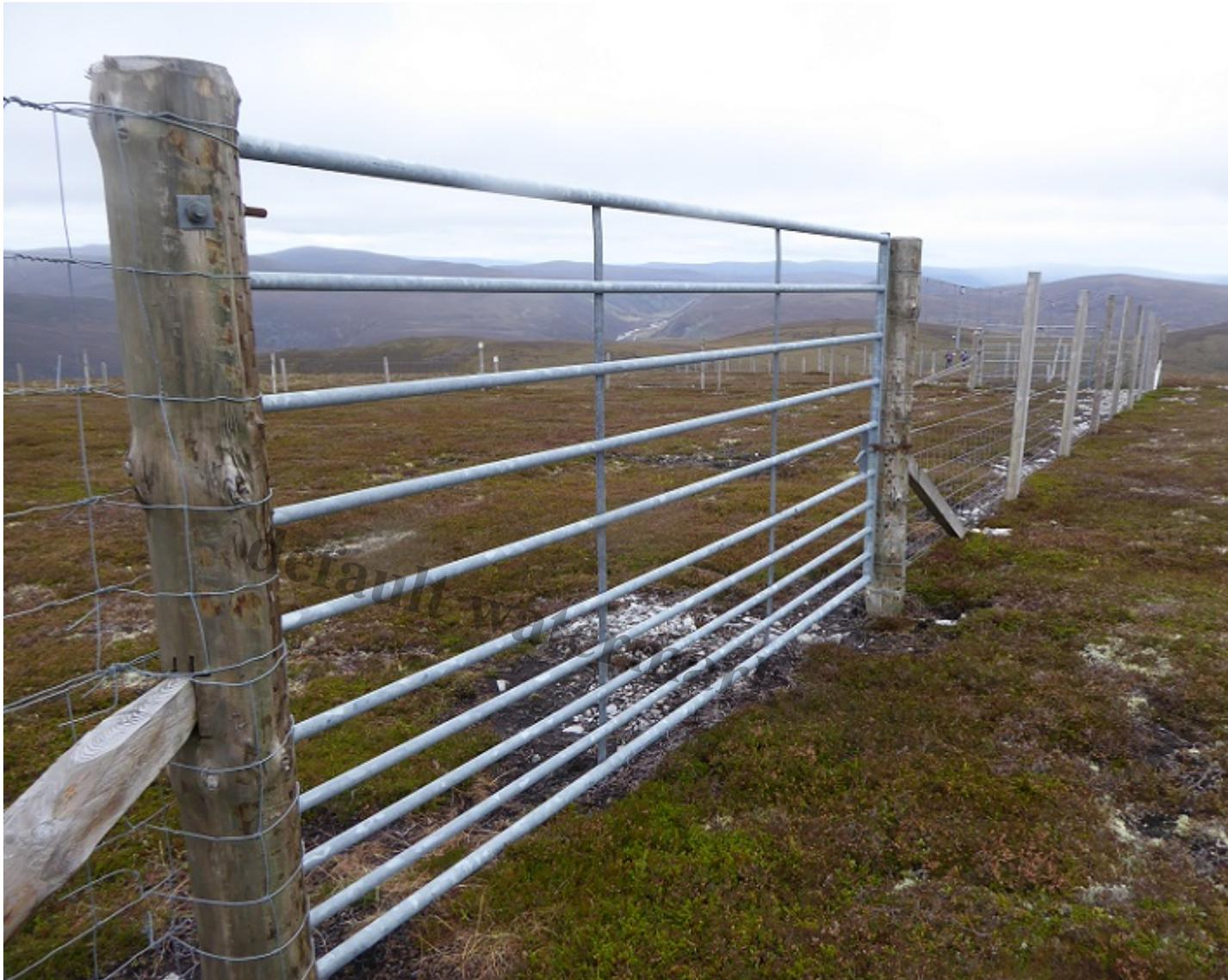
Junction of the traditional deer fence separating Invercauld and Delnadamph with the electric fence, erected by the Glen Avon estate beyond.
