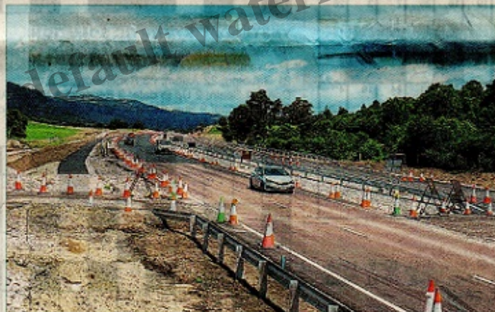
Dualling work on the A9. Picture: Glen Wallace
