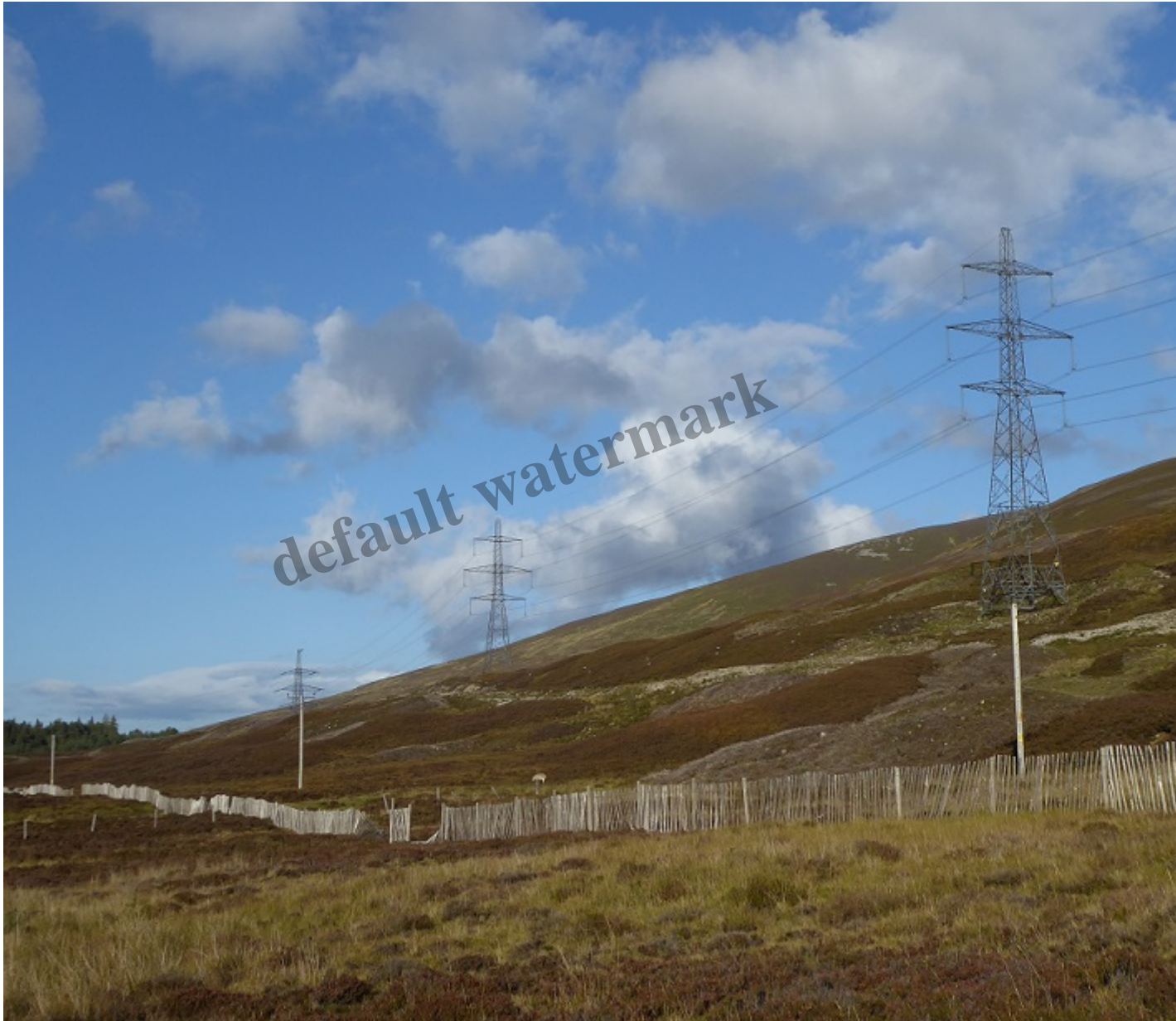
The Beaully Denny powerline and construction track scar. North Drumochter Lodge is in the woods in background. September 2020.
