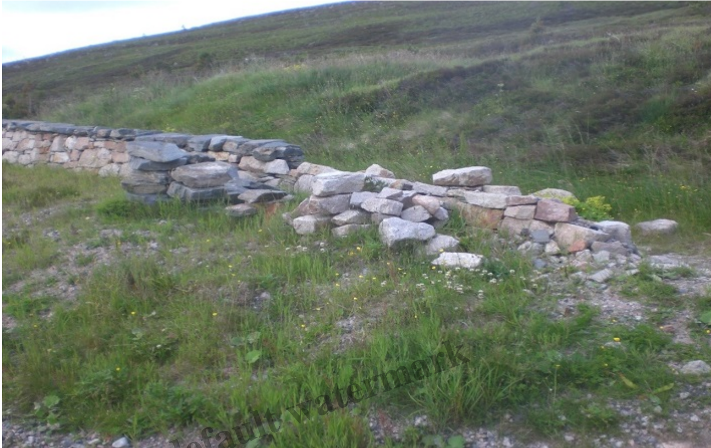
Collapsed stonework. Picture sent to HIE
