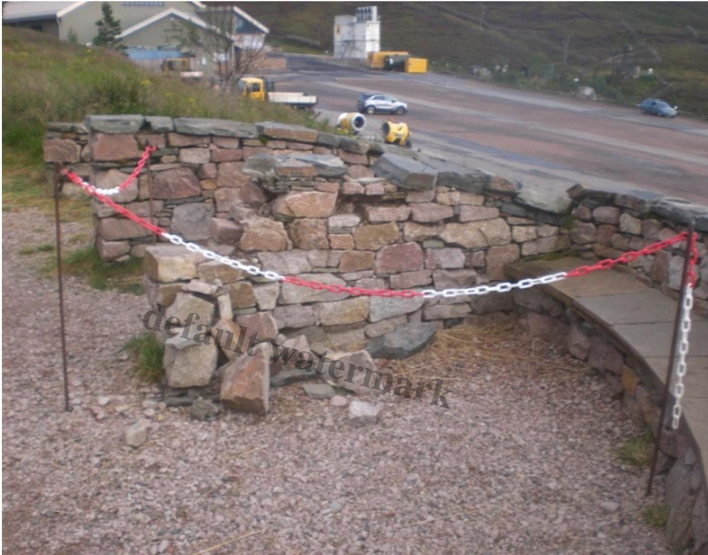
The dangerous section: taken down and roped off [no hazard signage though]
