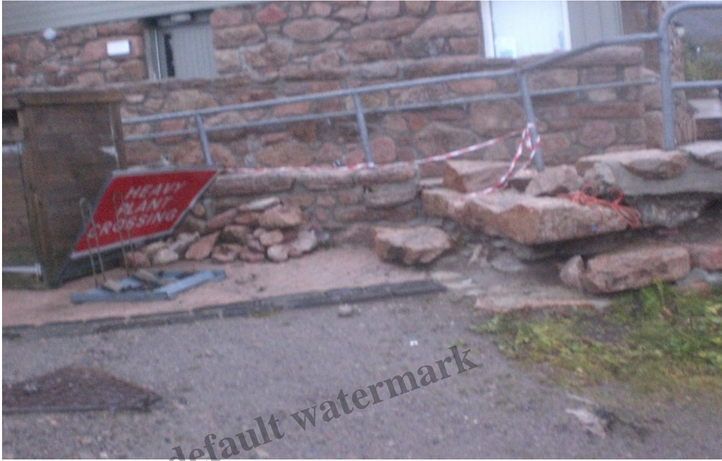
The wall next to the Daylodge.
