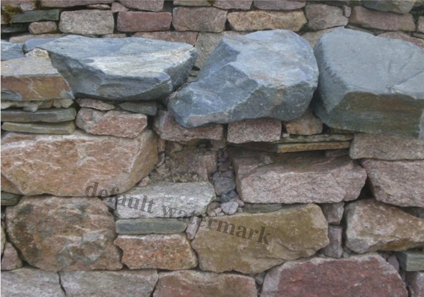
Picture of the missing stone which could have led that section of wall to collapse under the weight of childâ?!.sent to HIE
