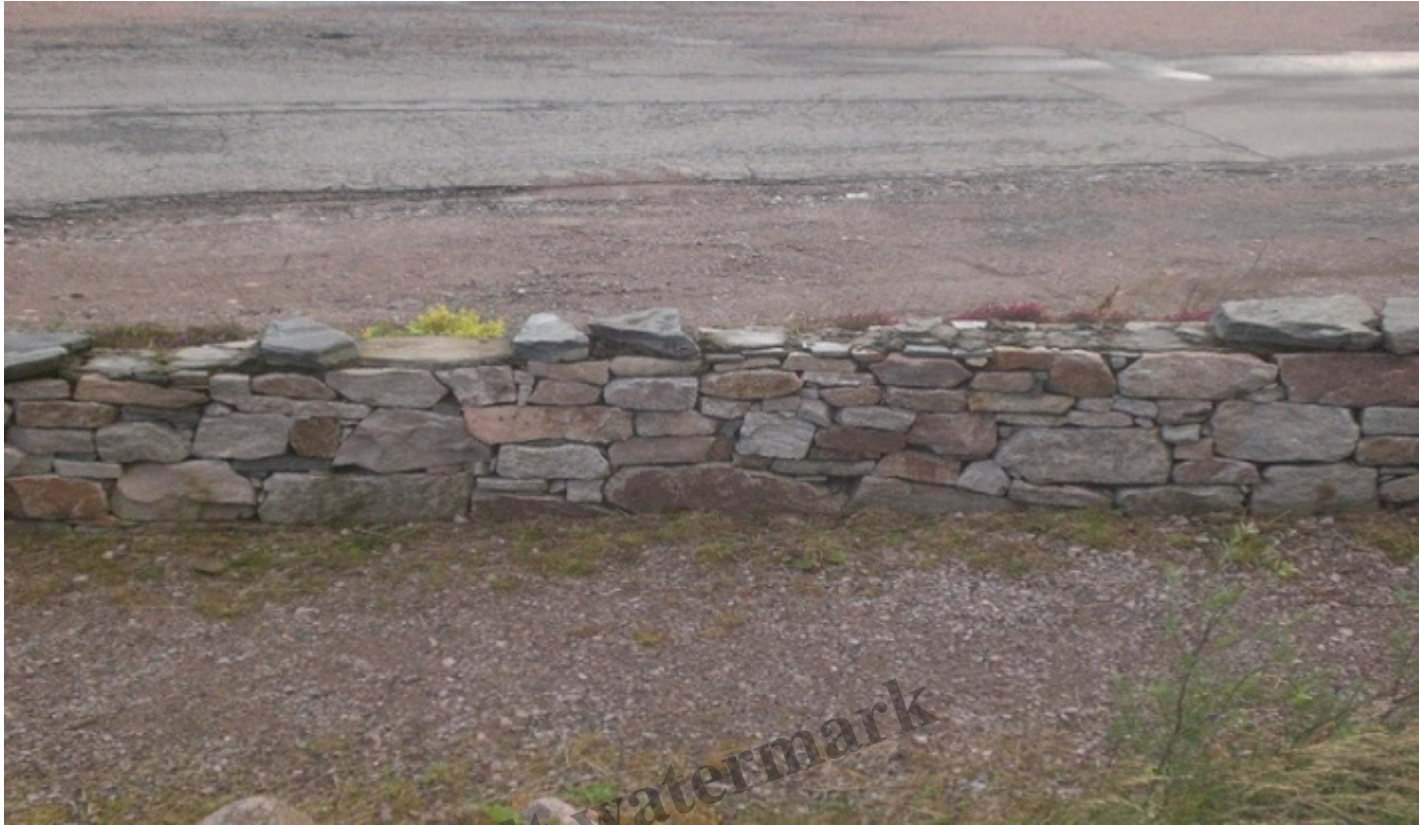
Loose Cap stones removed
