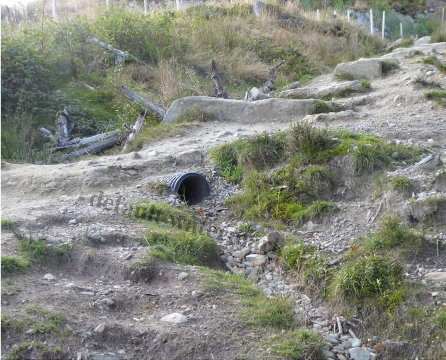
And viewed from closer up. Note how some of the former steps have become isolated islands of rock how much of the surface has been eroded from the top of the pipe
