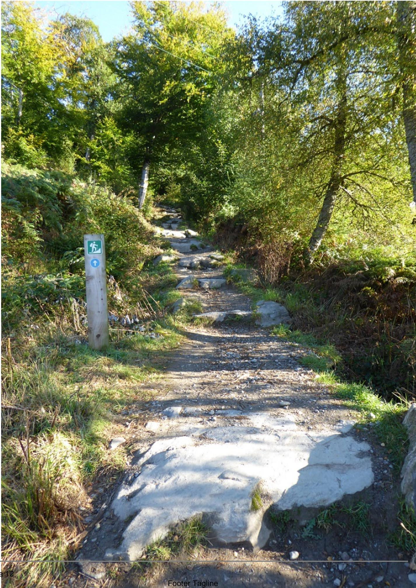
Note the signs of water erosion on the sections between the steps and the rocks on either side of each step, designed to prevent people walking round the edge.
