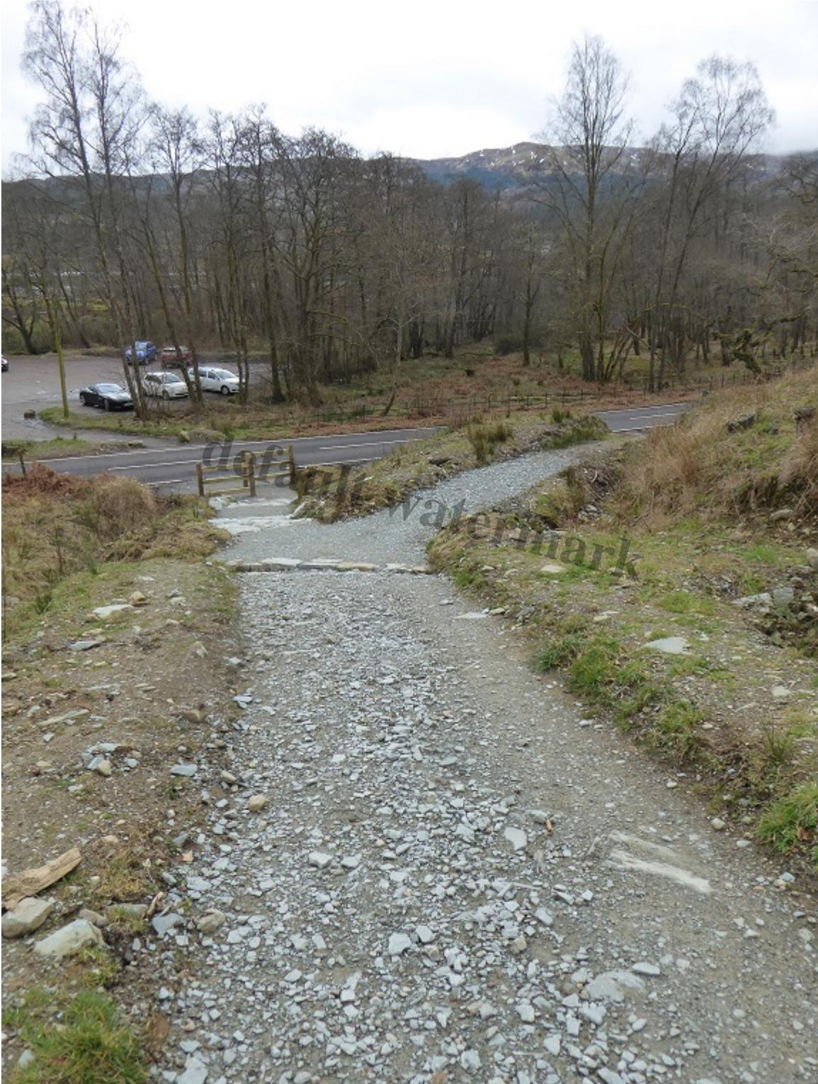
Tell tale signs of water erosion, not far above the steps, the fine material has been washed out from the left hand side of the path
