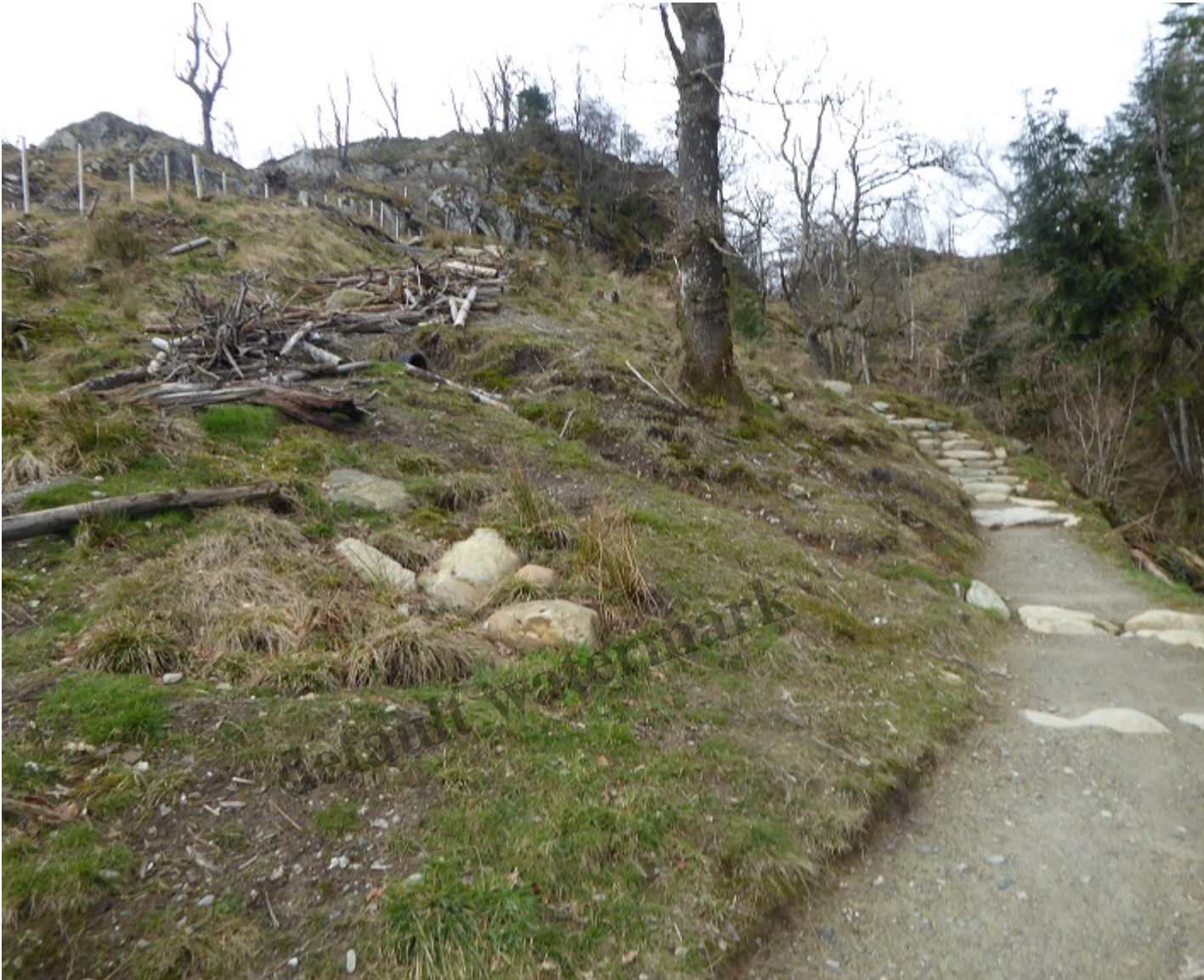
March 2019. Note the plastic culvert at the top of the obvious drainage ditch. The original new route directly up the hillside to the left of the large tree in the centre.
