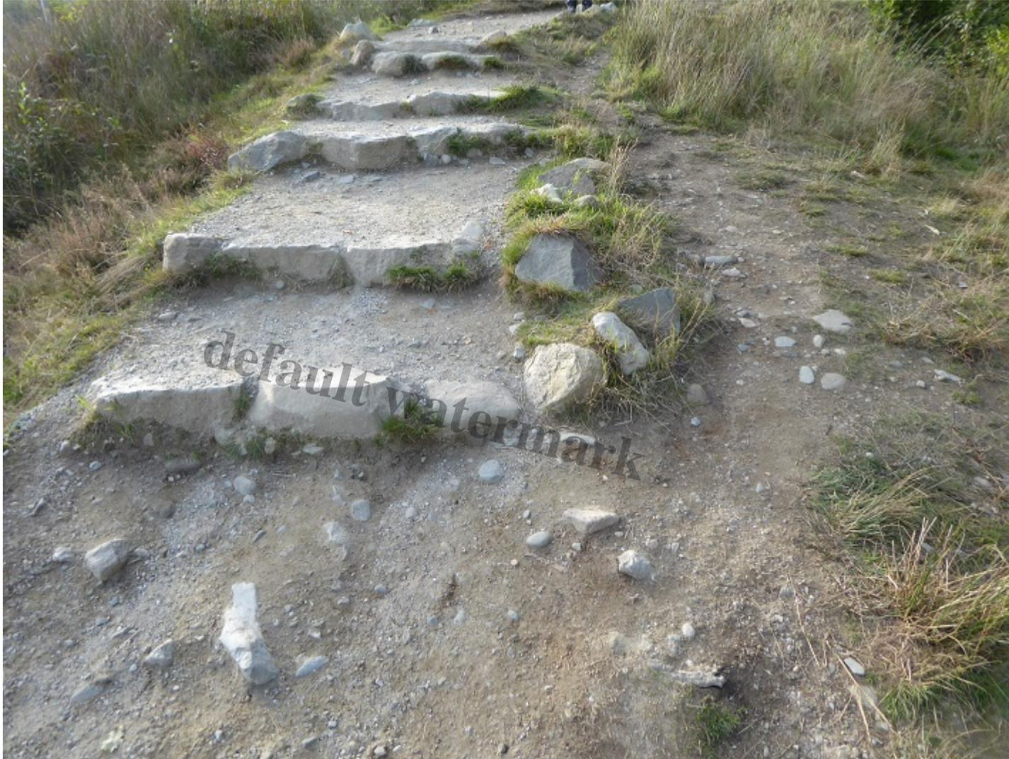
Clear signs of how the ground below the bottom step has eroded.
