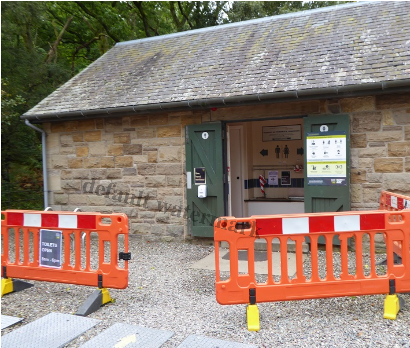
LLTNPA toilets at Milarrochy Bay
