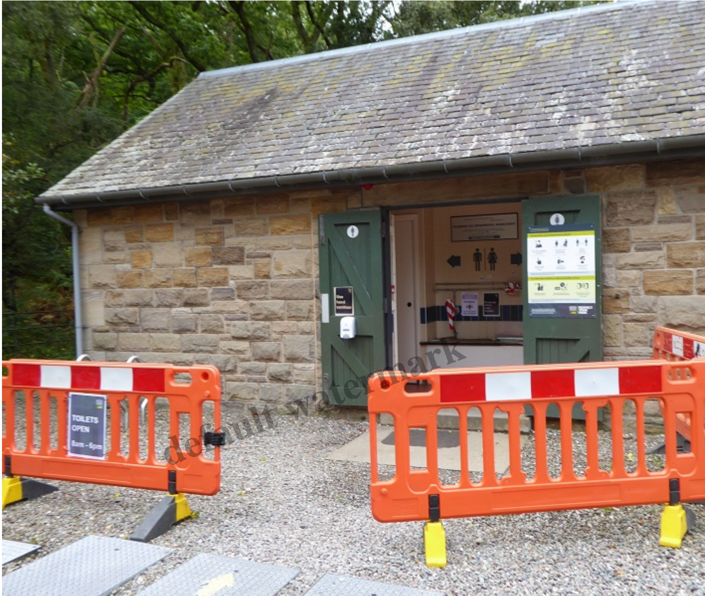
LLTNPA toilets at Milarrochy Bay
