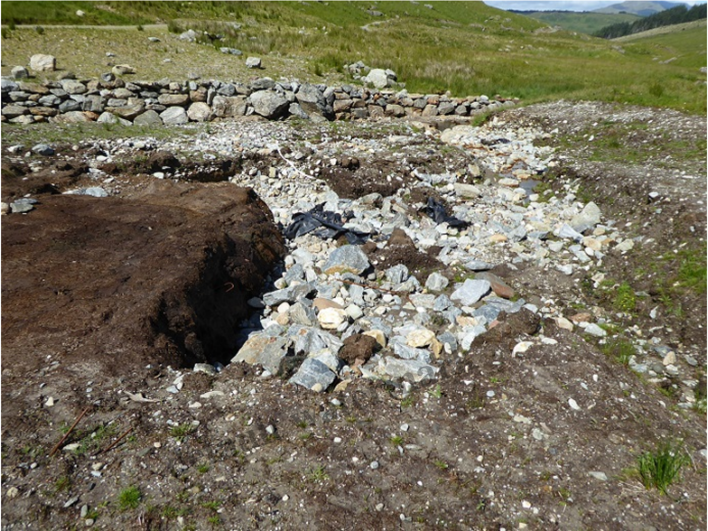
Looking down one of the new channels created by the flood over to far bank of the River Falloch below the intake. A large area of “restored” peat just waiting to be swept away.
