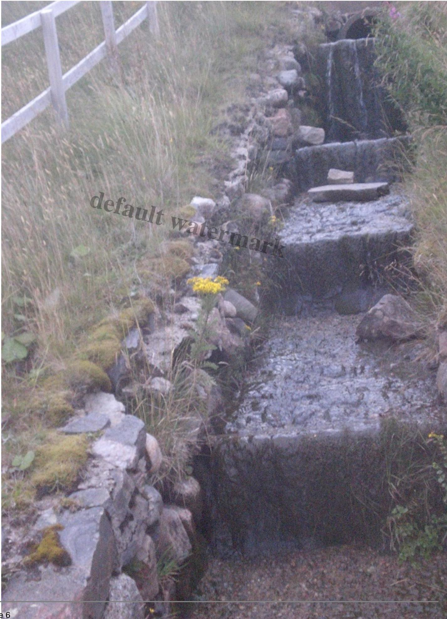
Lower Cas Car park: Drainage Channel with collapsing side walls.
