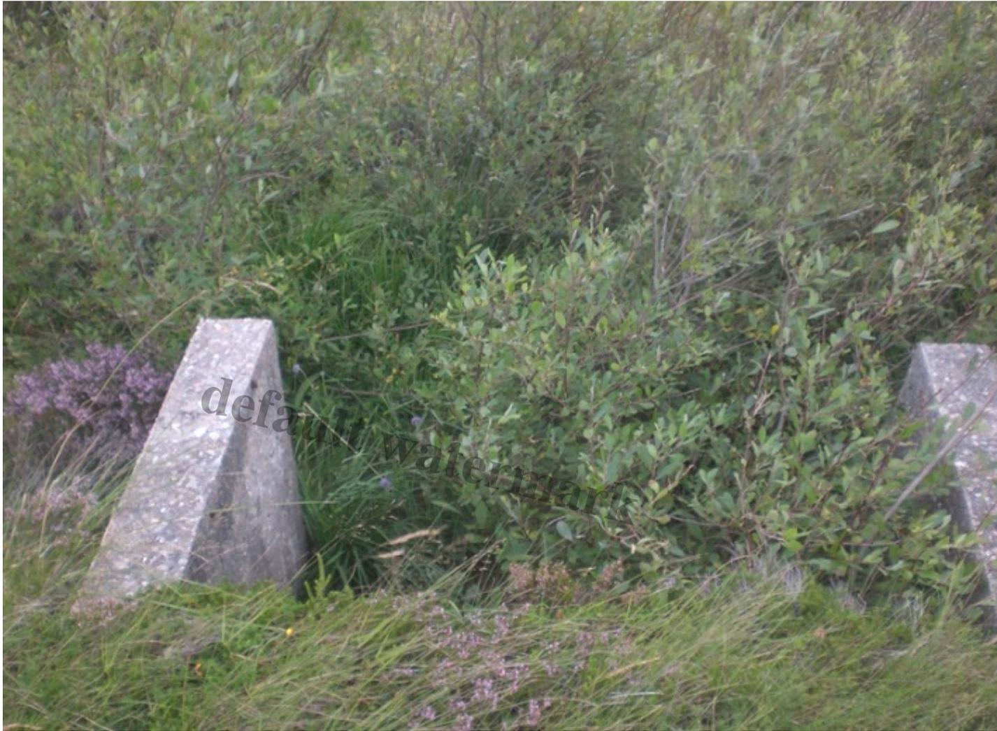
Link Road: Drainage outflow gully. Completely overgrown â?? eventually this could undermine the road
