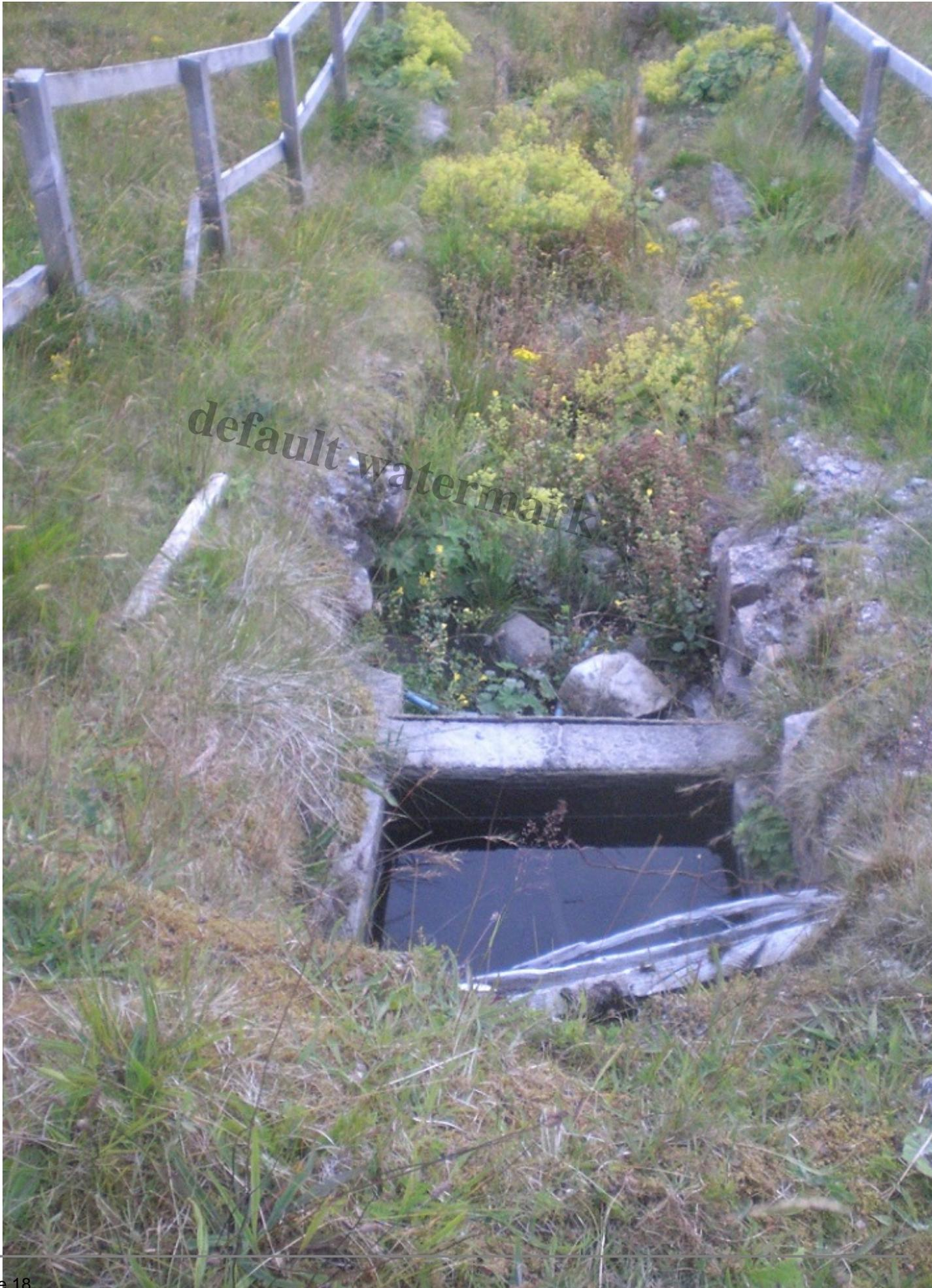
Link Road: Drainage outflow gully. Completely overgrown.
