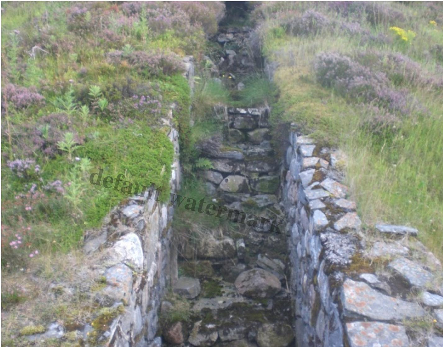
Link Road drainage channel. Unmaintained and as a result starting to fall to pieces.
