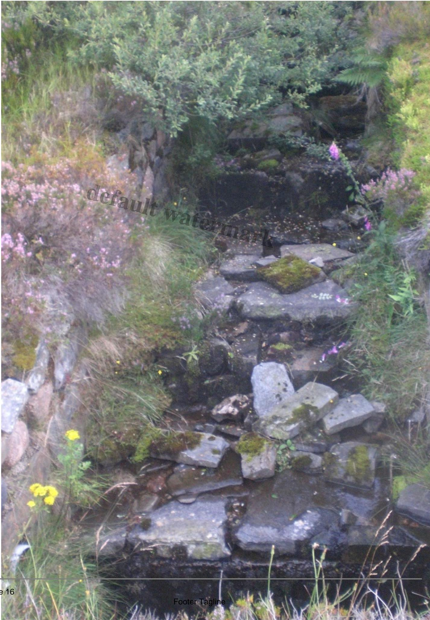
Link Road Drainage Channel: In a state of collapse.
