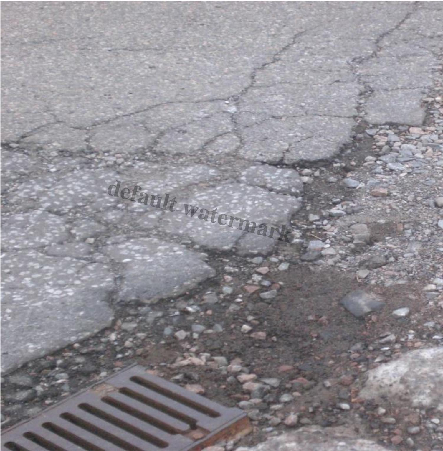
Two weeks after re-opening the car park and the result is clear. Car tyres have already removed some of the rubble, a hole has appeared and the next section of metal drain covering is now hazardous to car tyres.
