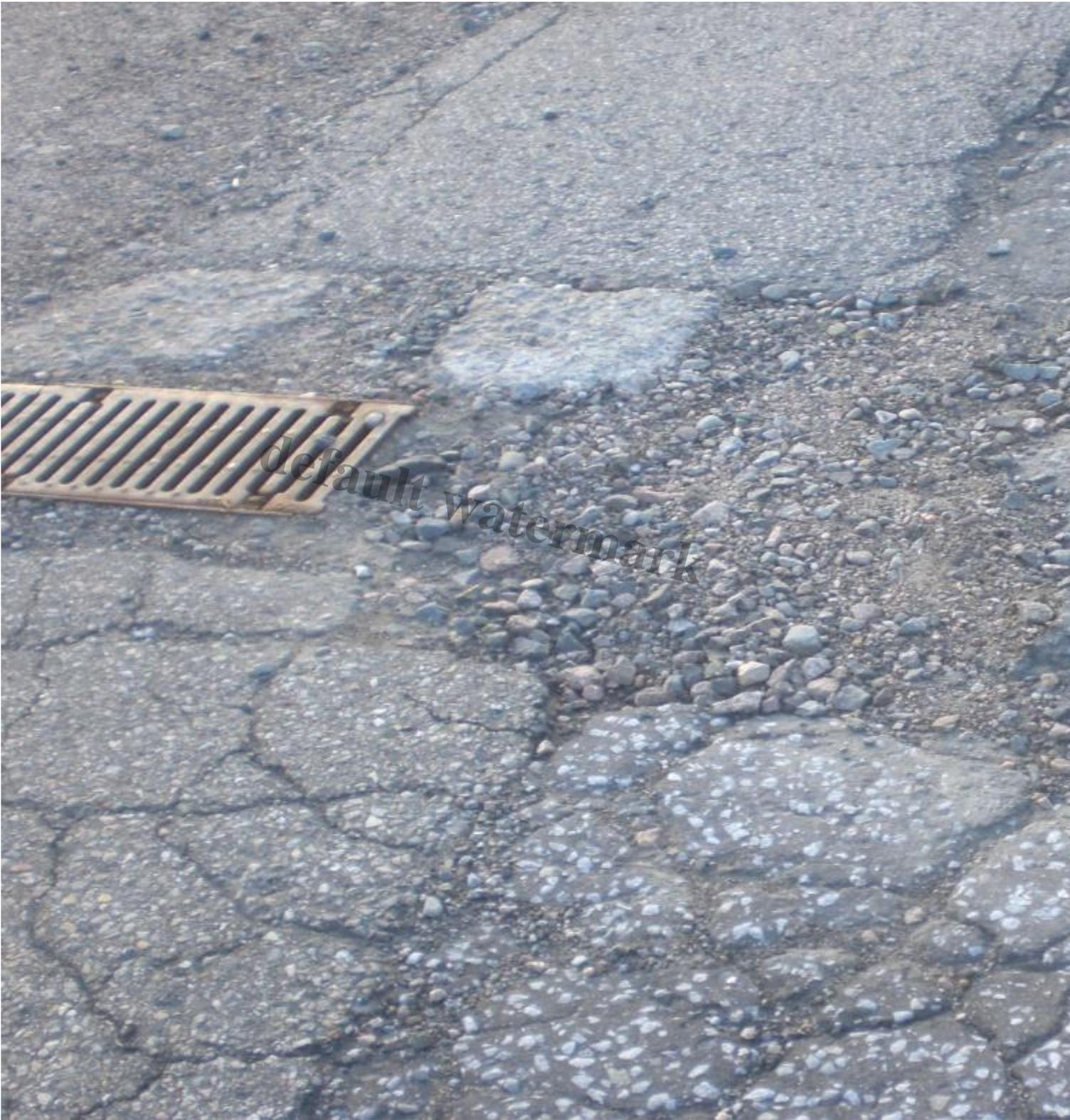
The metal drain cover was removed during the lockdown period and the hole filled with rubble.
