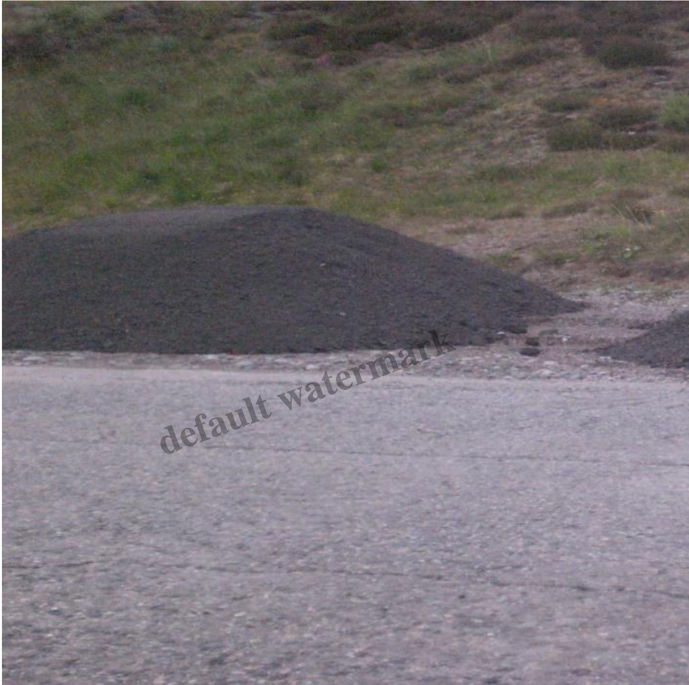
A couple of small piles of screeding material which consists of old roadway surface which has been p
