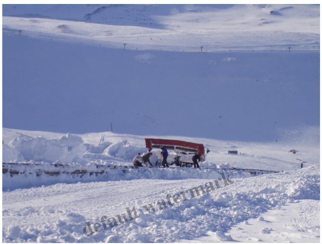
Snow burial of the track and subsequent digging out may have contributed to the funicular's structural issues. The proposed repairs though modest in comparison to the scale of the viaduct will nonetheless exacerbate problematic snow accumulation at the funicular viaduct.
