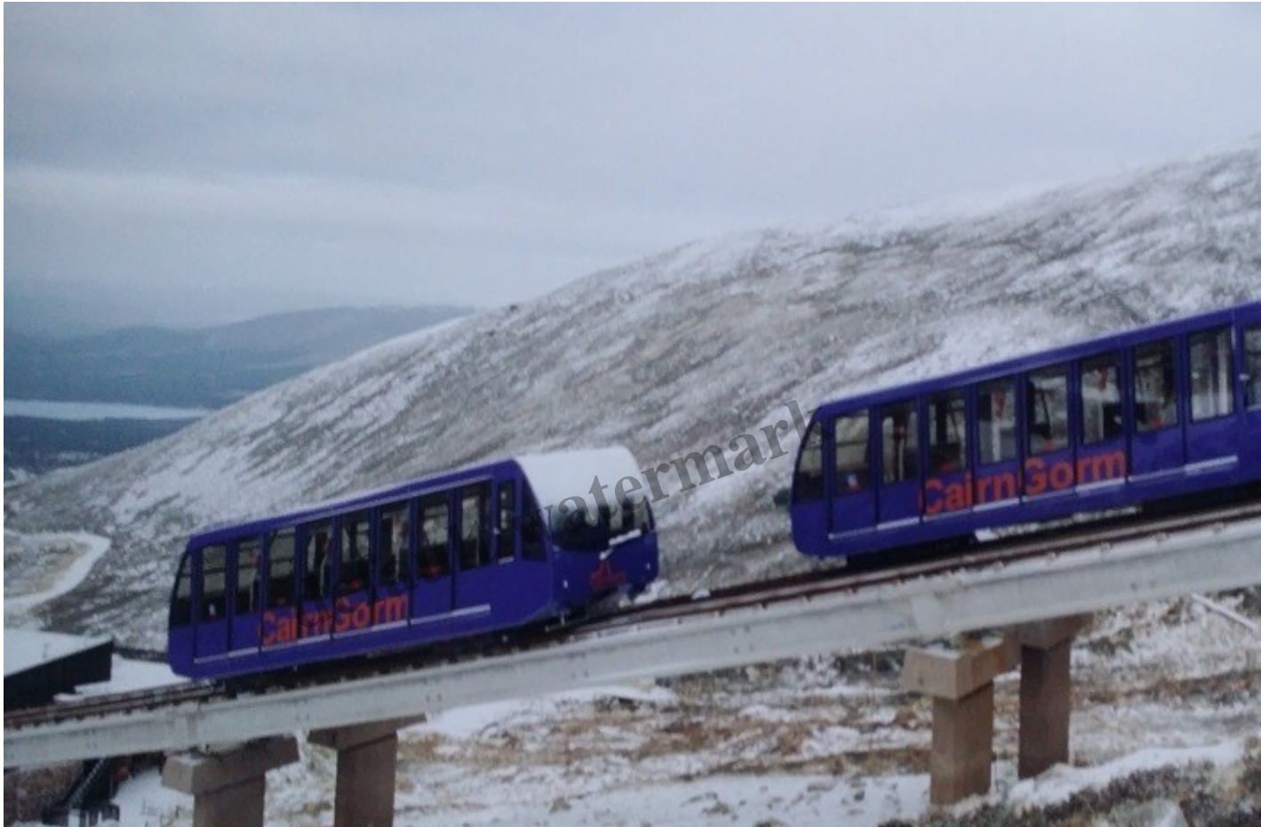
Funicular Carriages at the passing loop which is uphill from the mid-station upload/download area
