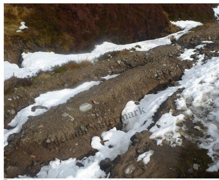
The eroded wheel ruts are now so deep as to make the track impassable to almost any vehicle
