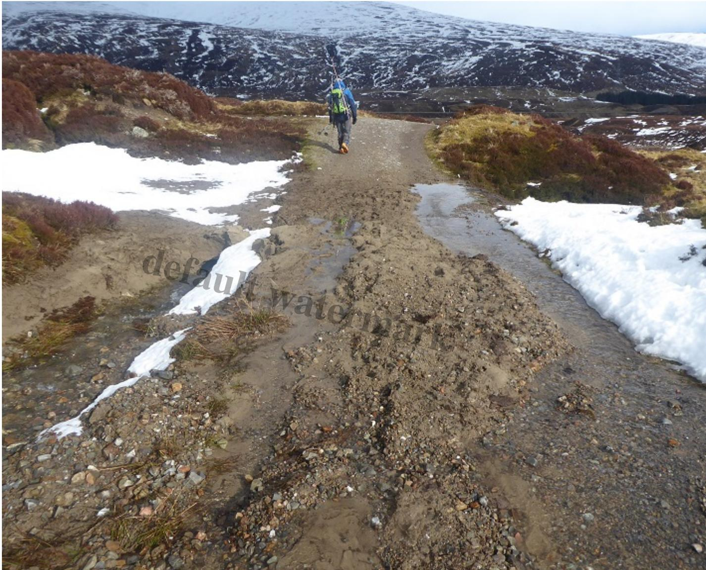
Eroded silt and other material washed down to below the steeper section. Note the depth of silt to the ditch
