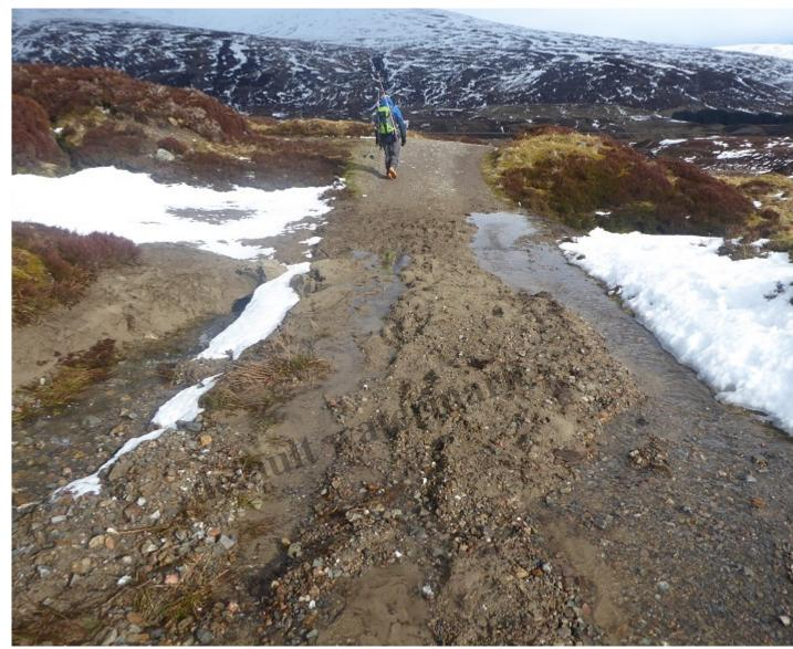
Eroded silt and other material washed down to below the steaper section. Note the depth of silt to the ditch
