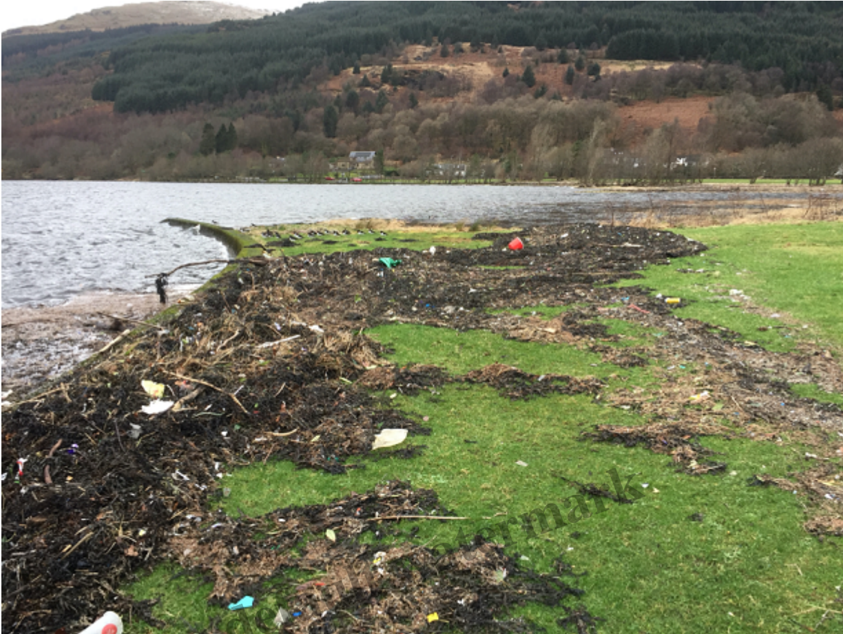
View west towards the Cobbler Carpark, showing the ramp in the foreground, originally intended for launching boats, during a previous attempt to enhance shoreline for recreational purposes. Probably seldom if ever used. Now allows vehicular access to beach. Photo credit Nick Halls 14th January 2020.
