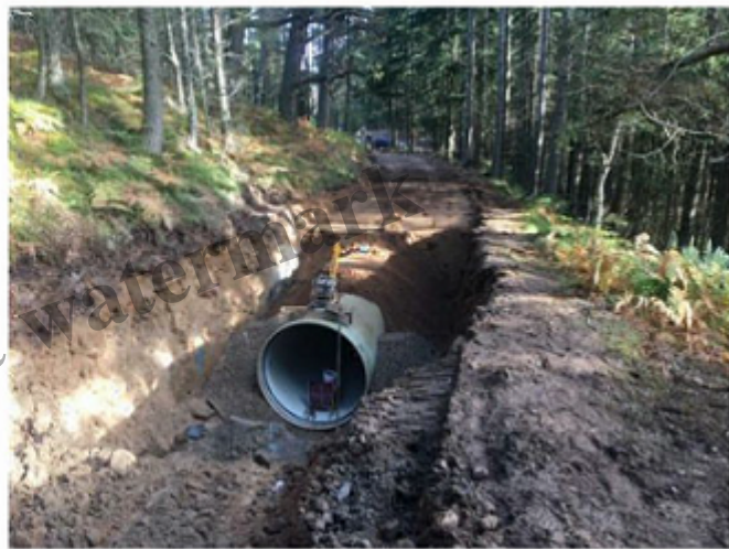
Photos 5-7: pipelaying activities – trench excavations & materials being transported by dumper
