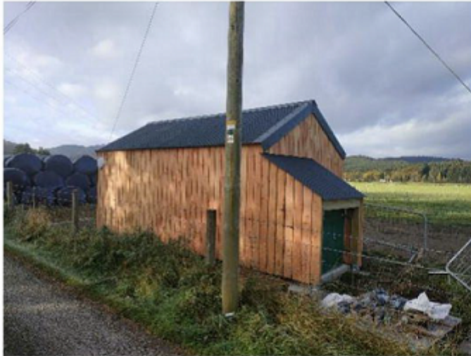
Photo 26: substation with cladding and roof in place.
