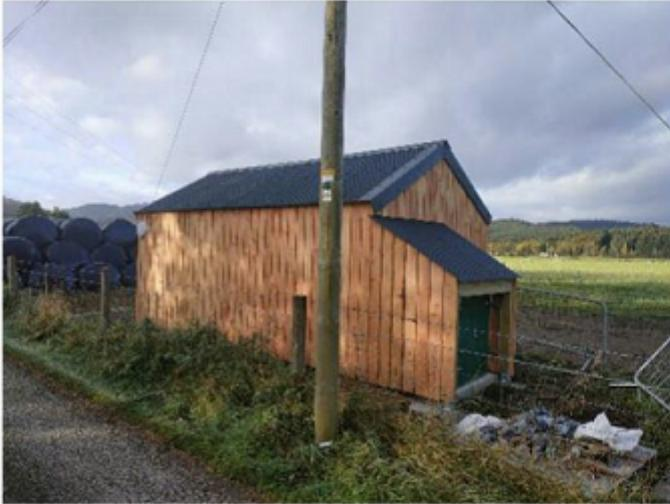
*Photo 26: substation with cladding and roof in place.*
