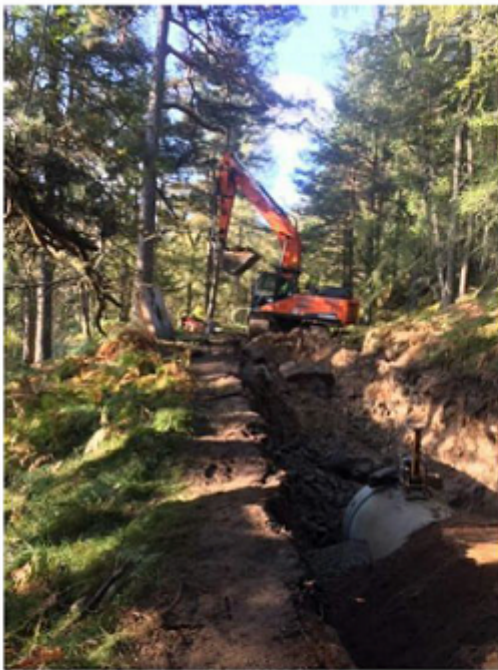
Photos 5-7: pipelaying activities – trench excavations & materials being transported by dumper
