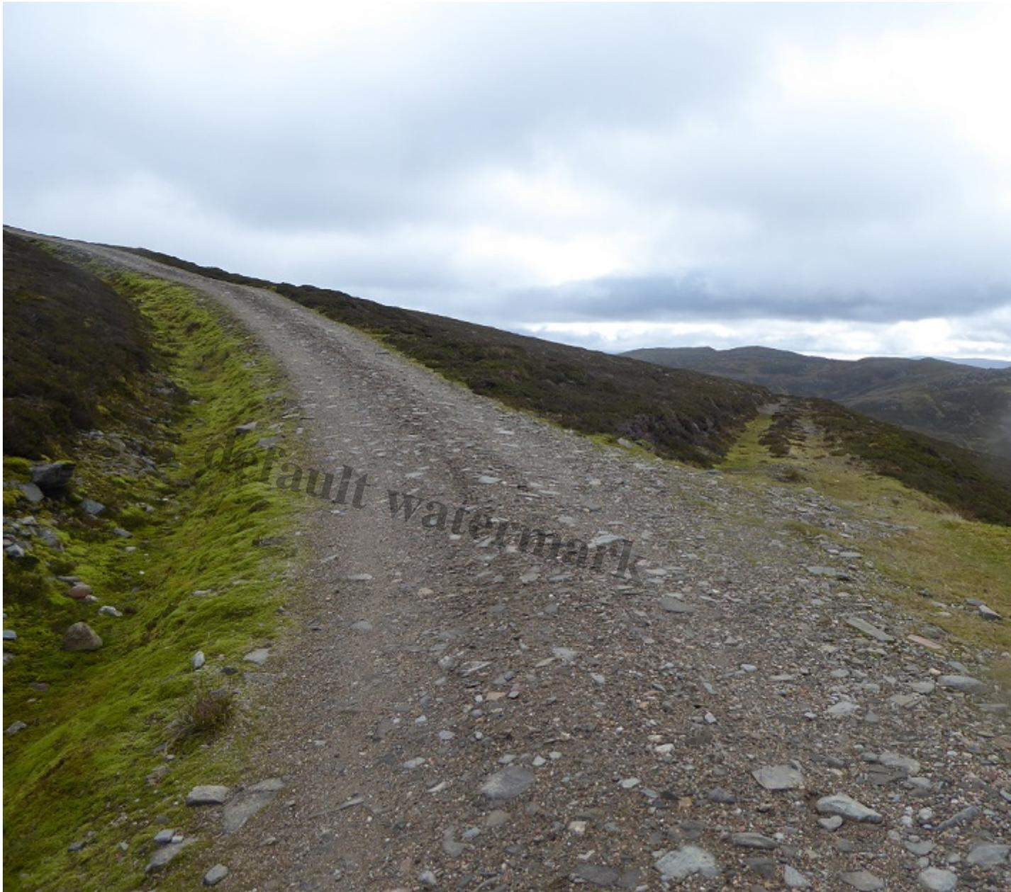
The failure to restore any vegetation in the drain on the left and the lack of any vegetated strip down track adds, completely unnecessarily, to the amount of water roads like this channel off the hill
