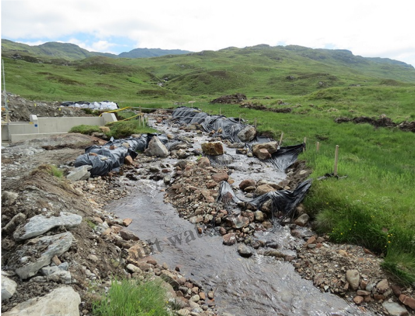
Diversion channel dug through peatland to construct hydro intake 2016. Note the piles of turf and peat to the right.
