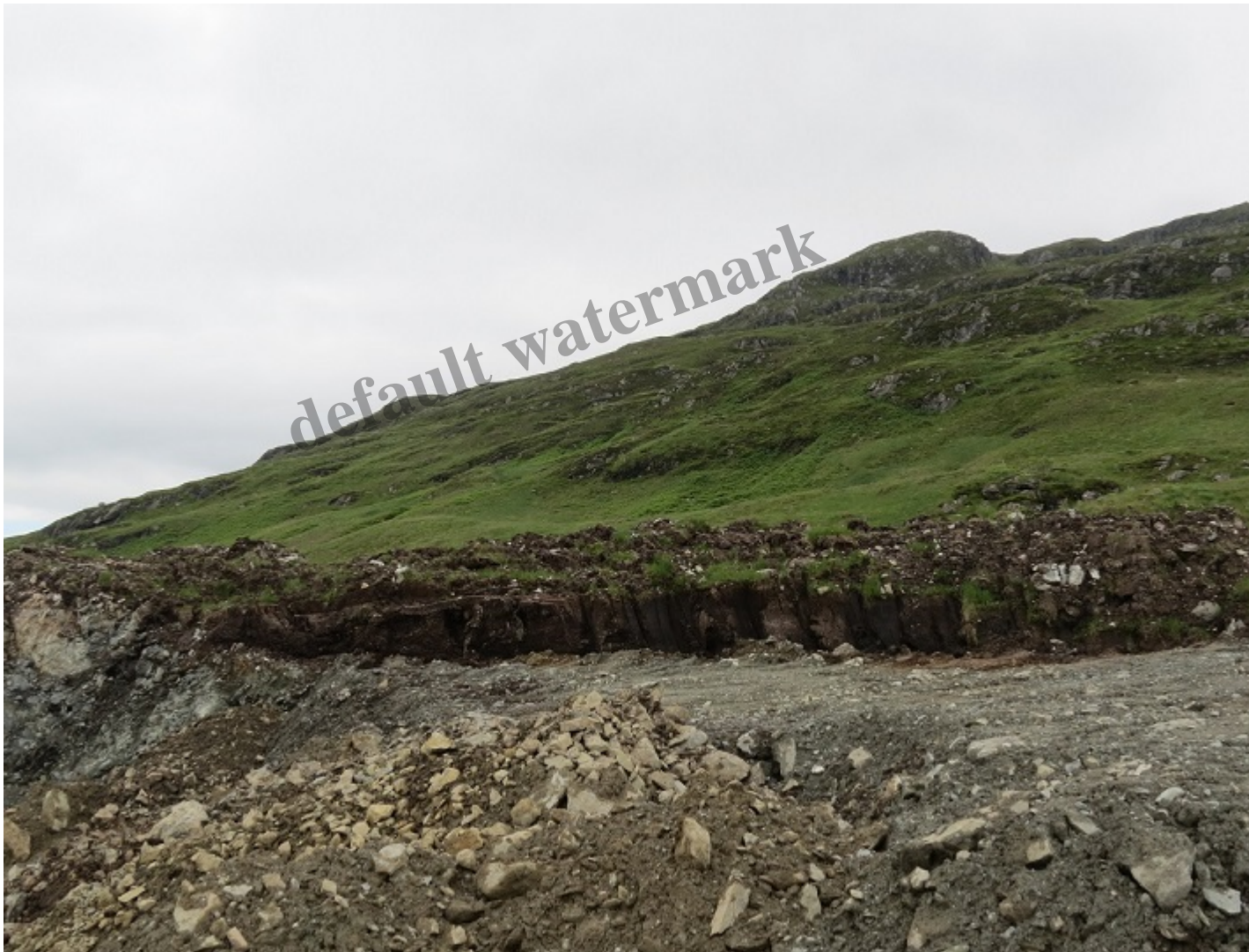
Partially restored borrow pit Ben Glas hydro 2016 showing levels of peat that were removed from the site – the edge of the peat was well over a metre high
