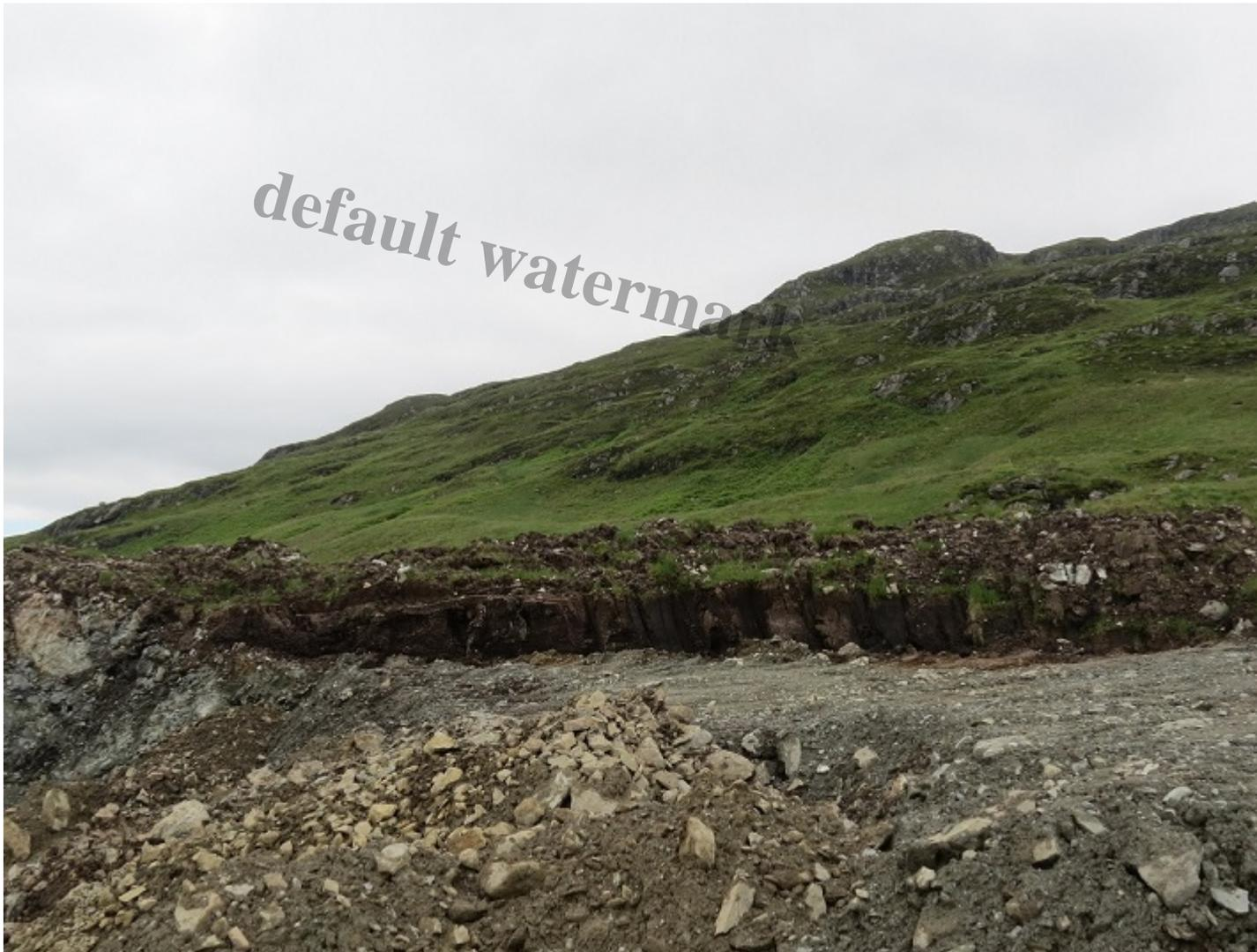
Partially restored borrow pit Ben Glas hydro 2016 showing levels of peat that were removed from the site – the edge of the peat was well over a metre high
