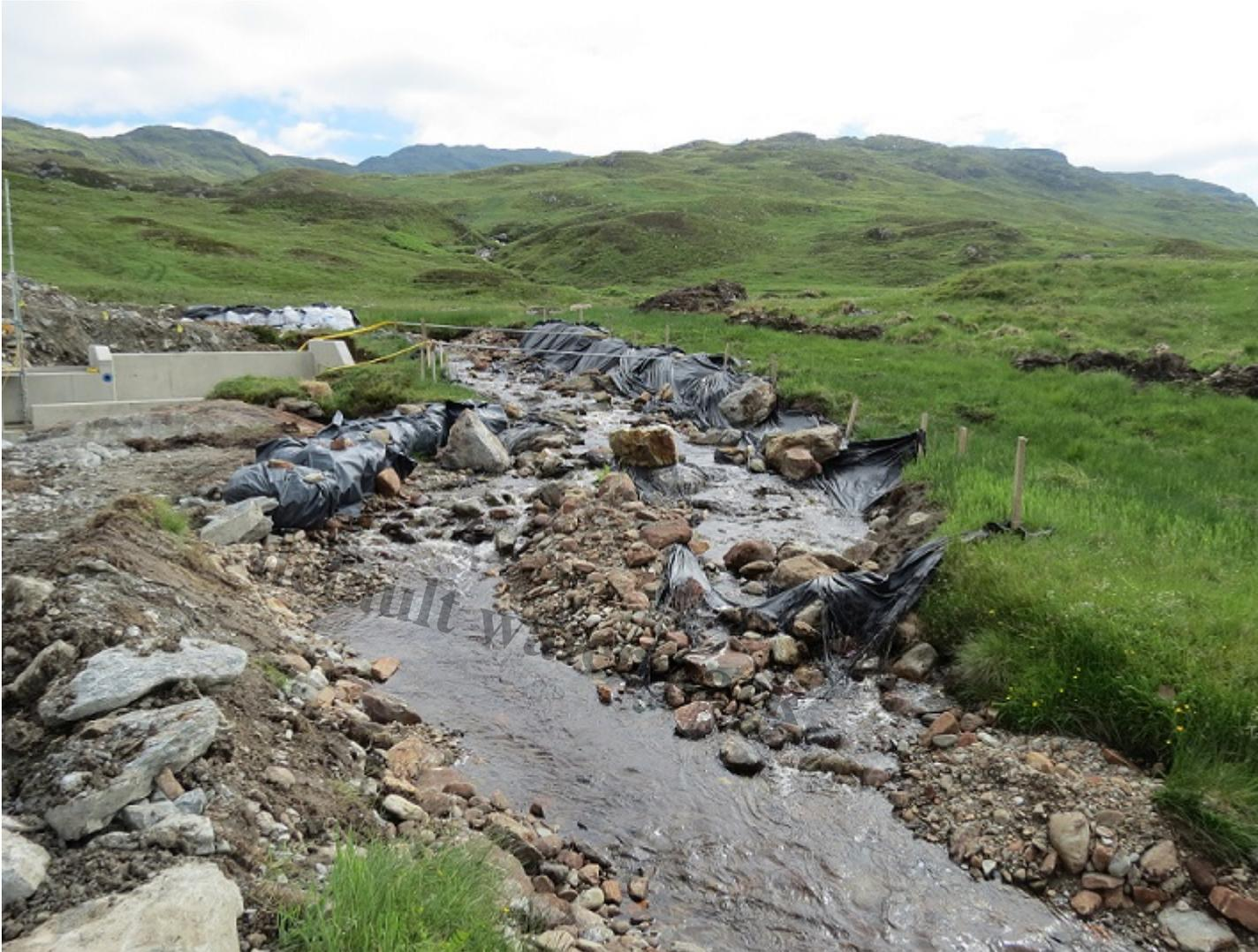
Diversion channel dug through peatland to construct hydro intake 2016. Note the piles of turf and peat to the right.
