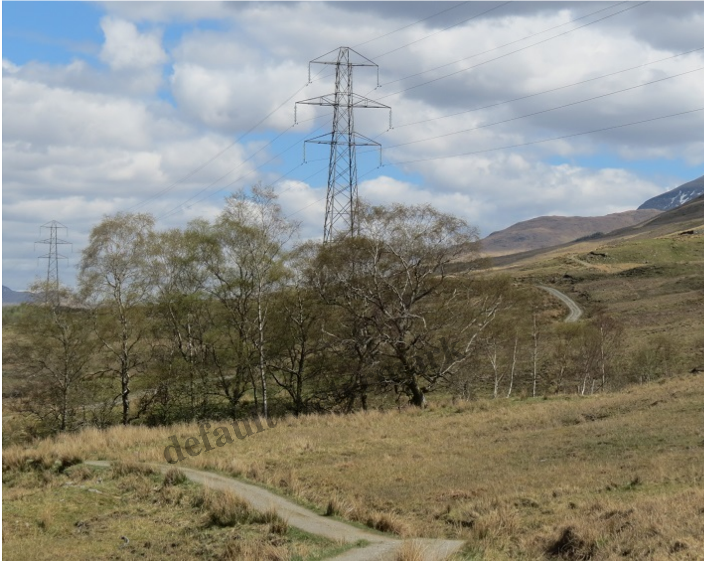
Powerlines above the West Highland Way in Glen Falloch
