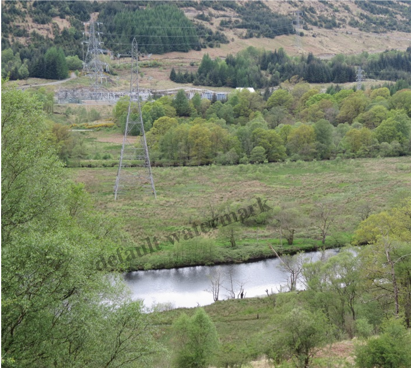
View from West Highland Way south of Ben Glas farm campsite over to the Falloch substation
