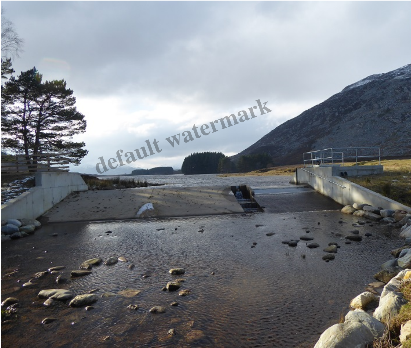
The hydro intake at the outflow of Loch Gynack which abstracts much of the water flowing out of the
