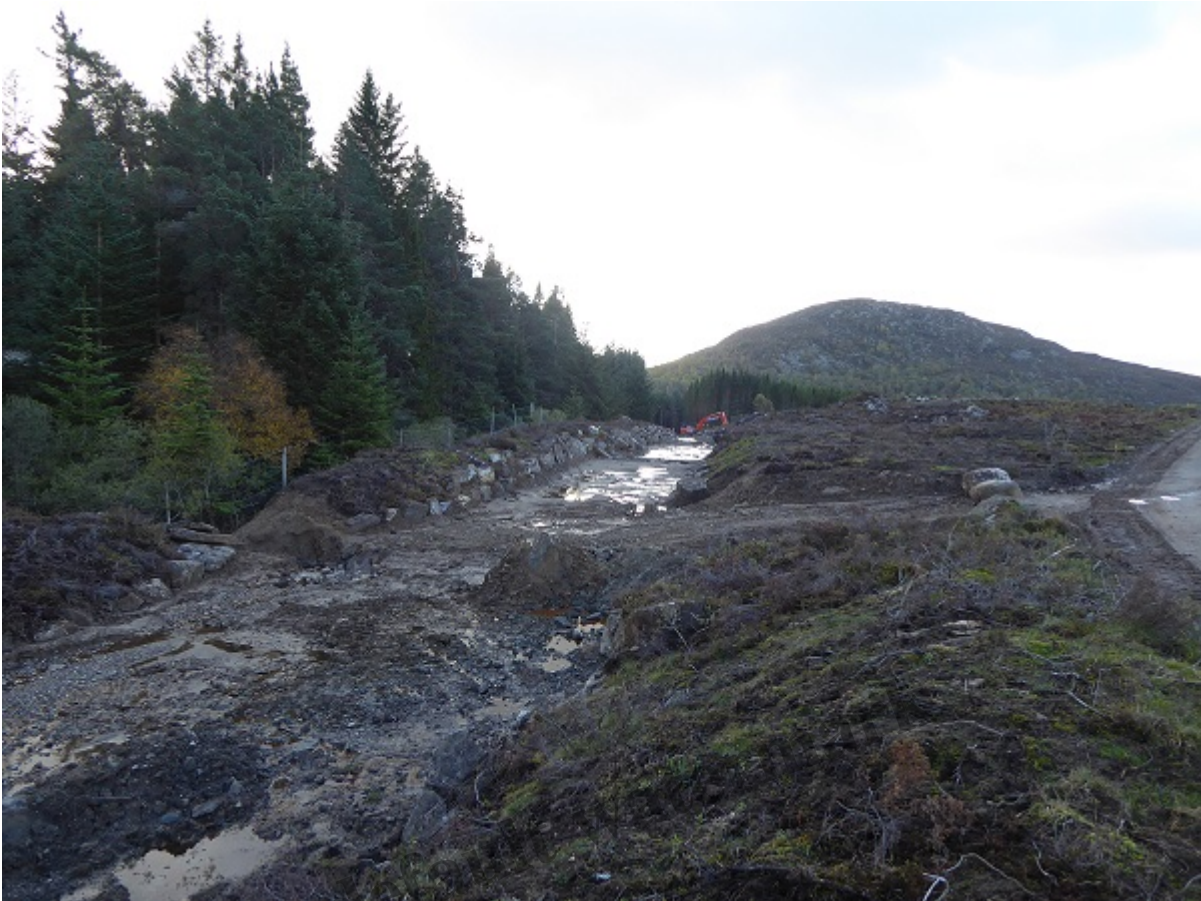
The overflow channel under construction October 2017 – note the new bank on the left
