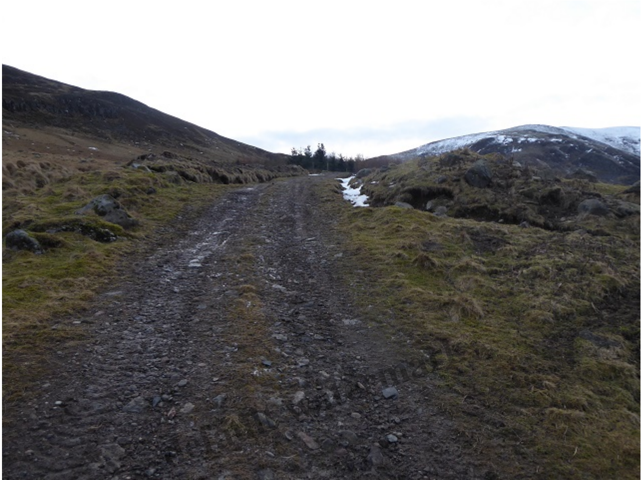
The first section of the road up to the wood is old and well constructed with a solid surface
