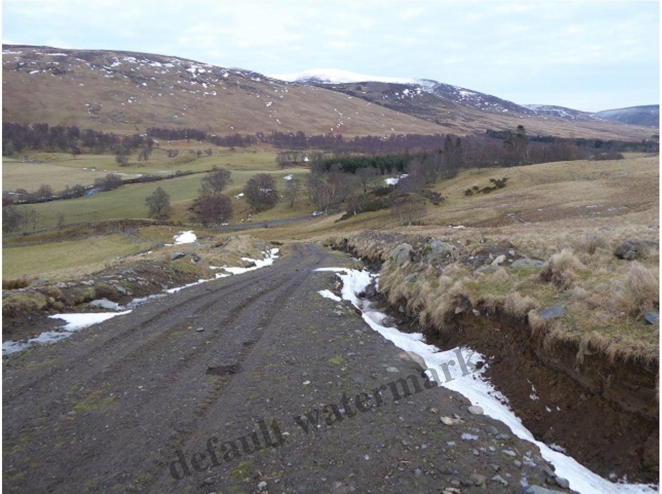
The improved section above is another matter – poorly constructed and far too wide
