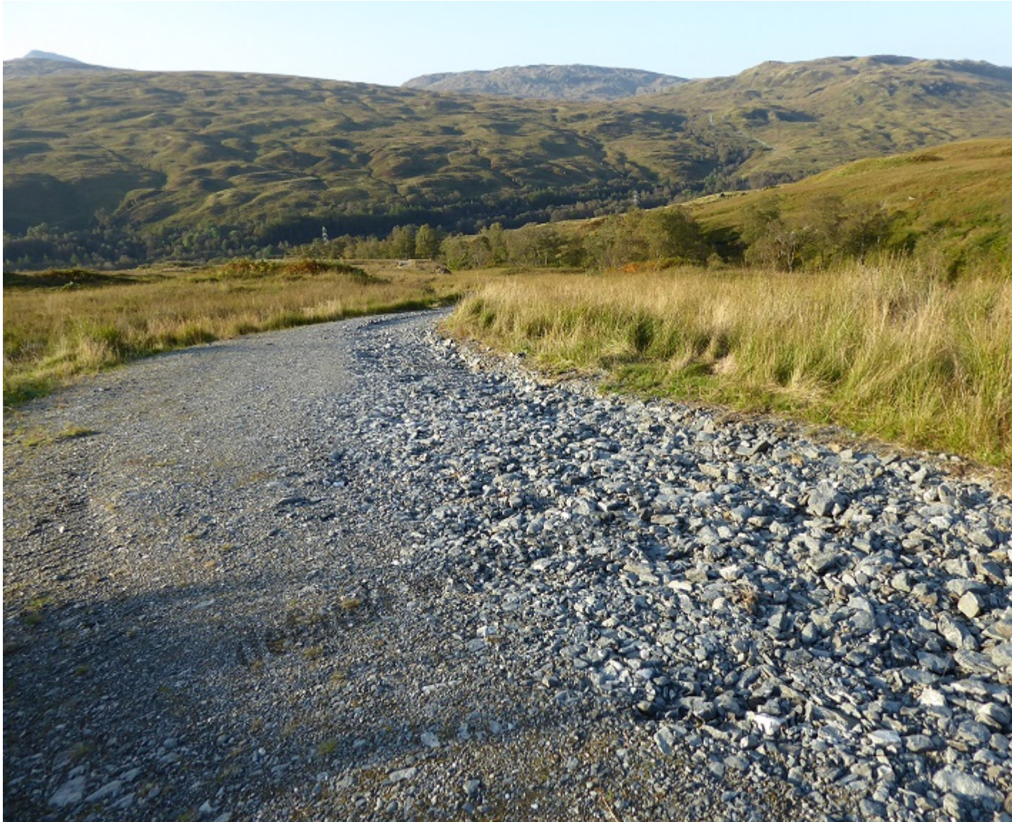
Section of Allt a Chuillinn road, which is more like a motorway than a track and contrary to LLTNPA specifications, with serious wash out on right side
