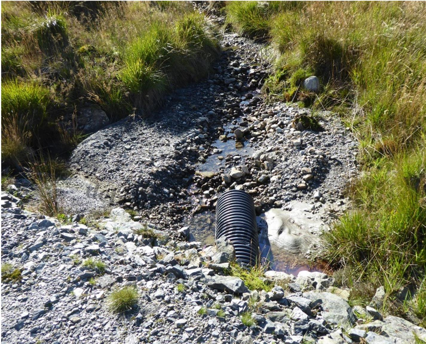
One of many protruding plastic pipes along the new road, silt visible to right, gravel wash out to left. also the eroding side of the track above the pipe.
