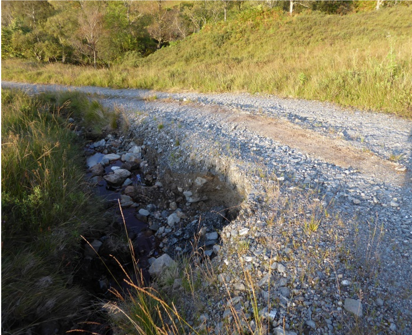
Edge of track eroded away by flood and now threatened with collapse
