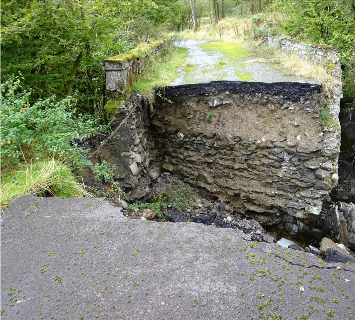
Bridge on the old road in Glen Falloch over the Eas Eonan swept away by the floods – could the Eonan intake have helped cause this?
