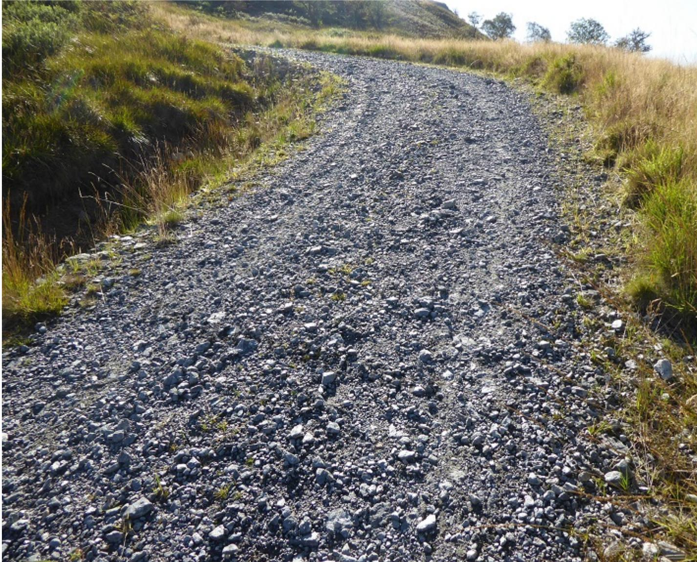
Fine material has been washed out from several sections of the new road and there is now a serious deep ruts developing which would make it unusable for vehicles.
