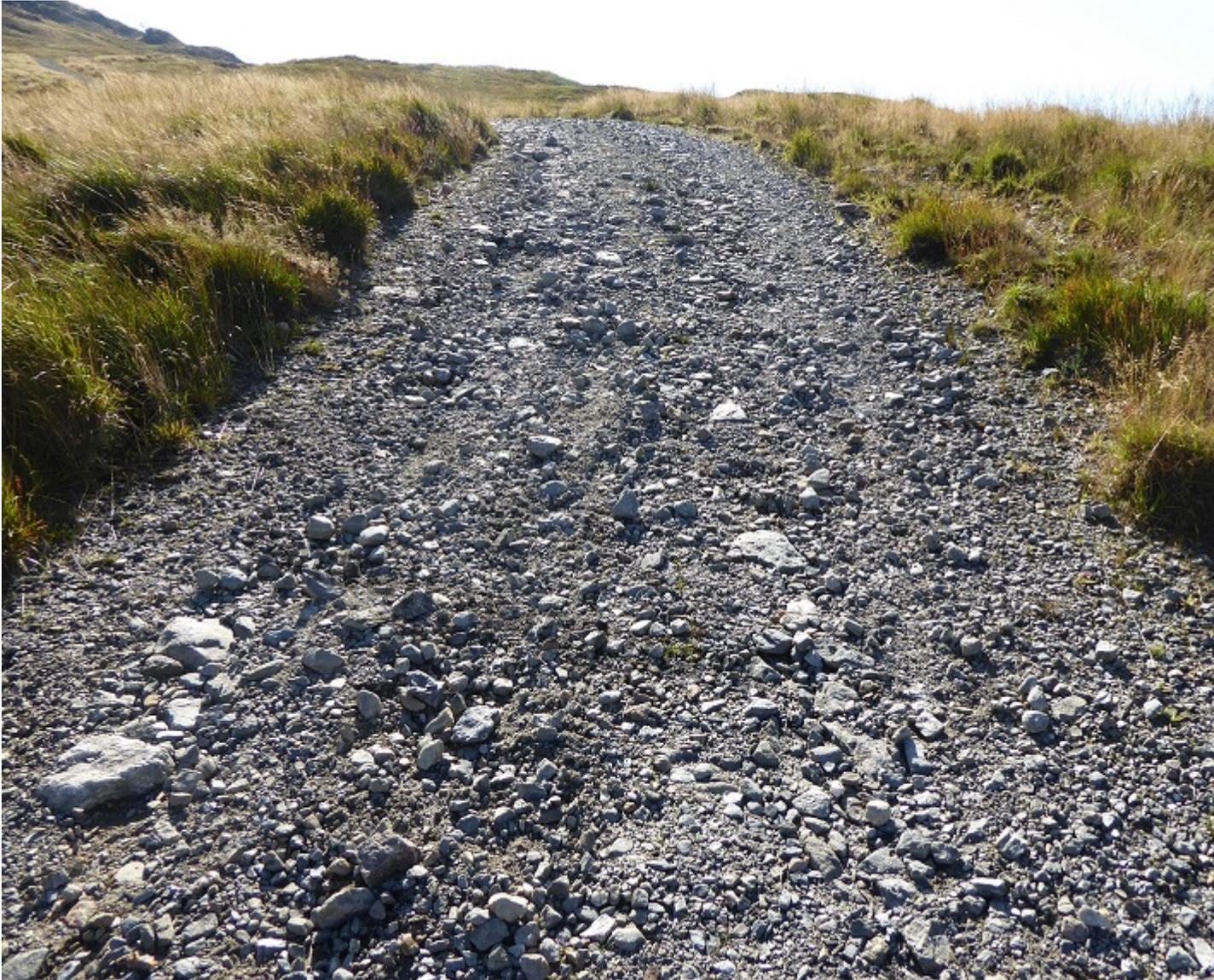
Example of section of road where the fine material has been washed out and where larger stones have started to be moved by the water.
