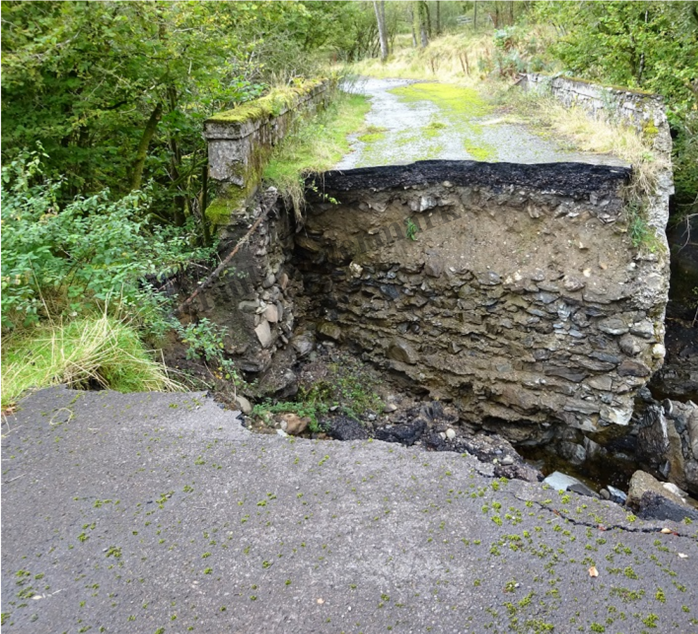
Bridge on the old road in Glen Falloch over the Eas Eonan swept away by the floods – could the hydro Eonan intake have helped cause this?
