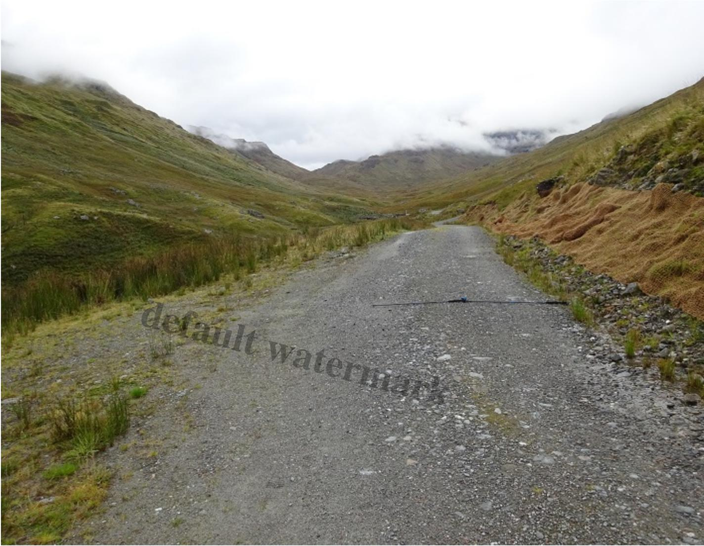
The road to the Glen Falloch Intake. Note how silt has been washed from the upper side to the lower side of the road widening it still further. The new textile matting that has been placed on the bank on right is the consequence of a fundamental failure in design – the bank is too steep. Photo Credit Kevin McGrath Sept 2019
