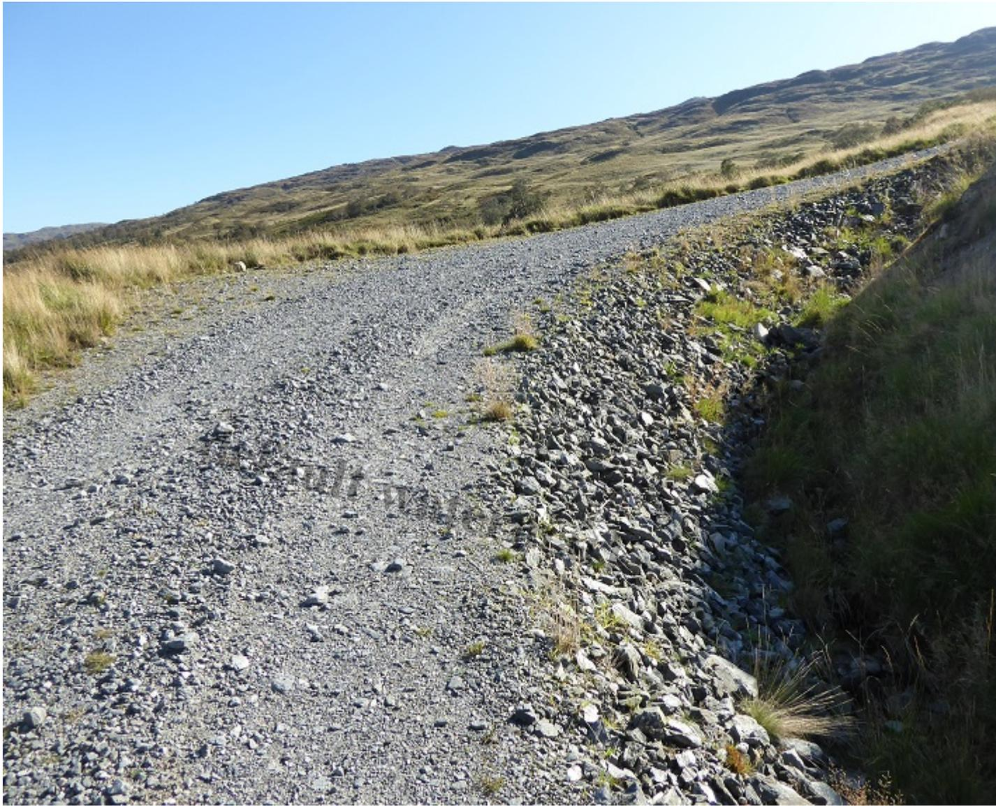
The right hand edge of the road is now starting to collapse into the enormous ditch
