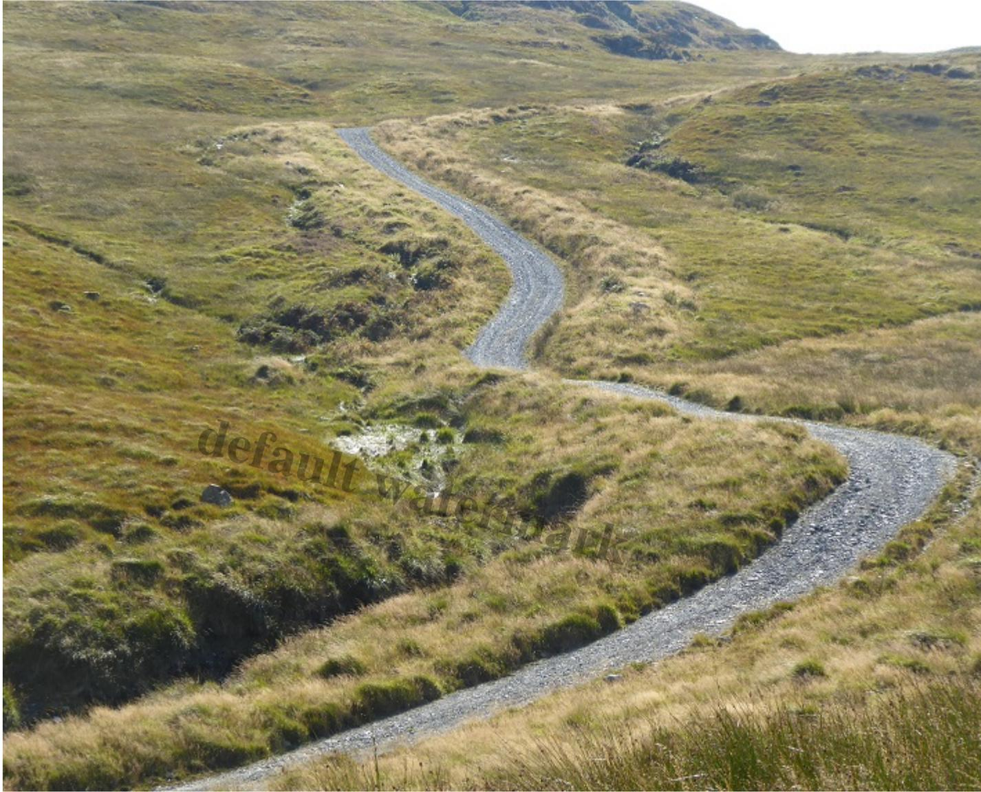
One of the middle sections of the road. The water is channelled down between the new banks that have been created here and is now seriously eroding the steep sections. As an illustration of how much water might have flowed here, note the flood flattened vegetation along the burn on the left.
