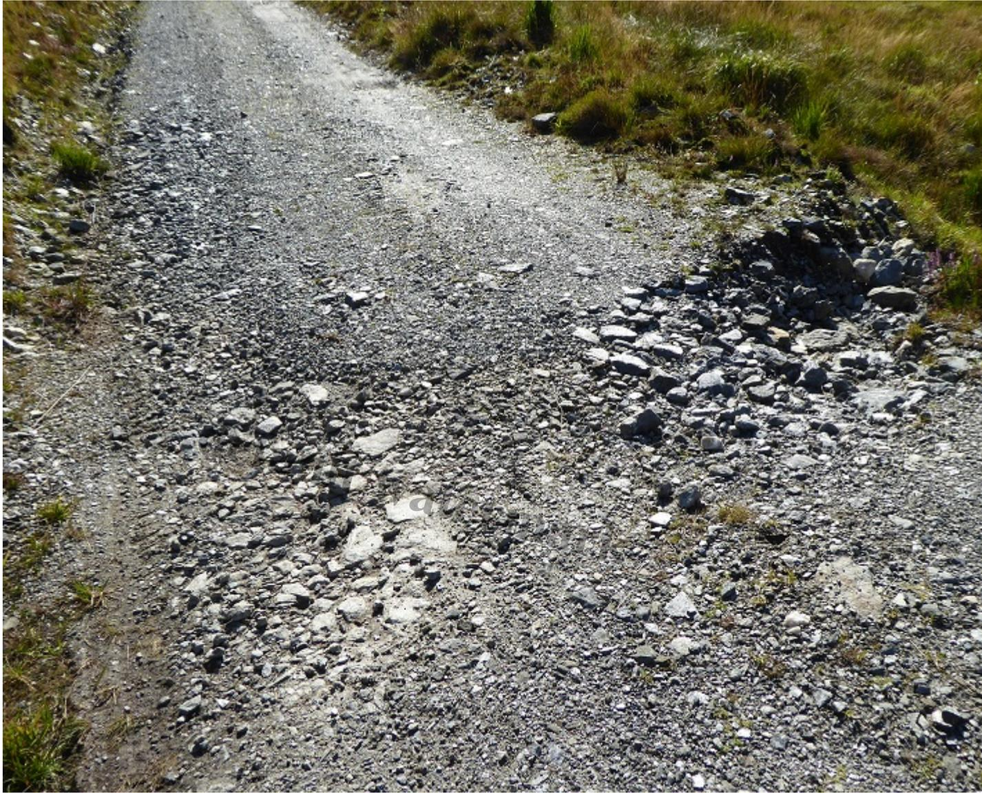
Collapsed section of road caused in part by water flowing across it and eroding its edge.
