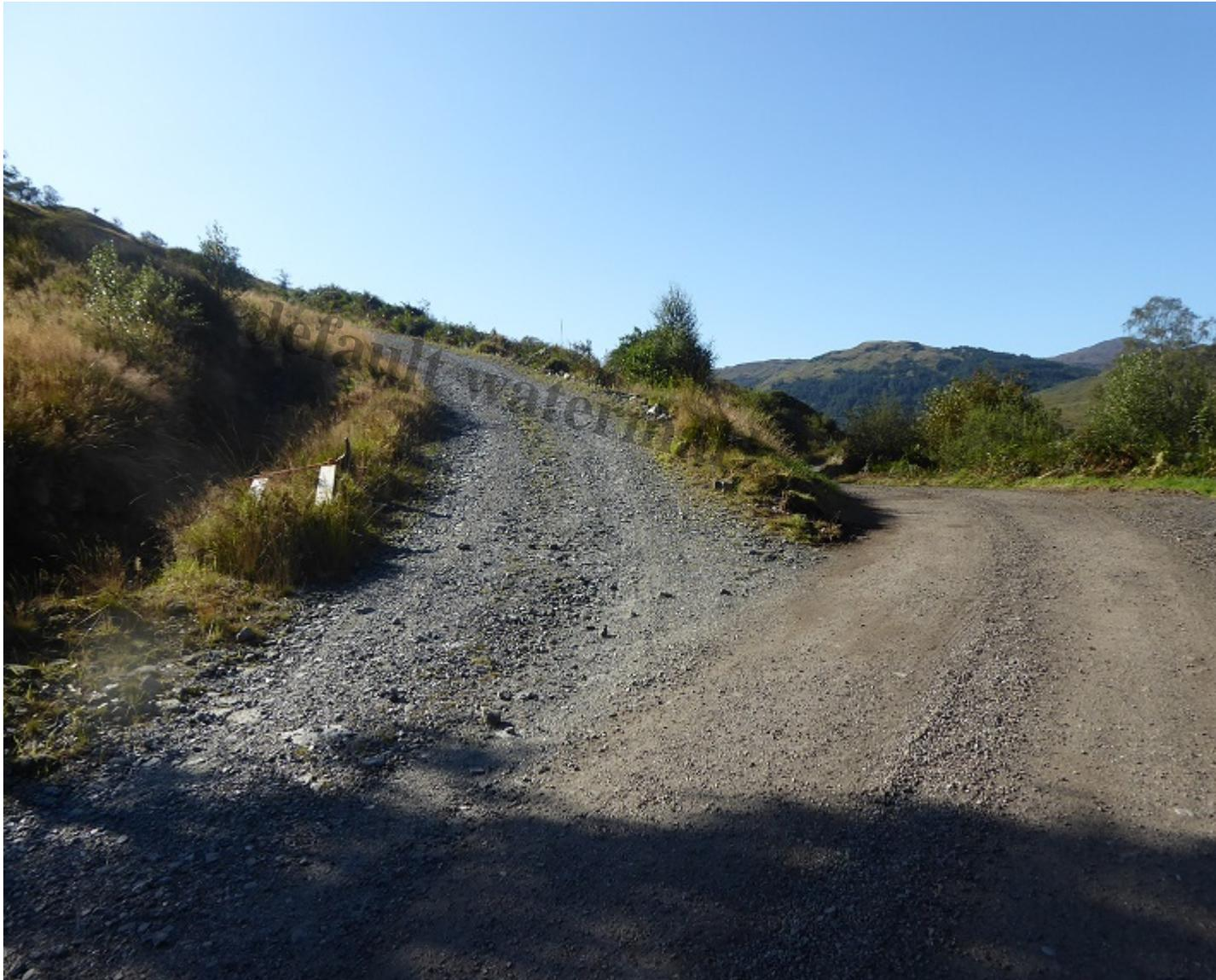
The start of the new Ben Glas hydro hill road illustrating the contrast between its surface, which is already eroding significantly, and the surface of the road below which has retained much finer material
