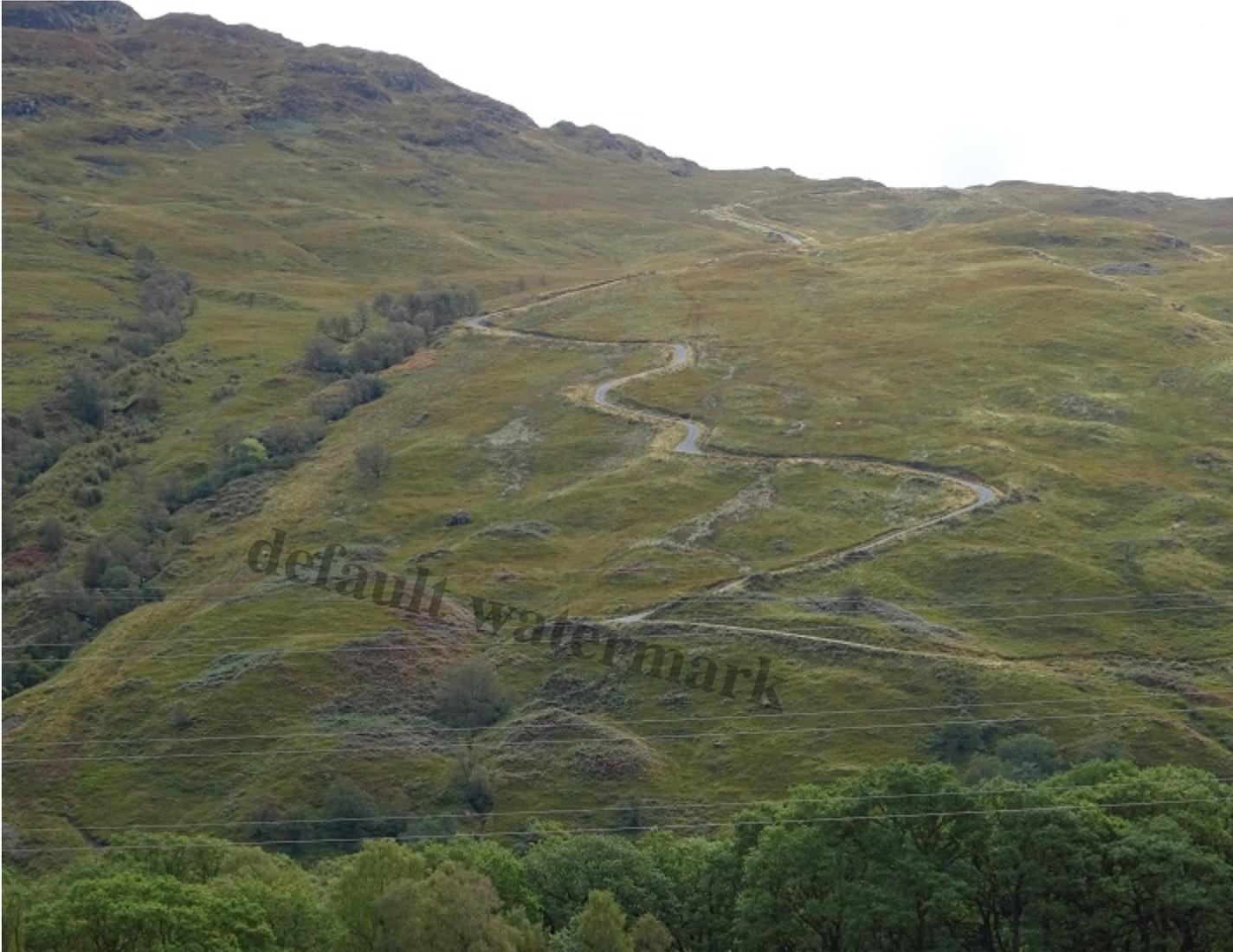
Ben Glas hydro road showing how material has been swept down from the road from the second bend onto the slopes below. Photo Credit Kevin McGrath Sept 2019
