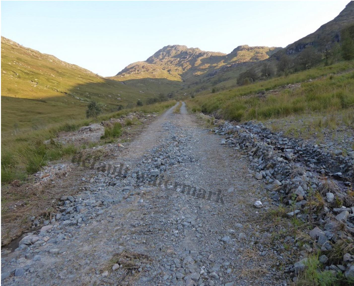
The view of the flood damaged area from below, showing how the central grass strip and part of surface swept away, with recent ditch work on right.
