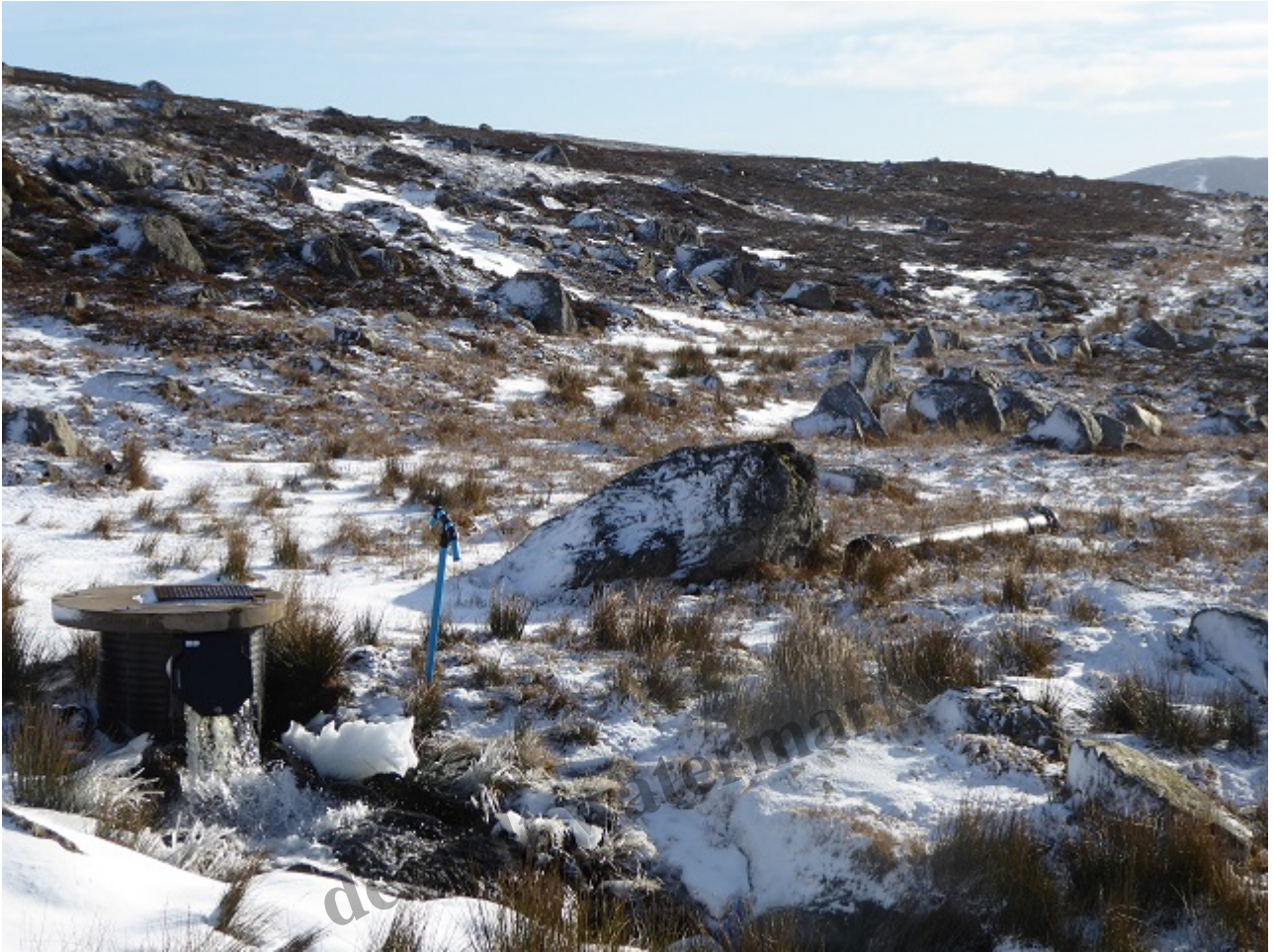
Abandoned pipe, centre right
