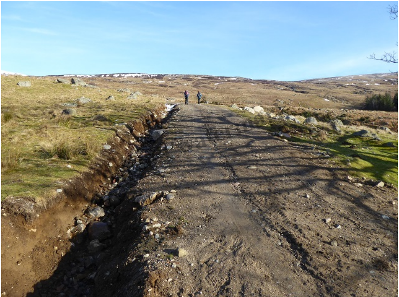
Near the bottom of the road, which runs north from the Clova hotel by the Corrie Burn, Feb 2019. Both the track surface and ditch are eroding. The footpath up to Loch Brandy lies out of sight to the right.
