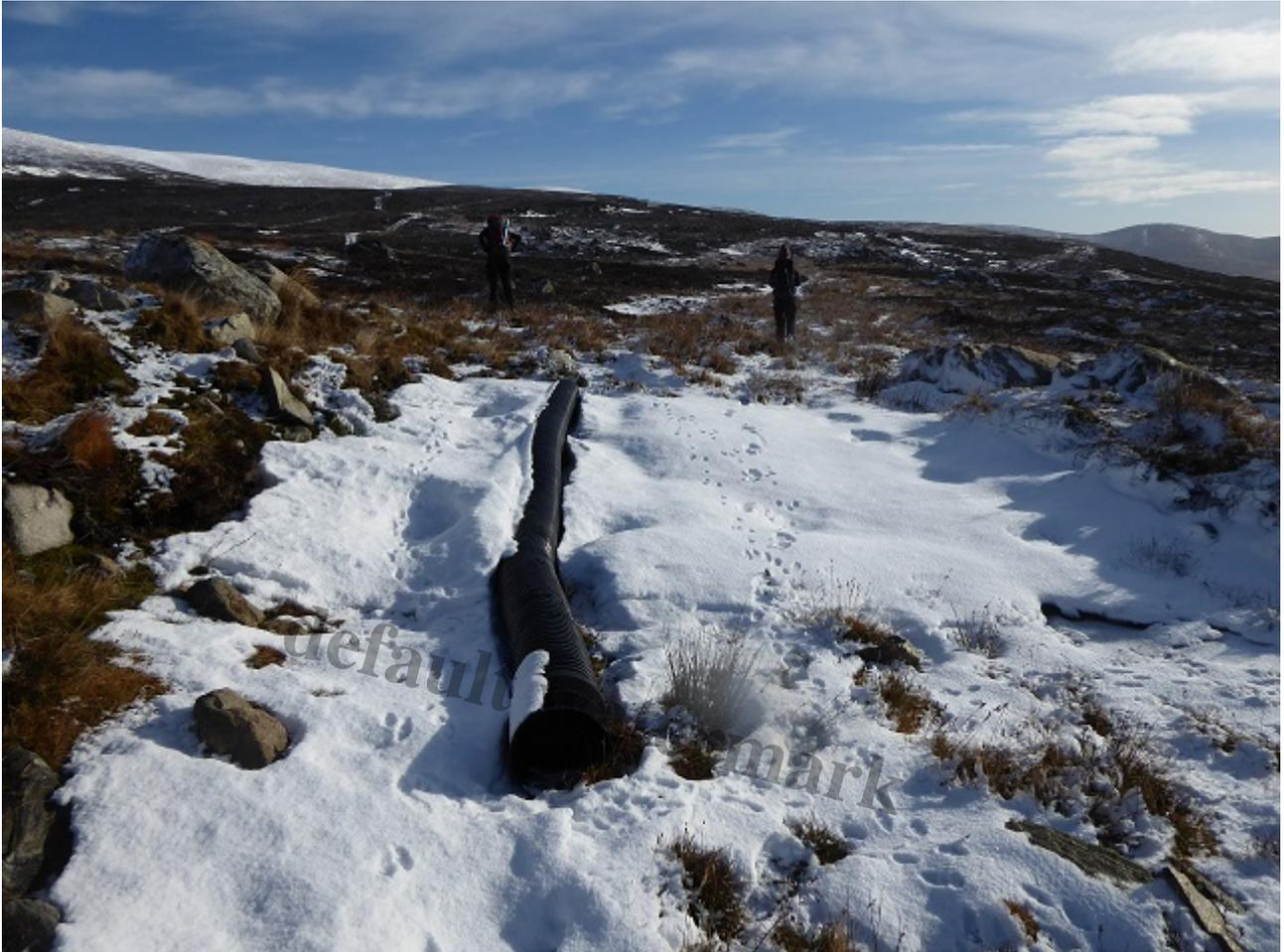
Drainage pipe laid down beyond • of constructed road by very boggy section of ATV track leading to hydro intake
