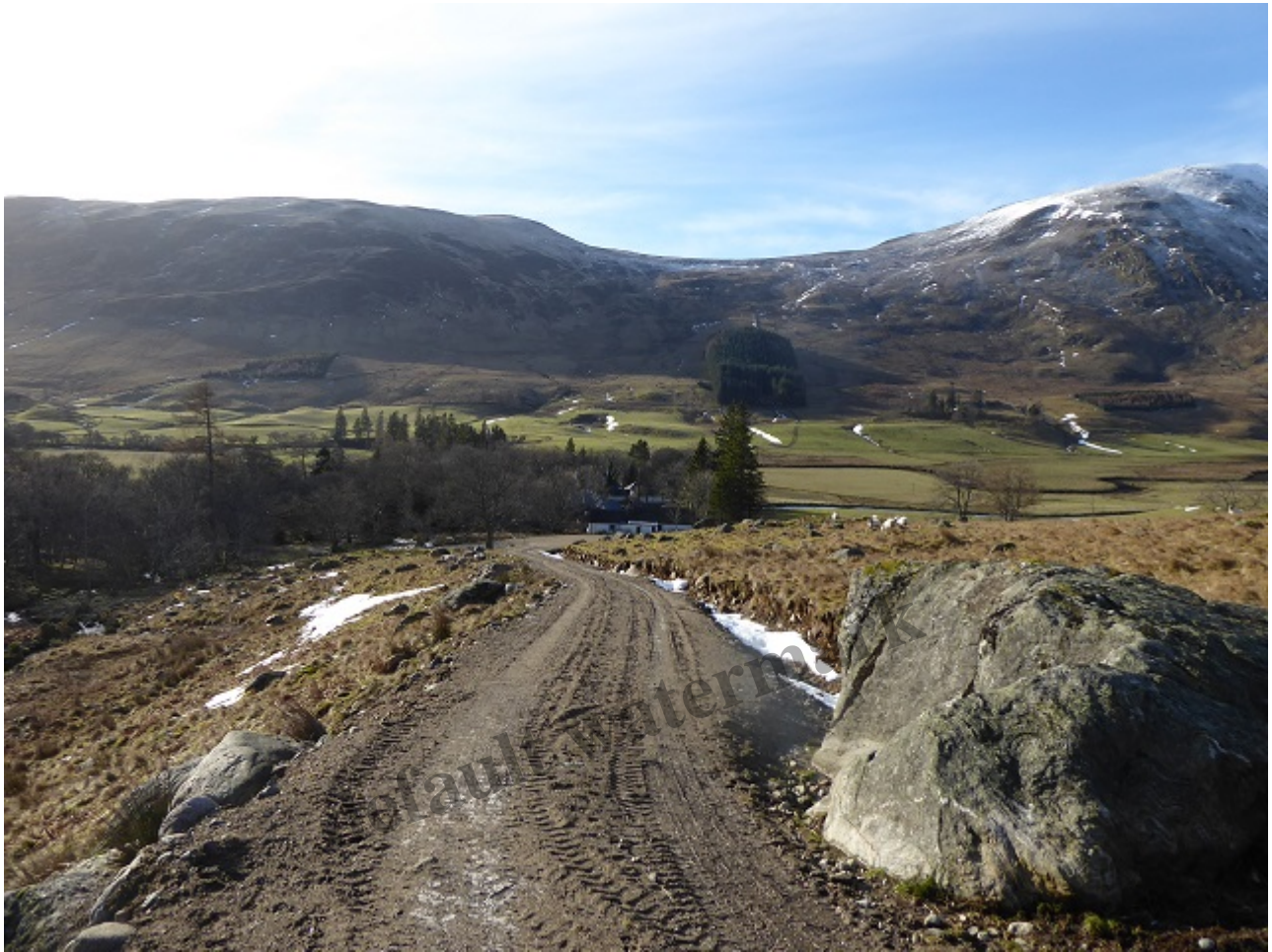
Looking down the first section of road. Feb 2019.
