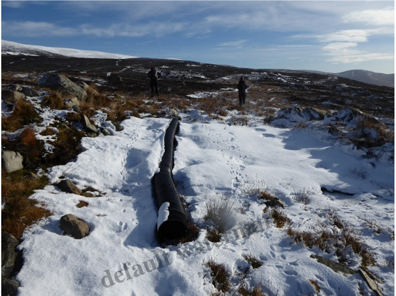
Drainage pipe laid down beyond “end” of constructed road by very boggy section of ATV track leading to hydro intake
