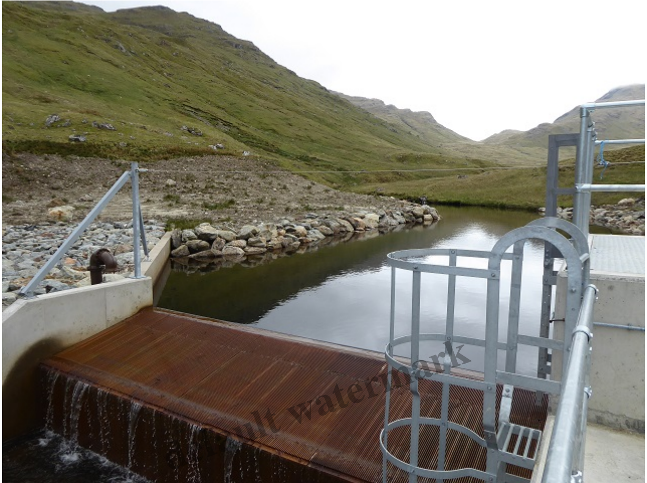
View over to same embankment May 2019
