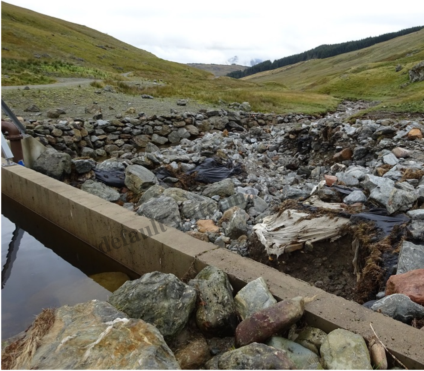
A closer view down from Upper Glen Falloch showing how boulders have been swept off the plastic
