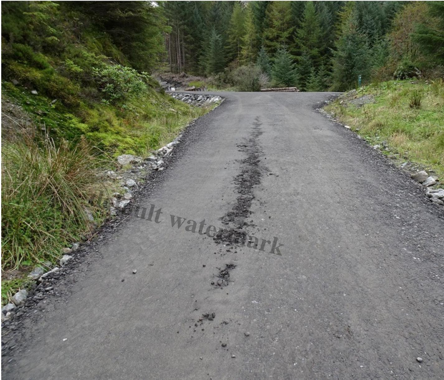
Disintegrating surface finish – one of many examples seen along the way
