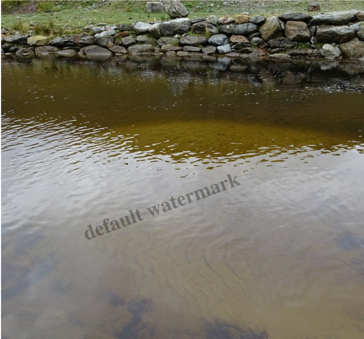
Bottom of intake pool September 2019 – the dam wall is just to the right. Photo Credit Kevin McGrath
