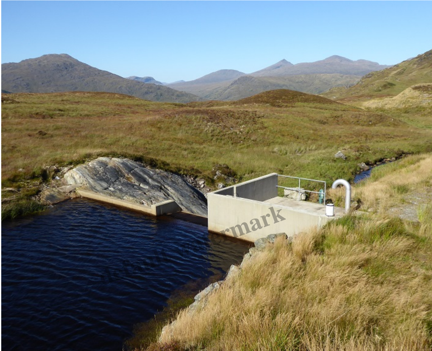
Southern Ben Glas hydro intake, Ben Lui massif in background
