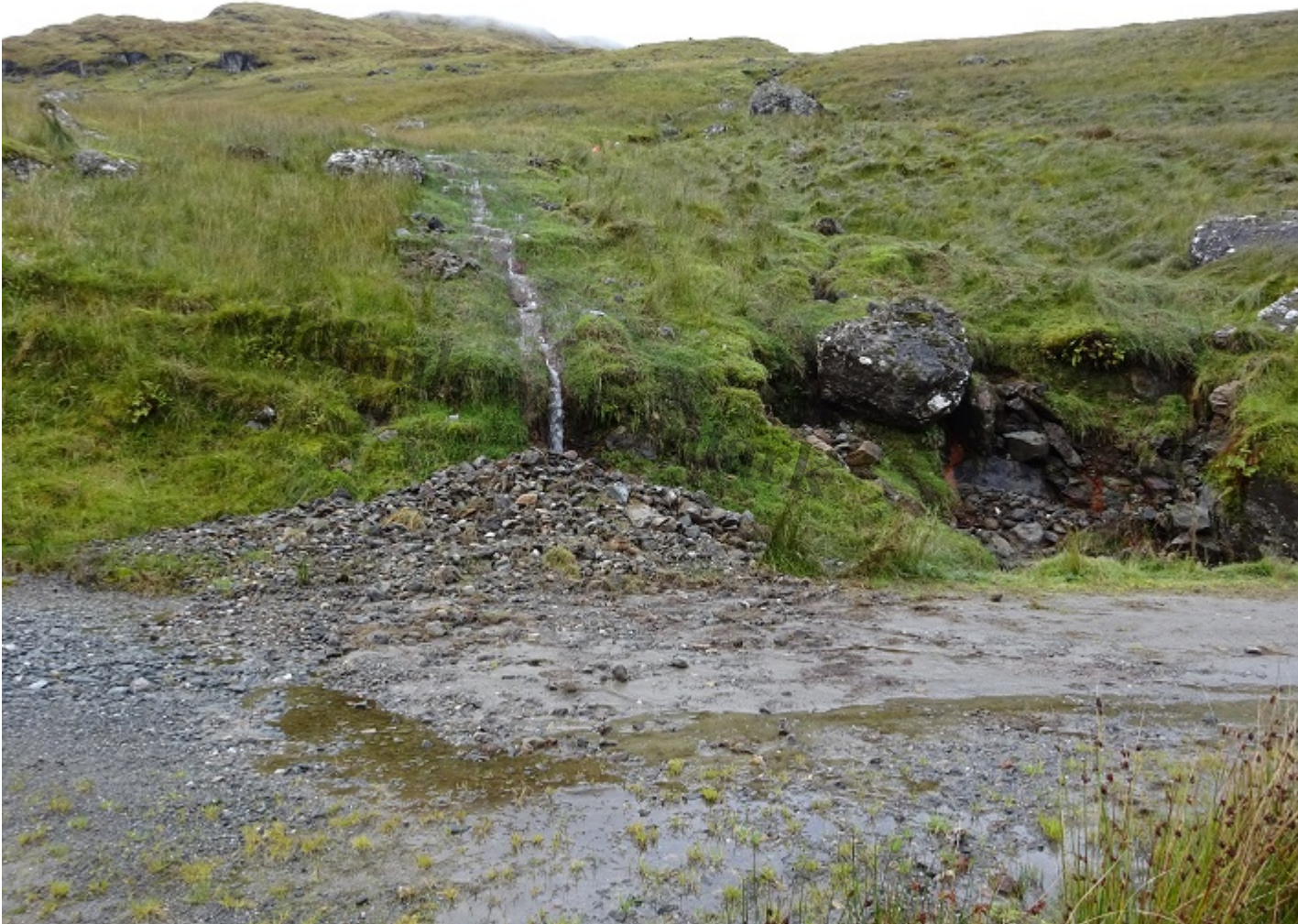
Burn by track up to Upper Glen Falloch hydro intake. Until recently it flowed down by the boulder on right. Note the amount of debris washed down by the burn onto the track. Photo credit Kevin McGra 25th September.
