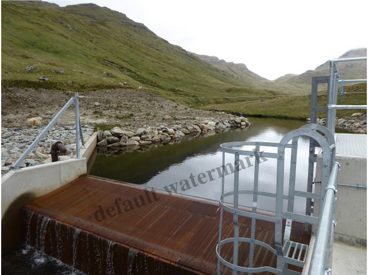
Upper Glen Falloch intake pool May 2019
