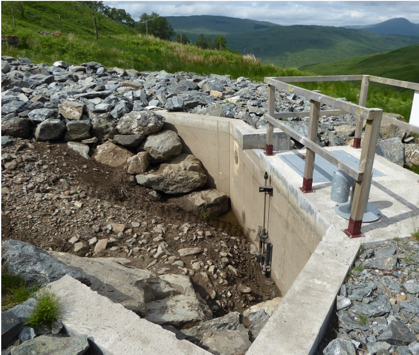
Photo of same dried up intake June 2018. Intake just to left of far post.
