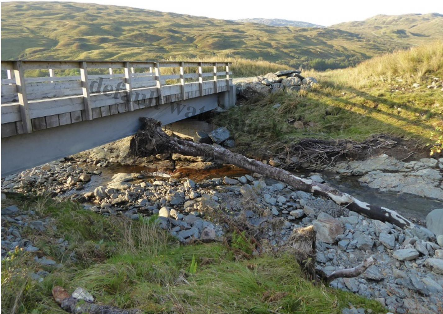
One scene from lower down the Allt a Chuillinn at the new bridge constructed for the hydro scheme. how vegetation has also been removed from the bank on the right
