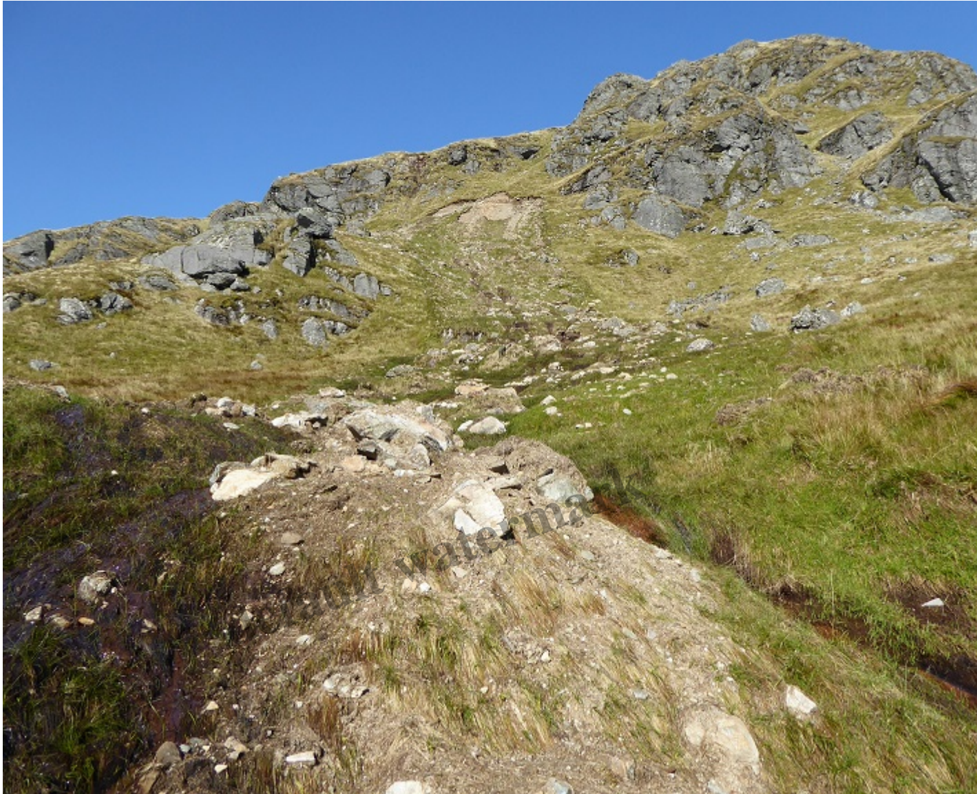
Looking up the same landslip from below
