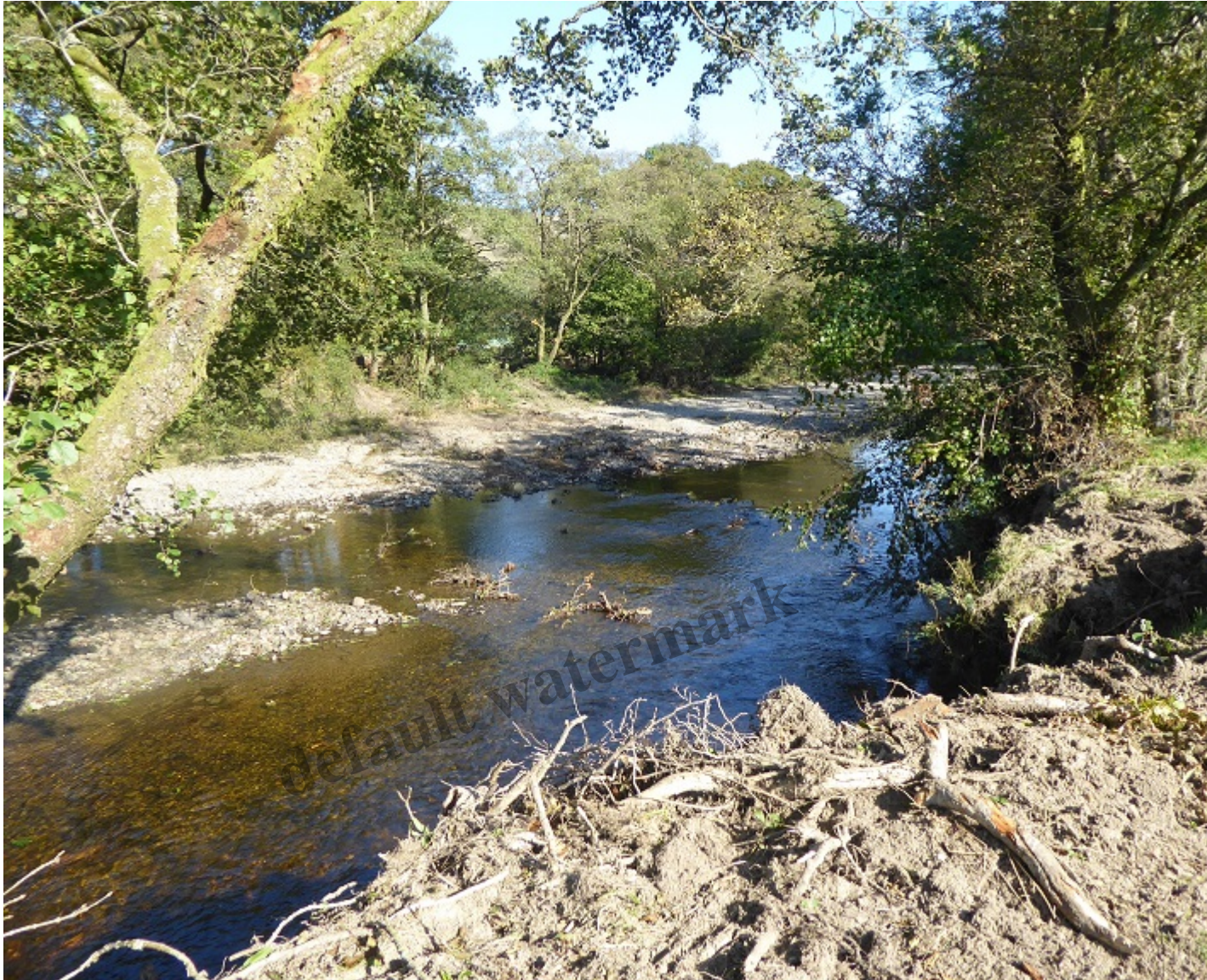
Several sections of bank have been completely stripped of trees and vegetation
