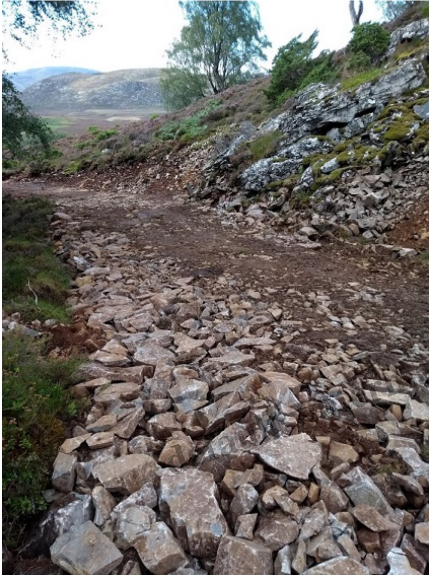
Base of new road being laid with signs of preliminary restoration of cutting on right side of track (stones piled on bank just above centre right of photo)
