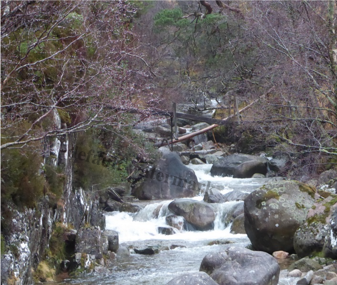
The confined gorge and pedestrian bridge just above the proposed location of the intake
