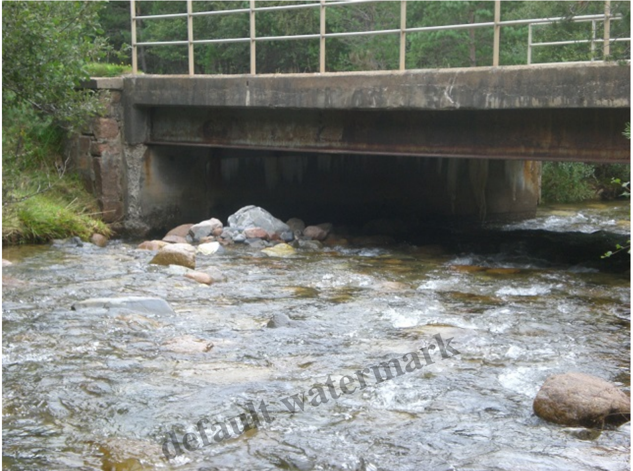
Allt Mhor bridge viewed from above. The flooding has created a new bank of boulders on the opposite side of the bridge to that which was infilled last year. Photo credit Alan Bratney.
