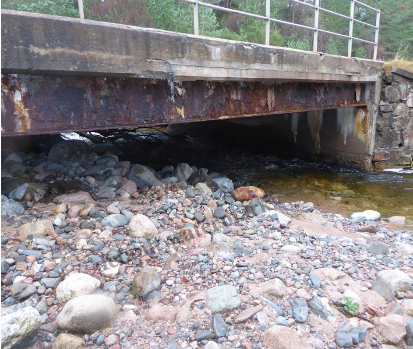
Allt Mhor bridge November – viewed from below – note how the left side of the bridge was half blocked by boulders
