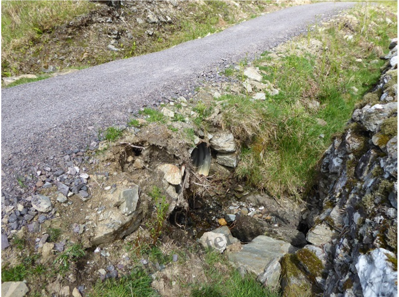
Another collapsing culvert which unless addressed is likely to erode back into the path surface in the near future
