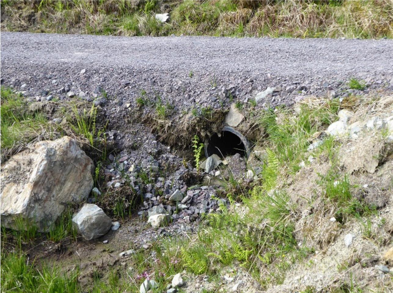
Surfacing from the path is already eroding away and the standard of finishing around the culverts is as poor as any old bulldozed track. Is this the way to treat the old military road and what is our best known long distance walking route?
