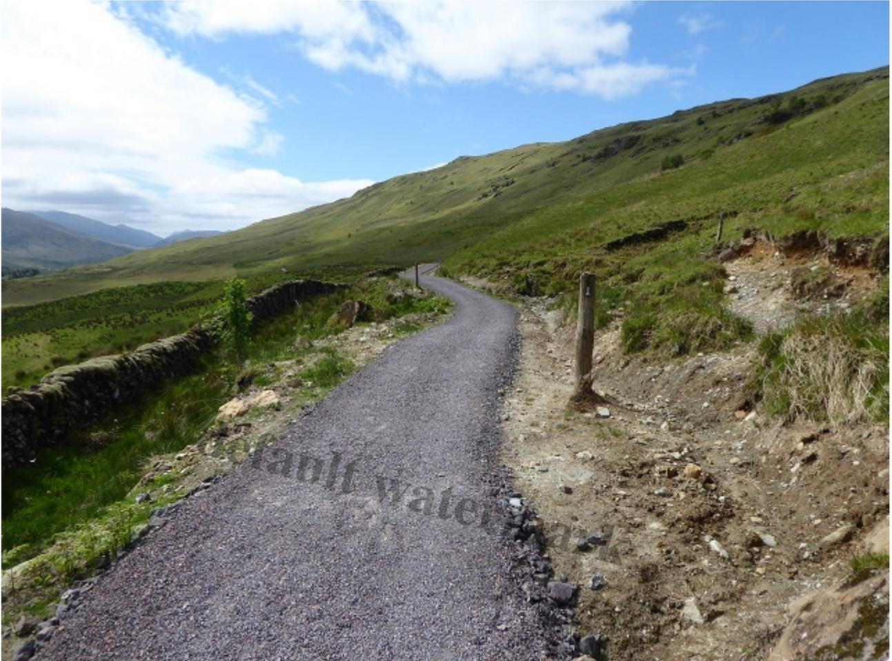
The ground in this photo could have immediately been restored with turves if they had been kept instead of dumped on the lower side of the path. Instead its likely to take several years to revegetate.
