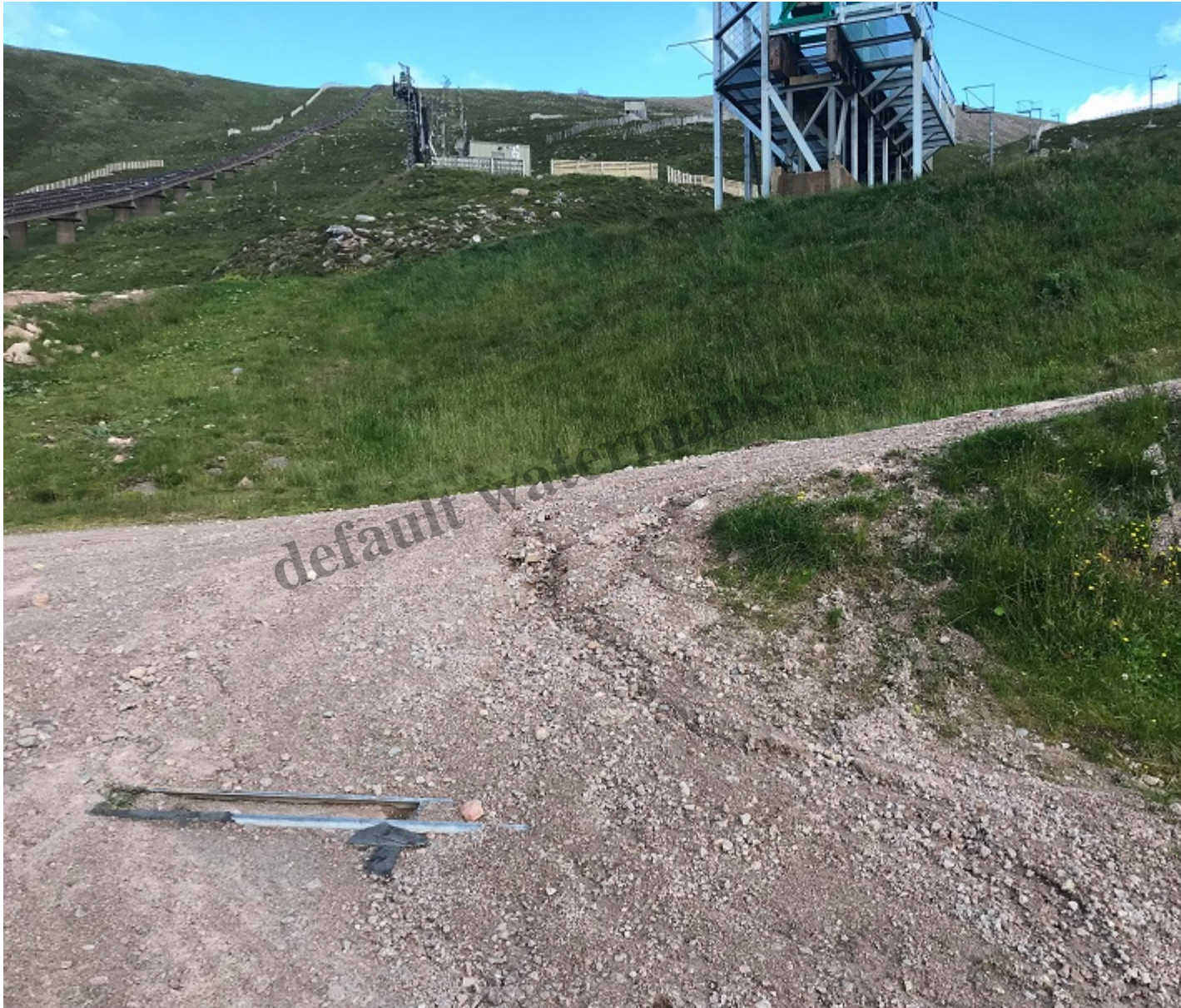
Granitic Material is being washed down the steepest section of track, has almost completely filled in bars and has covered much of the vegetation alongside the track. Photo courtesy of Alan Bratney.
