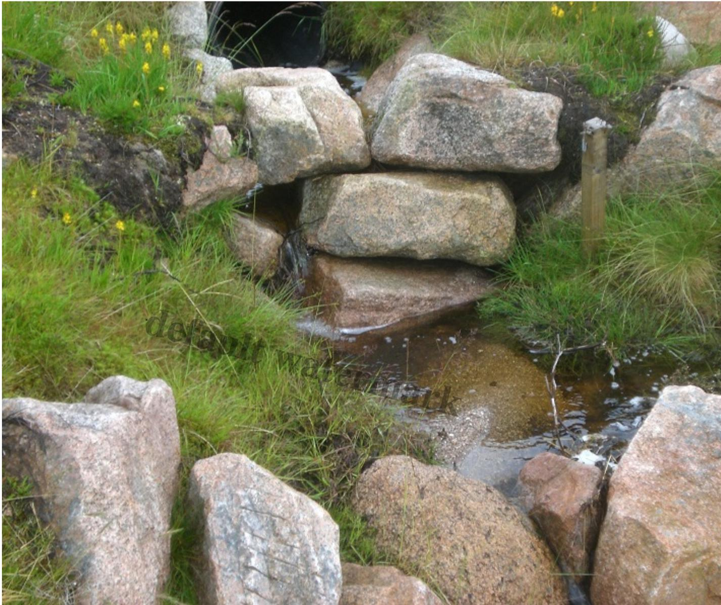
Infilled silt trap below the shieling track designed to reduce the amount of grit washed down the mountain. The trap would never have been needed if the planners do not anticipate the track would continue to erode. The traps were supposed to be regularly emptied. Photo Credit Alan Bratney.
