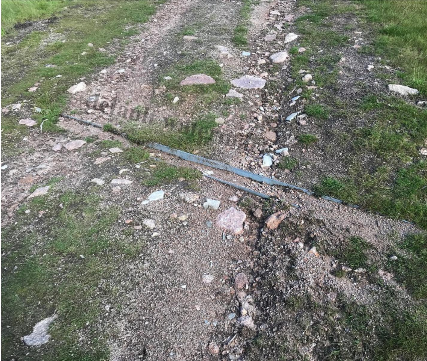
The reseeded along the edge of track and of the central strip has not prevented large amounts of gravel from being eroded and washed down the track. Photo courtesy of Alan Bratney.
