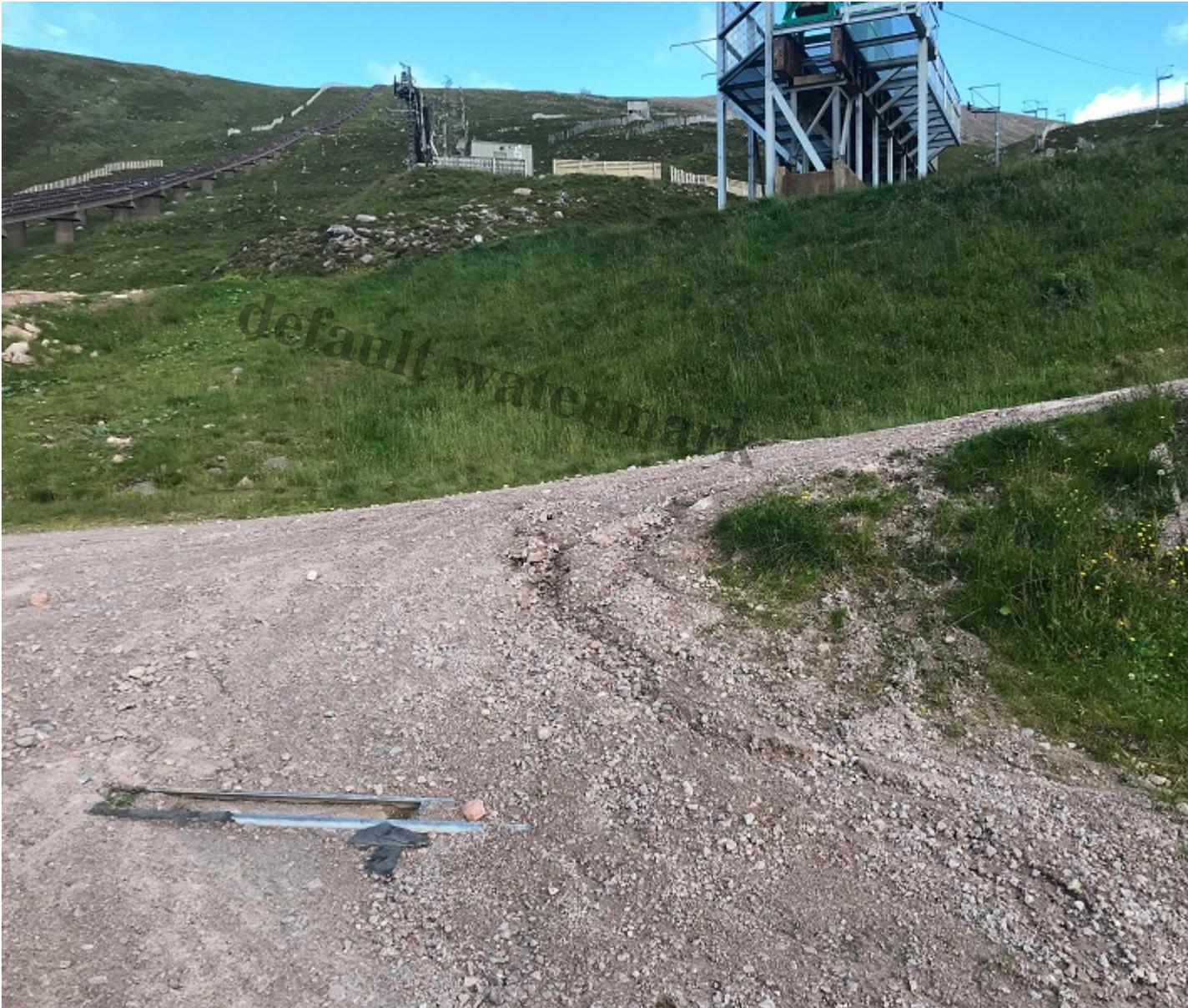
Erosion of Shieling Track at Cairngorm taken BEFORE the recent heavy rainfall. Note how material washed away by the water has spilled onto the vegetation, widening the track, the erosion channel at the corner and the water bar has filled in. This and other tracks appear at high risk of washing away completely in future heavy rain. Photo courtesy of Alan Bratney.
