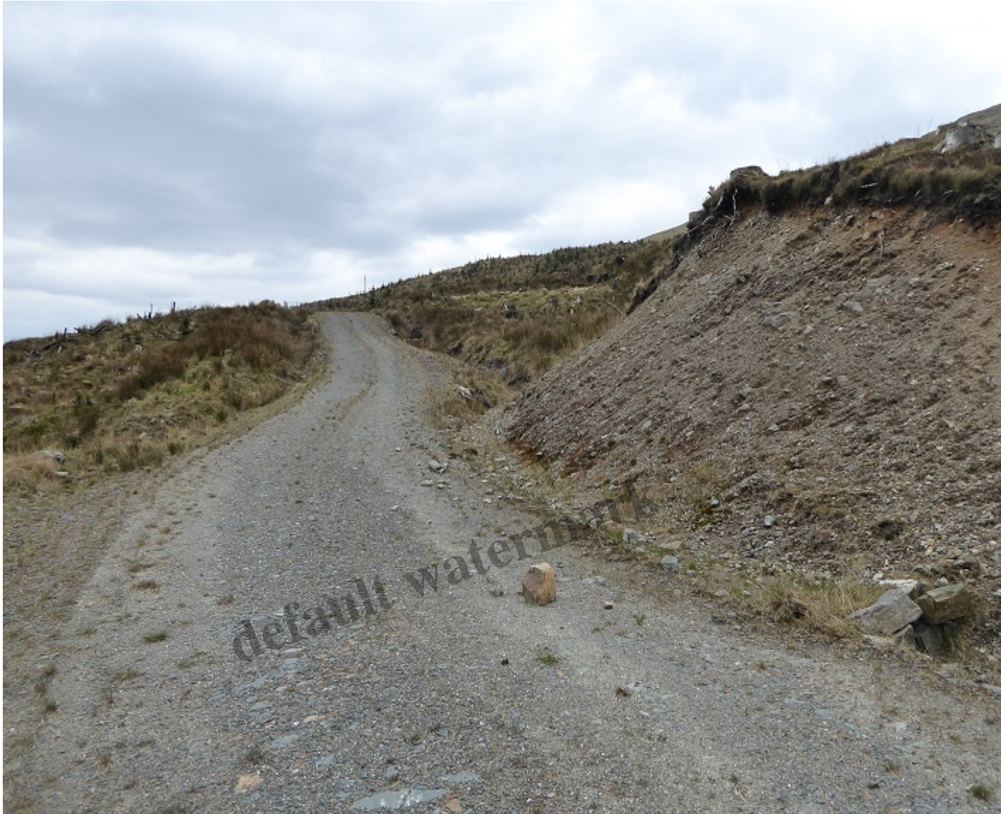
The top spur to the intake – there has been no attempt to restore the bank which is now eroding
