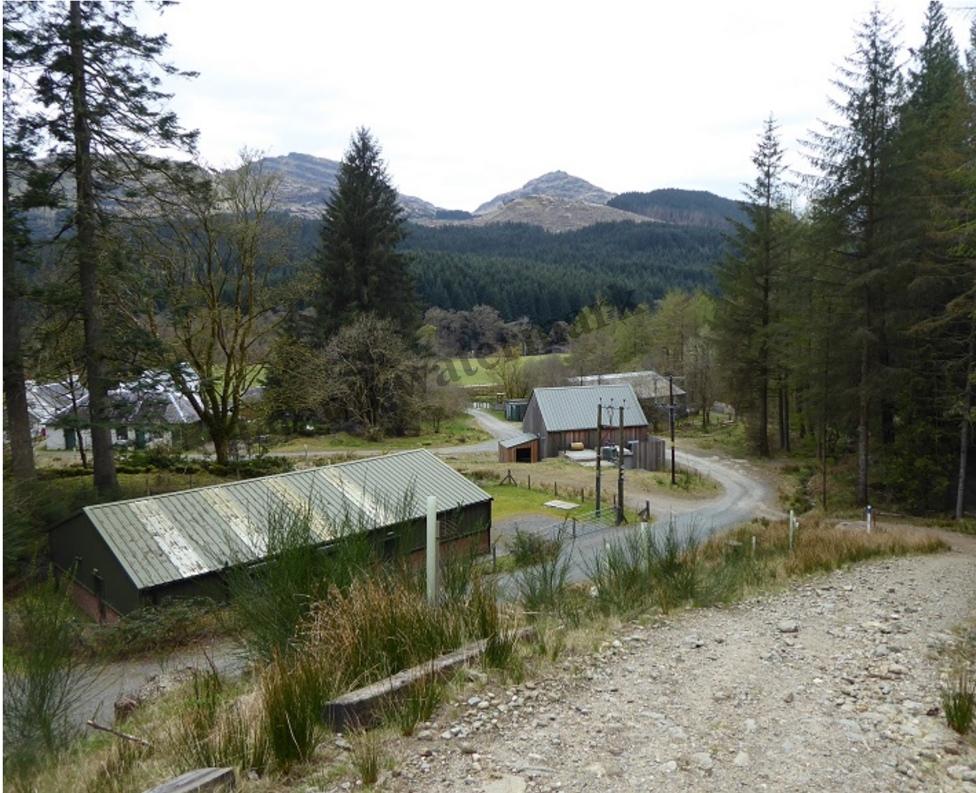
Powerhouse just right of centre, Beinn Bheula behind on left
