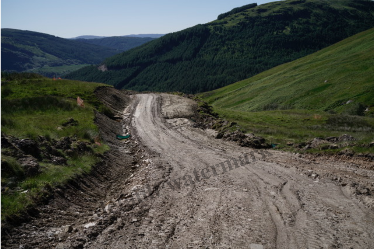
More turves dumped upside down – the best way possible to kill of the vegetation. Photo Credit Tom Prentice.
