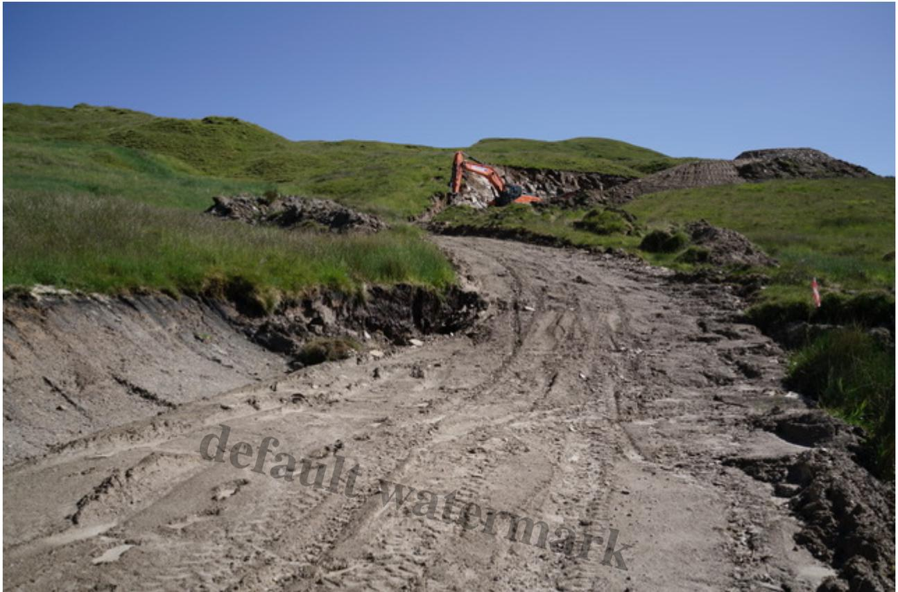
Construction in progress. Note the bare sides to the ditch on the left and the piles of peat and turves on either side of the road. Photo Credit Tom Prentice.
