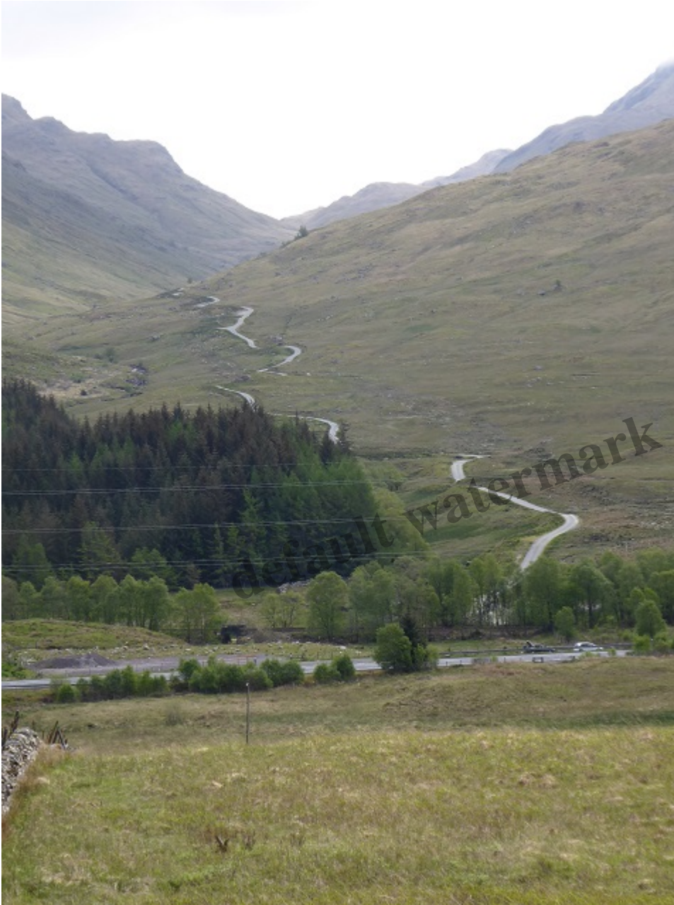
The first two sections of the upper Glen Falloch hydro road viewed from just below the West Highland Way
