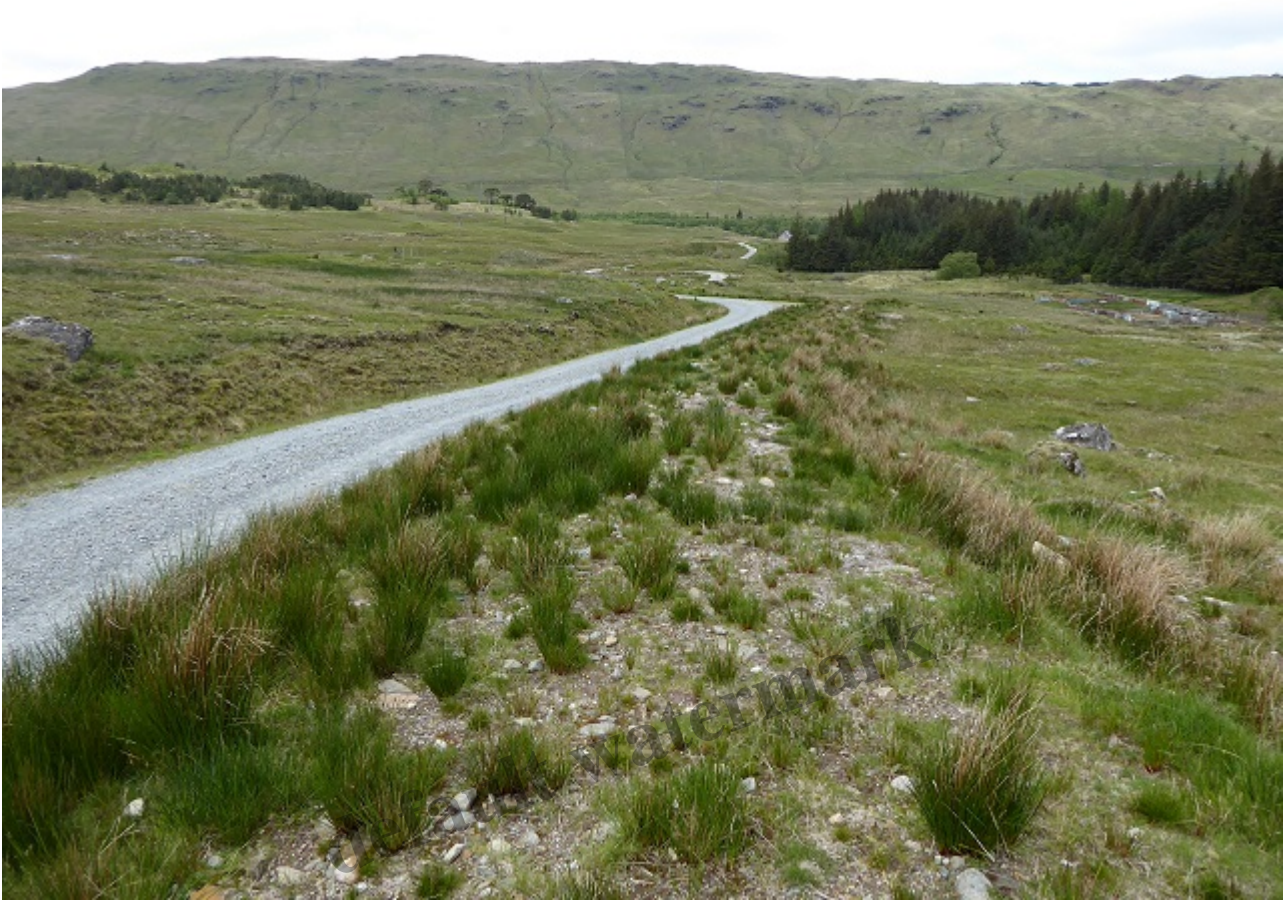
Looking back north along the road to the powerhouse.
