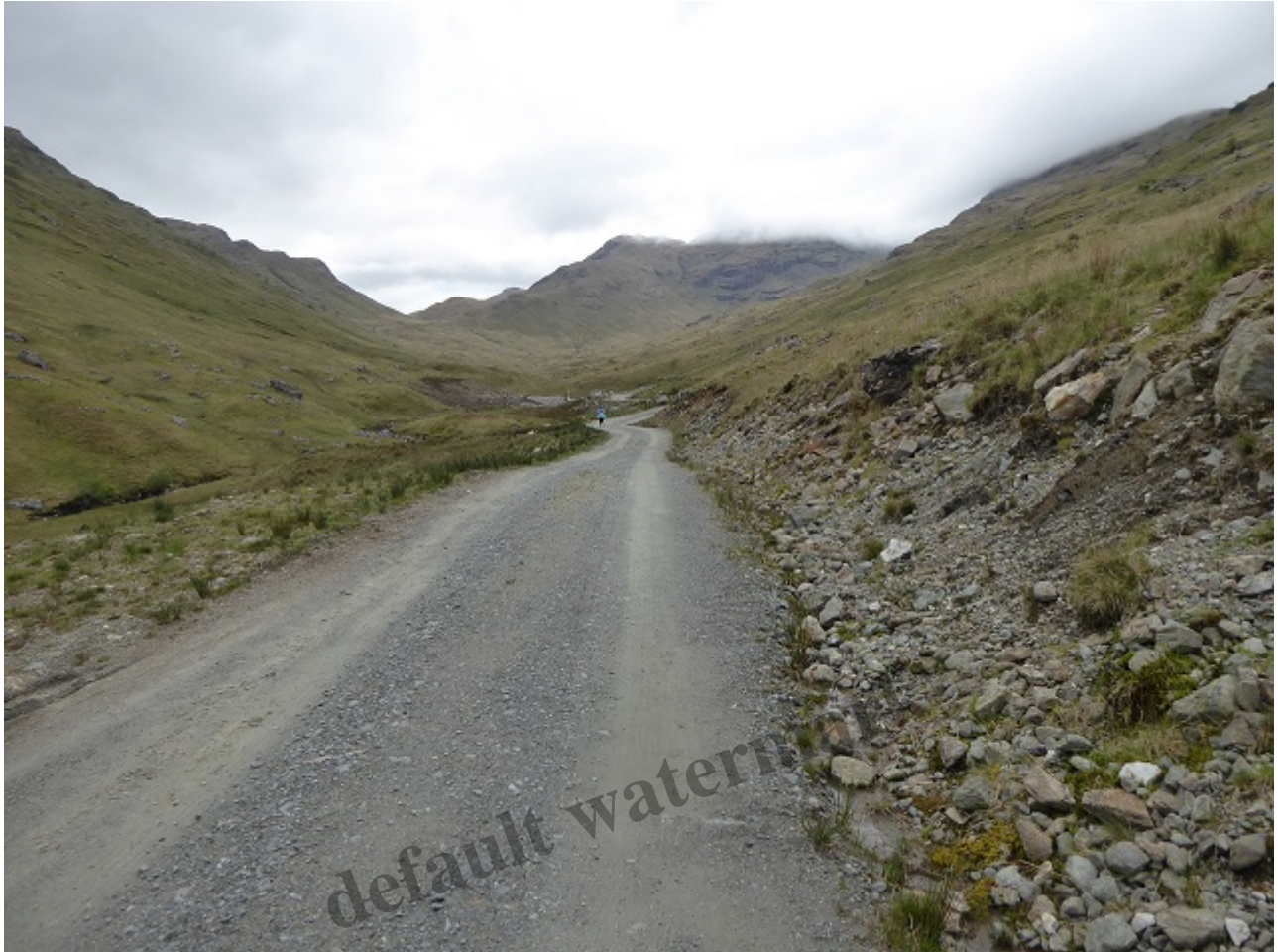
Looking towards hydro intake and Beinn a Chroin along final section of road. Note stones eroding out of unrestored bank on right.
