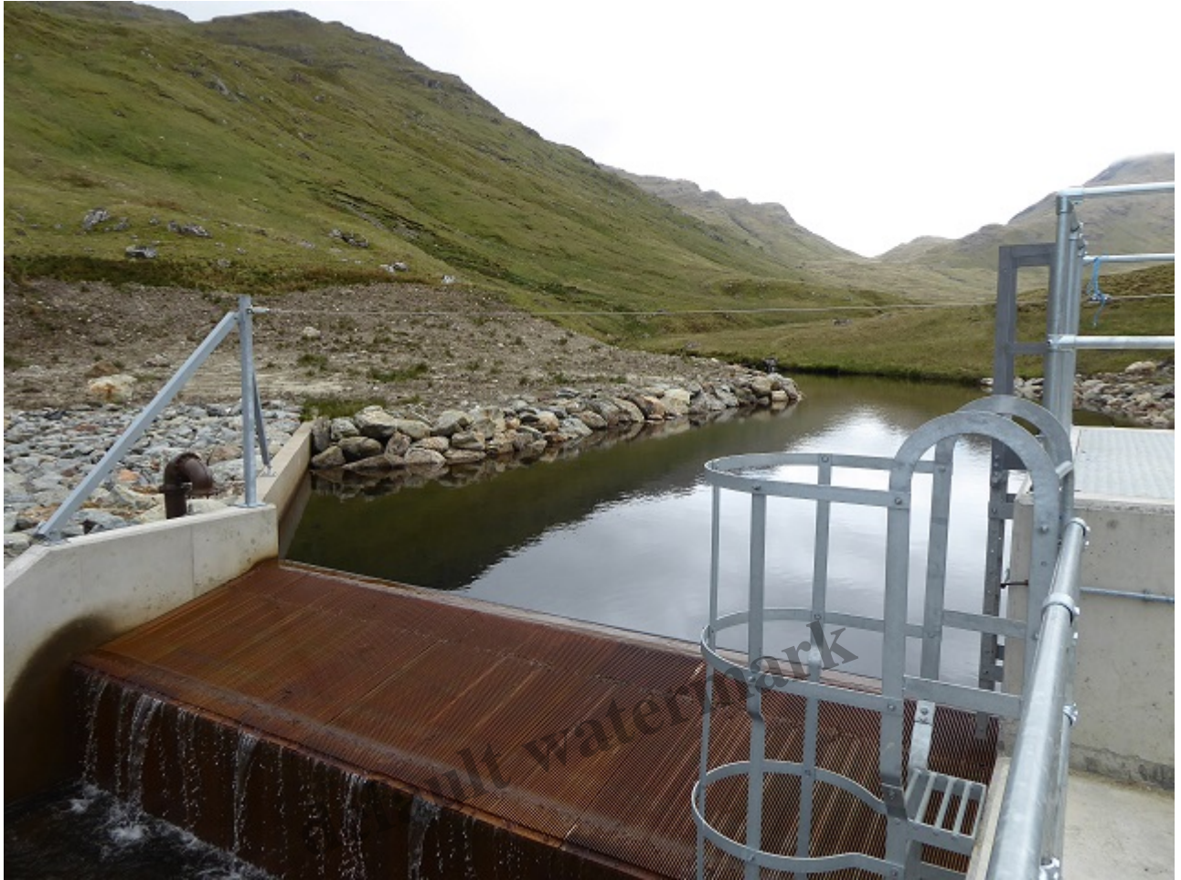
View upstream from hydro intake – at least the pipe on the left has been painted brown!
