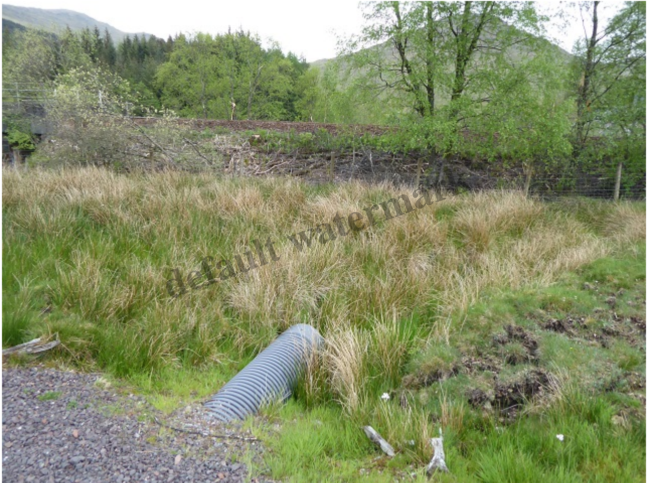
Protruding culvert on new section of footpath between the layby commonly used to access An Caisteal and Beinn a Chroin and the river Falloch
