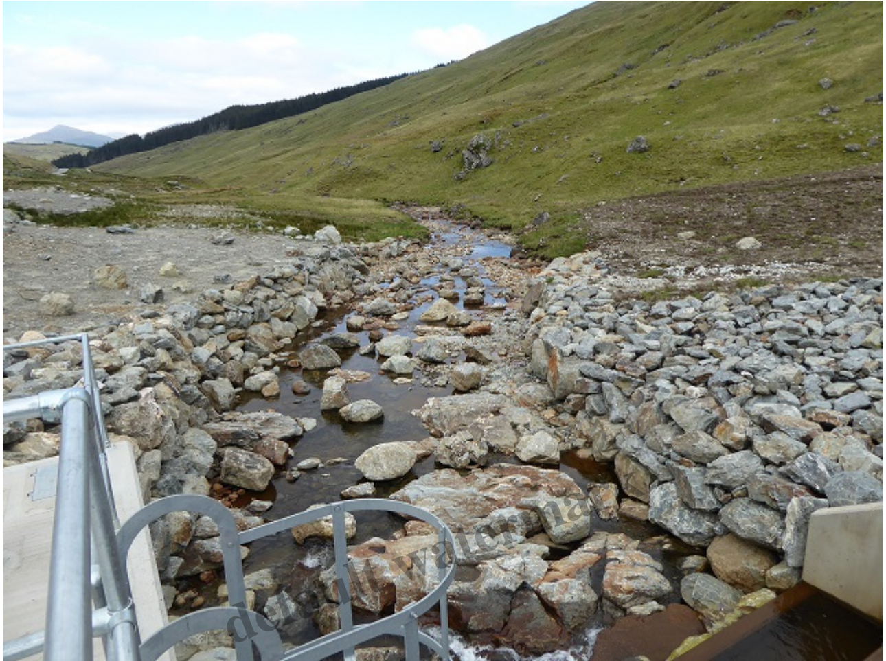
View downstream from hydro intake. The scattered boulders on the bare patch appear to be “landscaping”.
