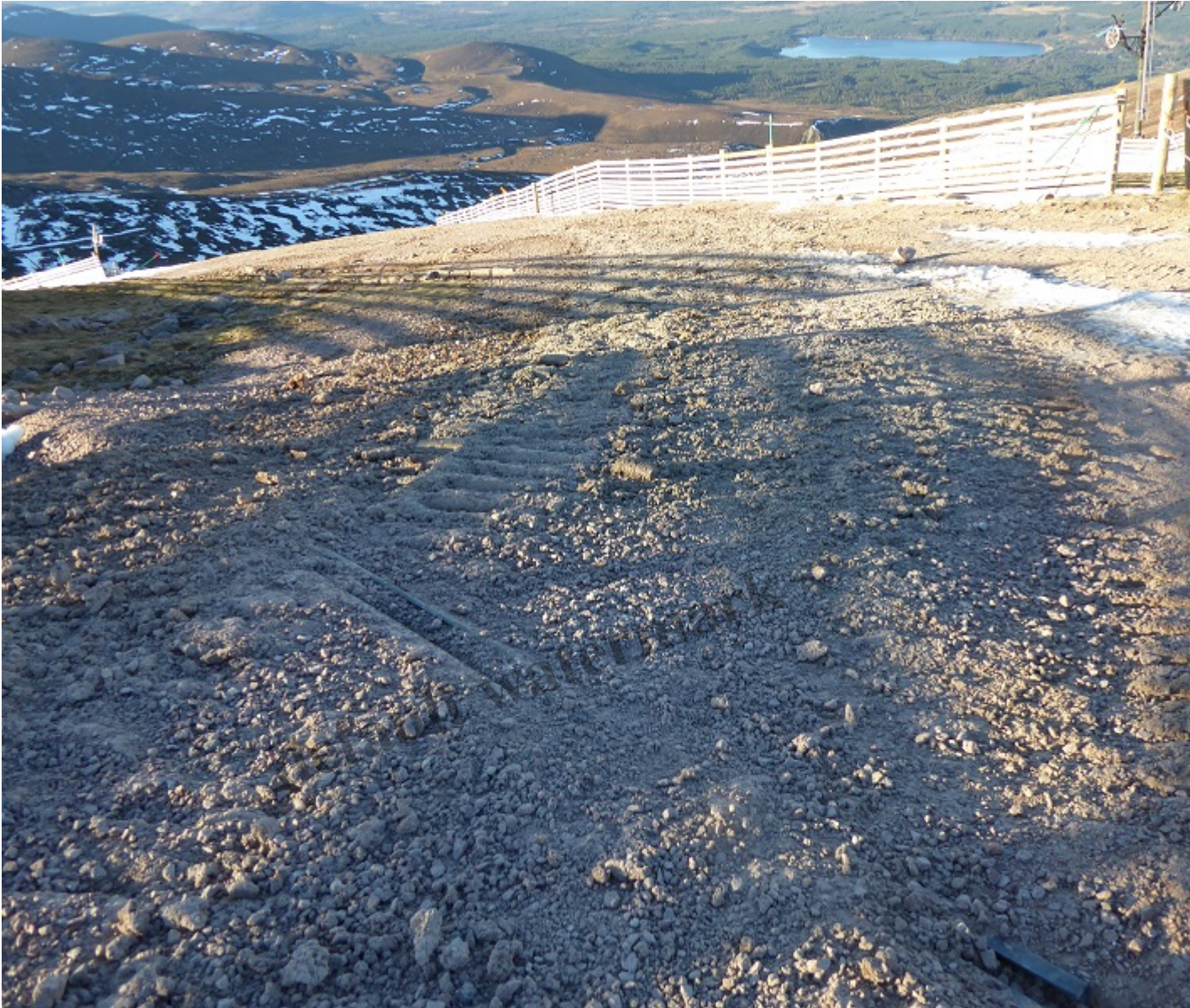
The start of the road down from the Ptarmigan showing the impact of vehicles on gravelly soils
