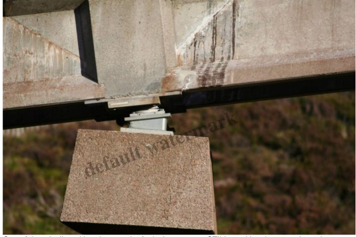
One of the misaligned bearings on the funicular – we are STILL awaiting the report into what caused this
