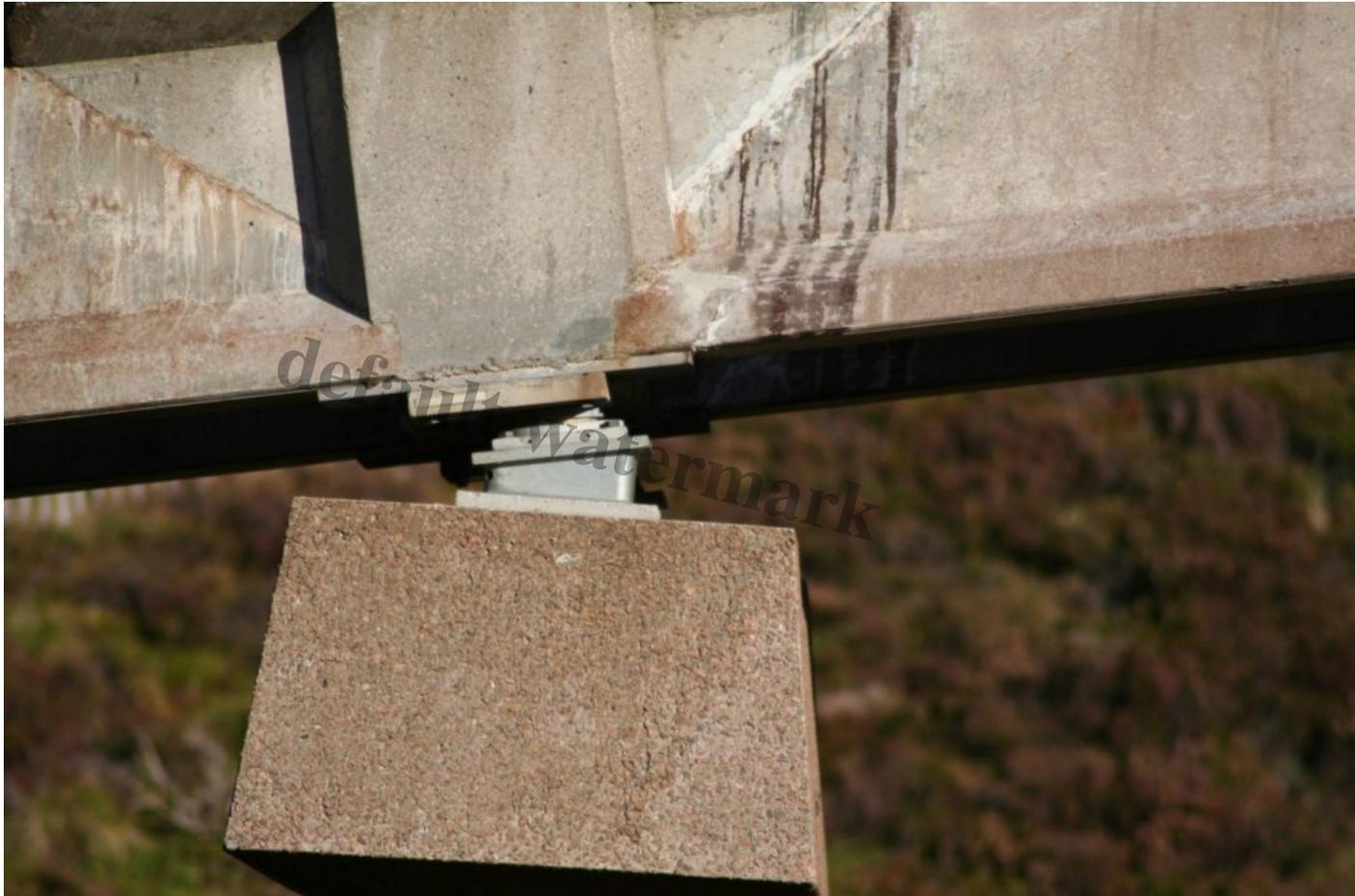
One of the misaligned bearings on the funicular â?? we are STILL awaiting the report into what caused this
