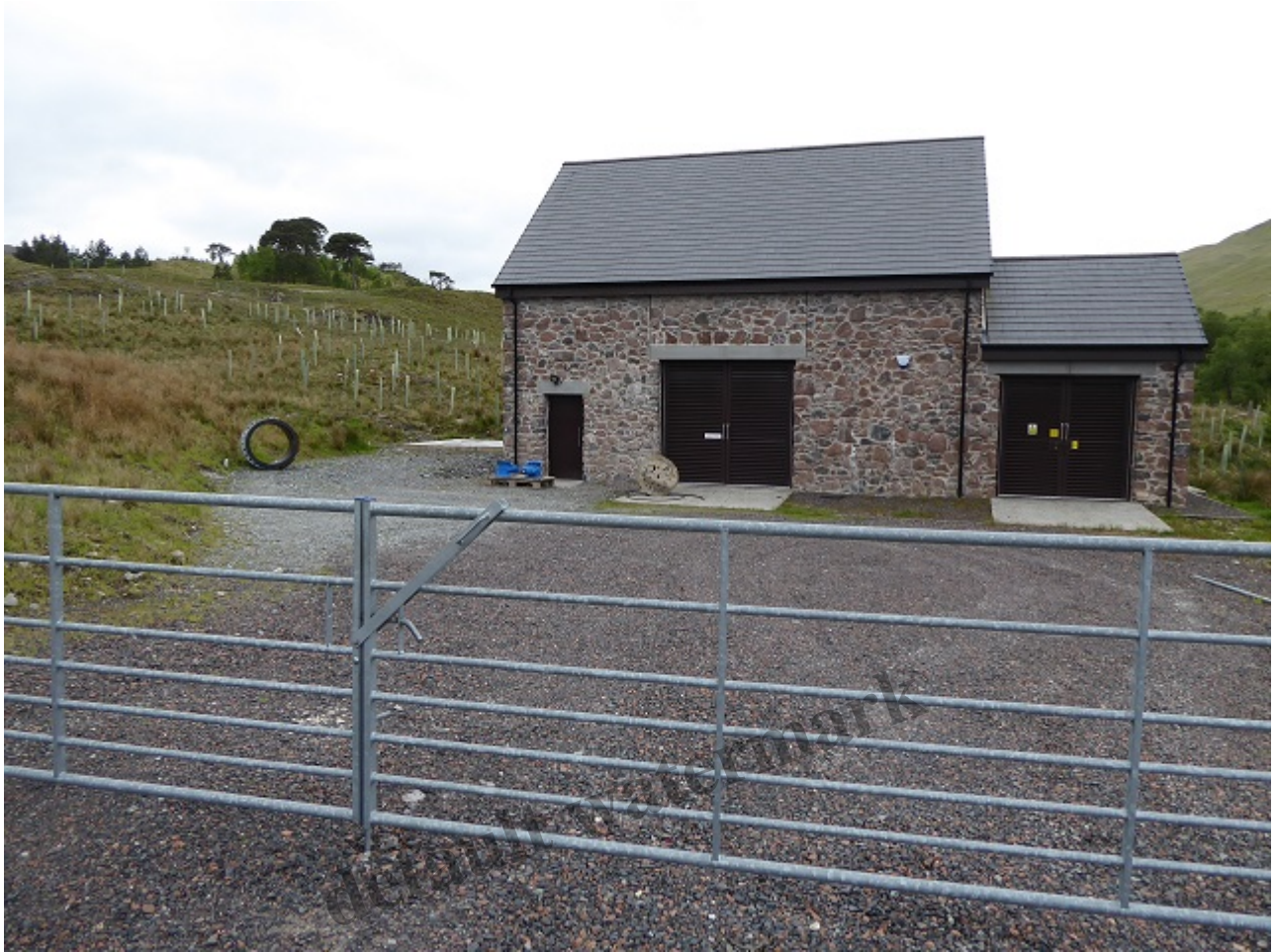
Upper Glen Falloch powerhouse May 2019 , with woodland planting all around and the eastern edge of the Caledonian Forest maybe 200m further back
