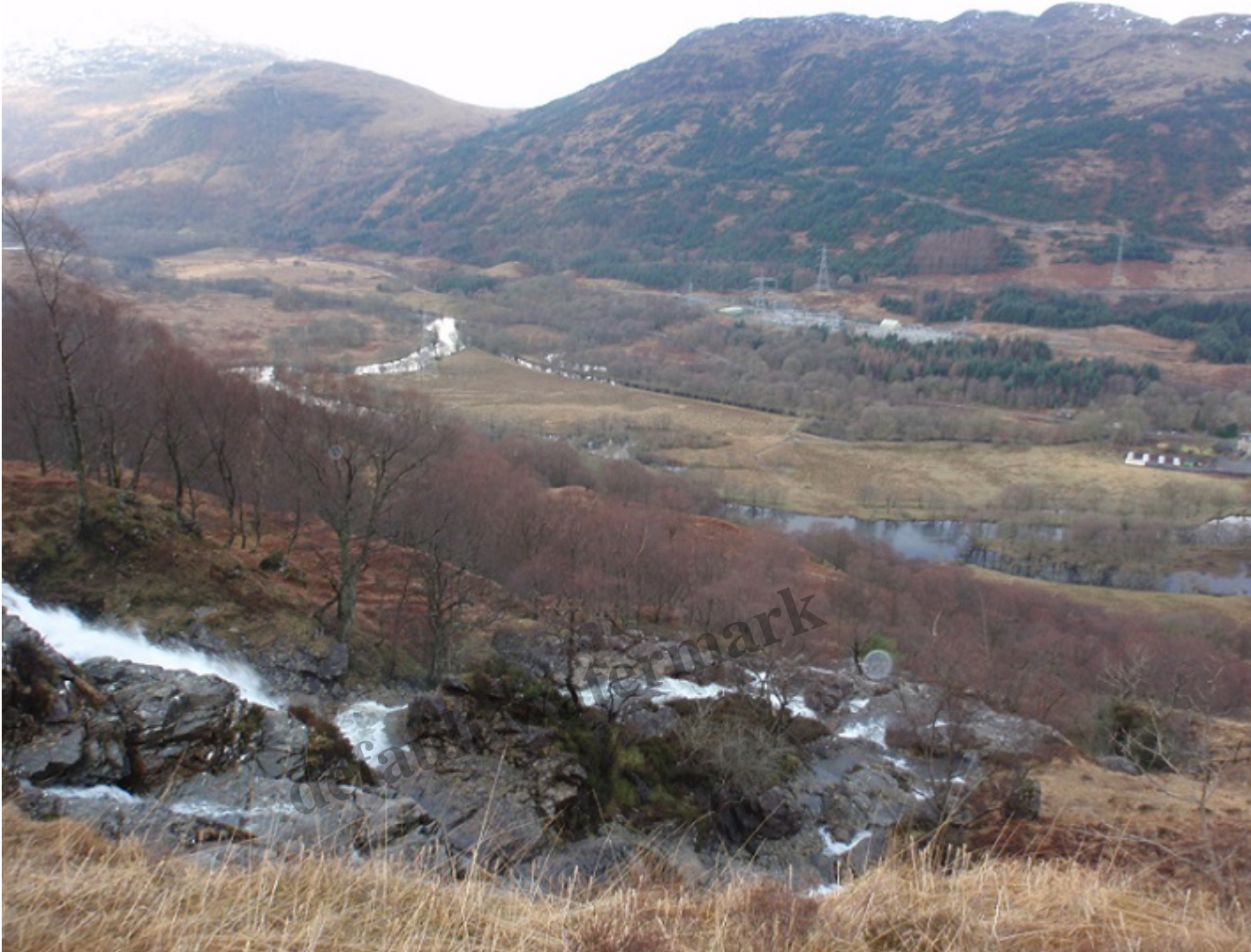
Garabal Hill viewed from Eagle Falls, with Ben Vorlich to the left. The road, clearly visible behind the electricity sub-station, which sits within the estate boundary, and pylons has created a great scar across its eastern flank.
