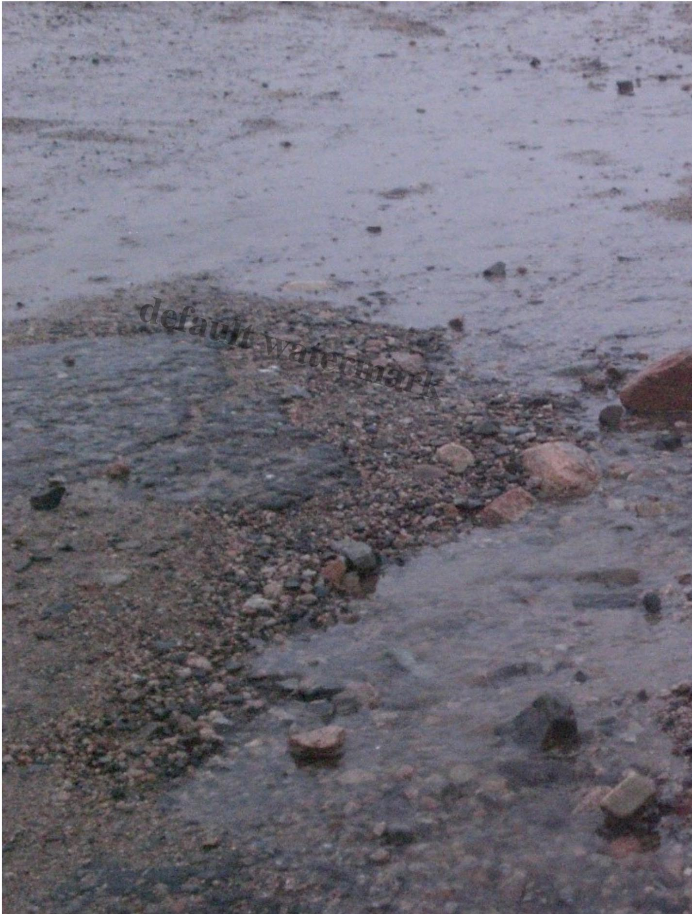
No drains to collect the rainwater so it flows downhill gathering volume and causing unnecessary damage
