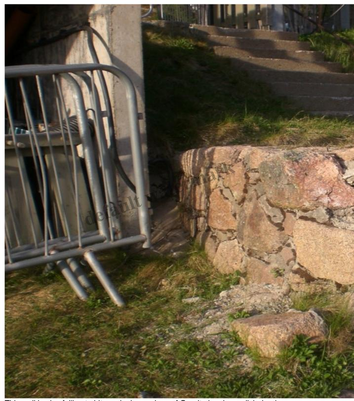
This wall is also falling to bits and a large piece of Granite has been dislodged.
