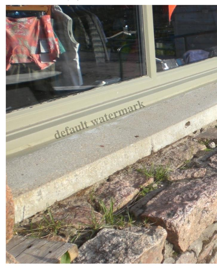
Vegetation on the window ledge outside the Retail Shop. That's exactly how the mortar gets loosene
