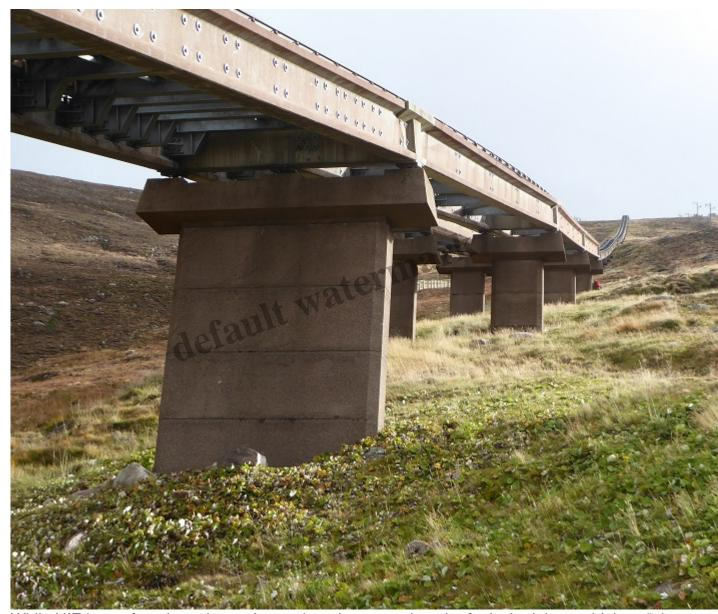
While HIE has refused to release the engineering report into the funicular it has said that "piers need strengthened and realigned, beams need strengthening, and all bearings need replaced on the piers
