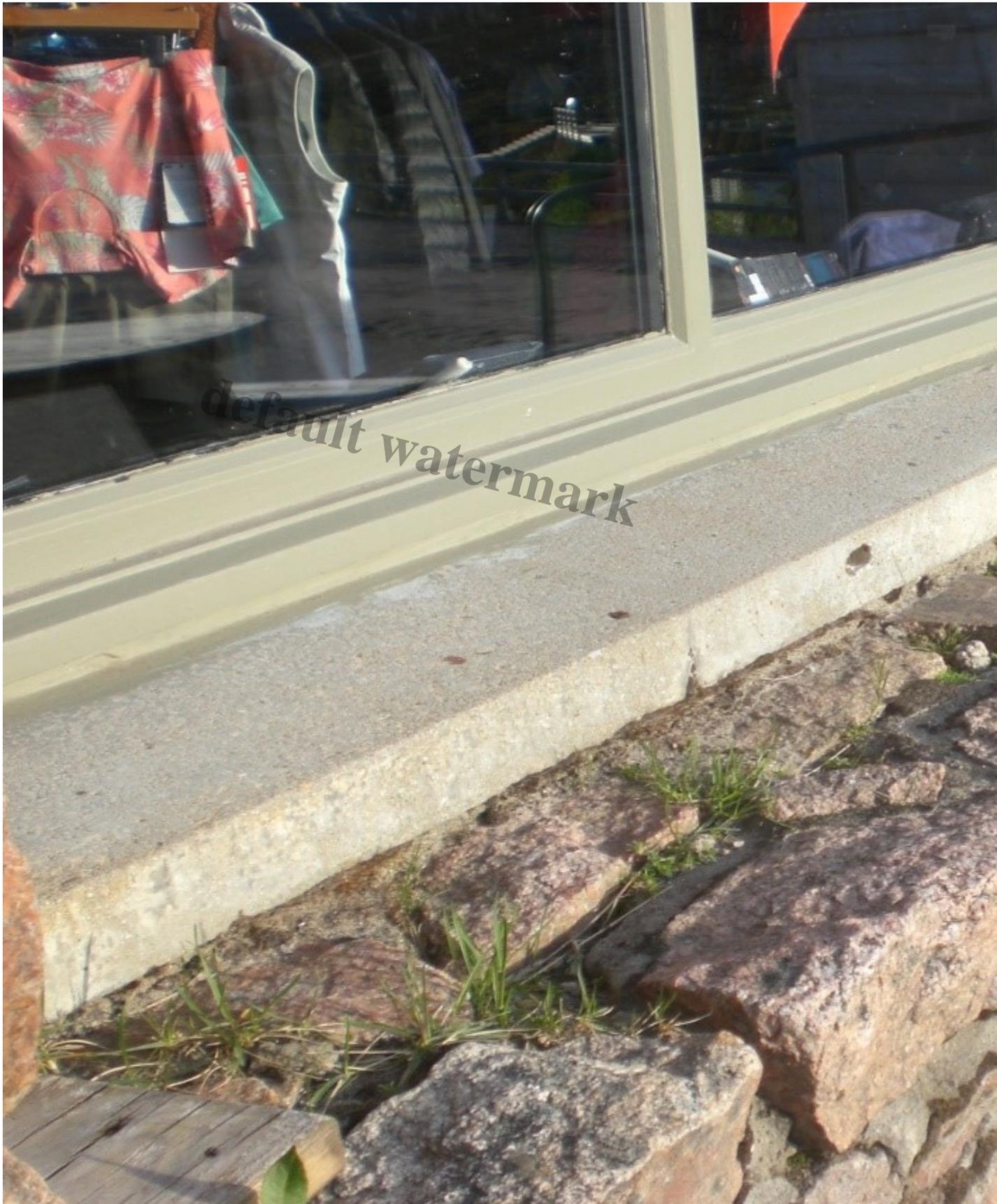
Vegetation on the window ledge outside the Retail Shop. That's exactly how the mortar gets loose on stonework.
