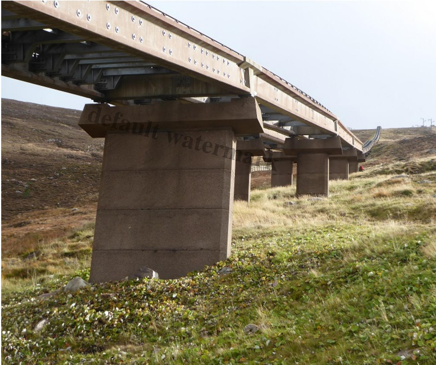
While HIE has refused to release the engineering report into the funicular it has said that *“piers need strengthened and realigned, beams need strengthening, and all bearings need replaced on the piers*
