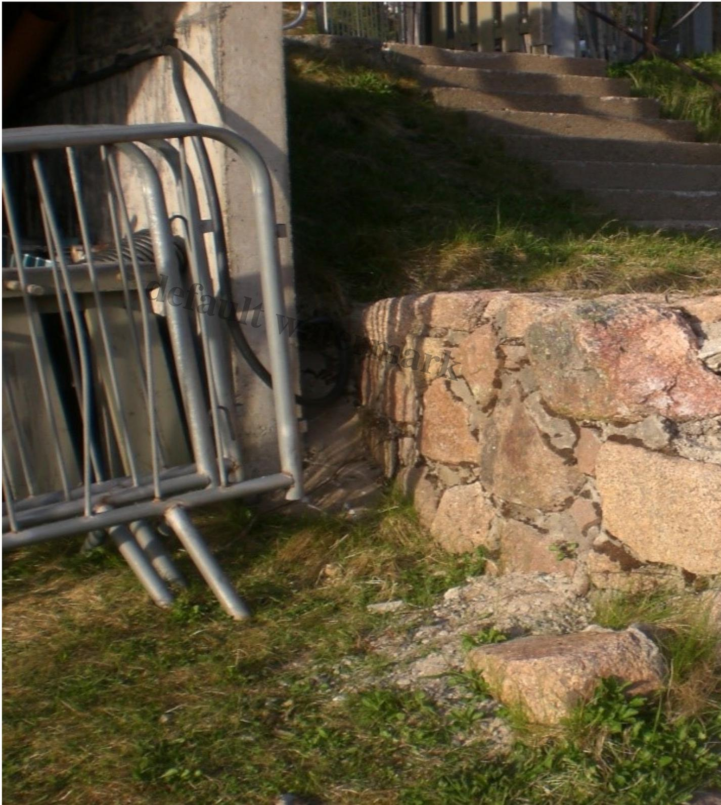
This wall is also falling to bits and a large piece of Granite has been dislodged.
