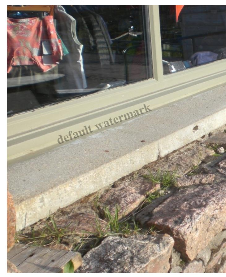
Vegetation on the window ledge outside the Retail Shop. That's exactly how the mortar gets loosened
