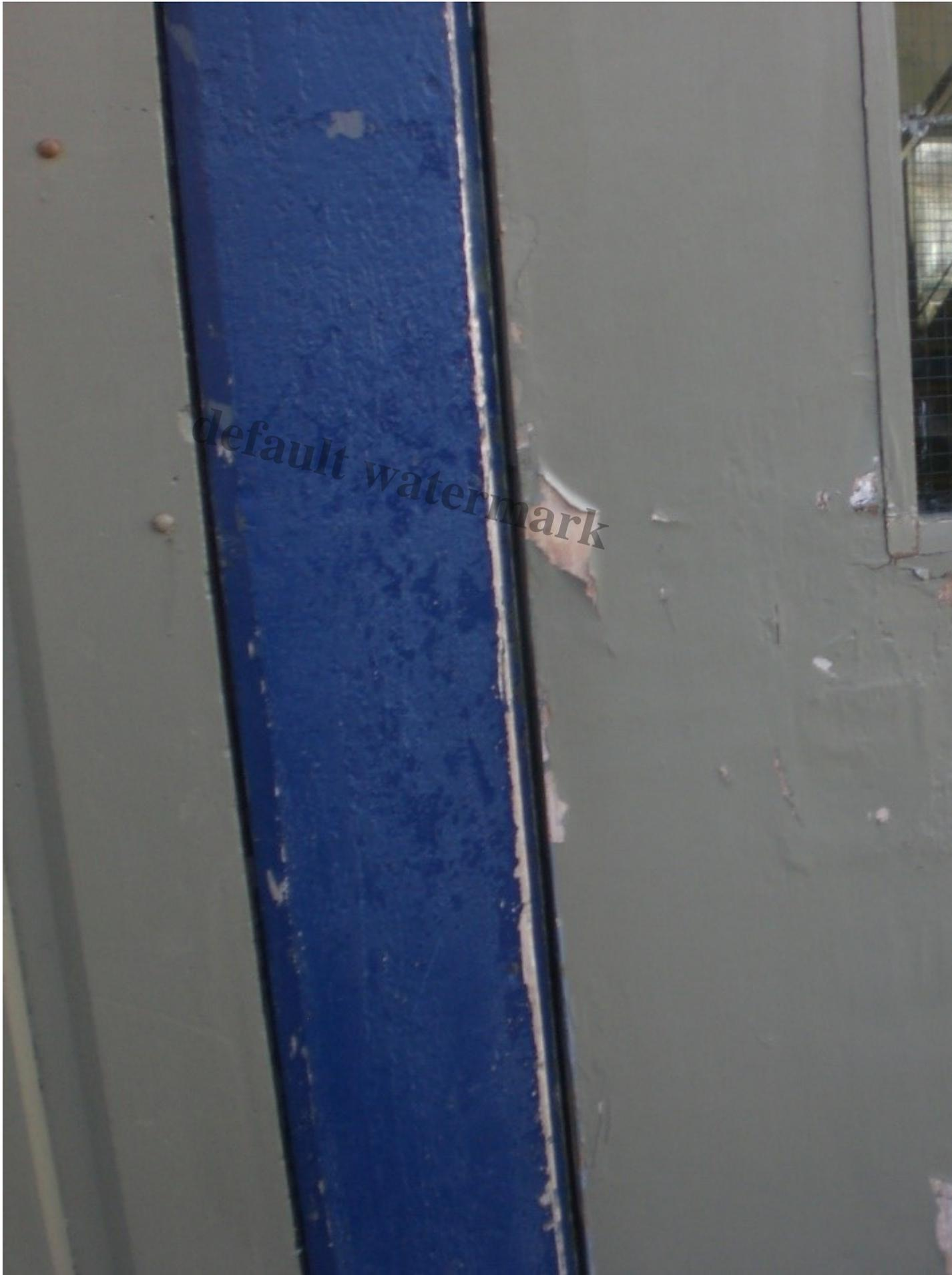
The Fire Exit from the café. The door is rotten and should be replaced immediately.
