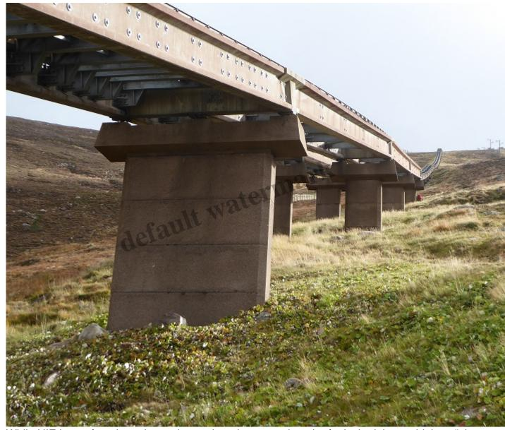
While HIE has refused to release the engineering report into the funicular it has said that "piers neestrengthened and realigned, beams need strengthening, and all bearings need replaced on the piers
