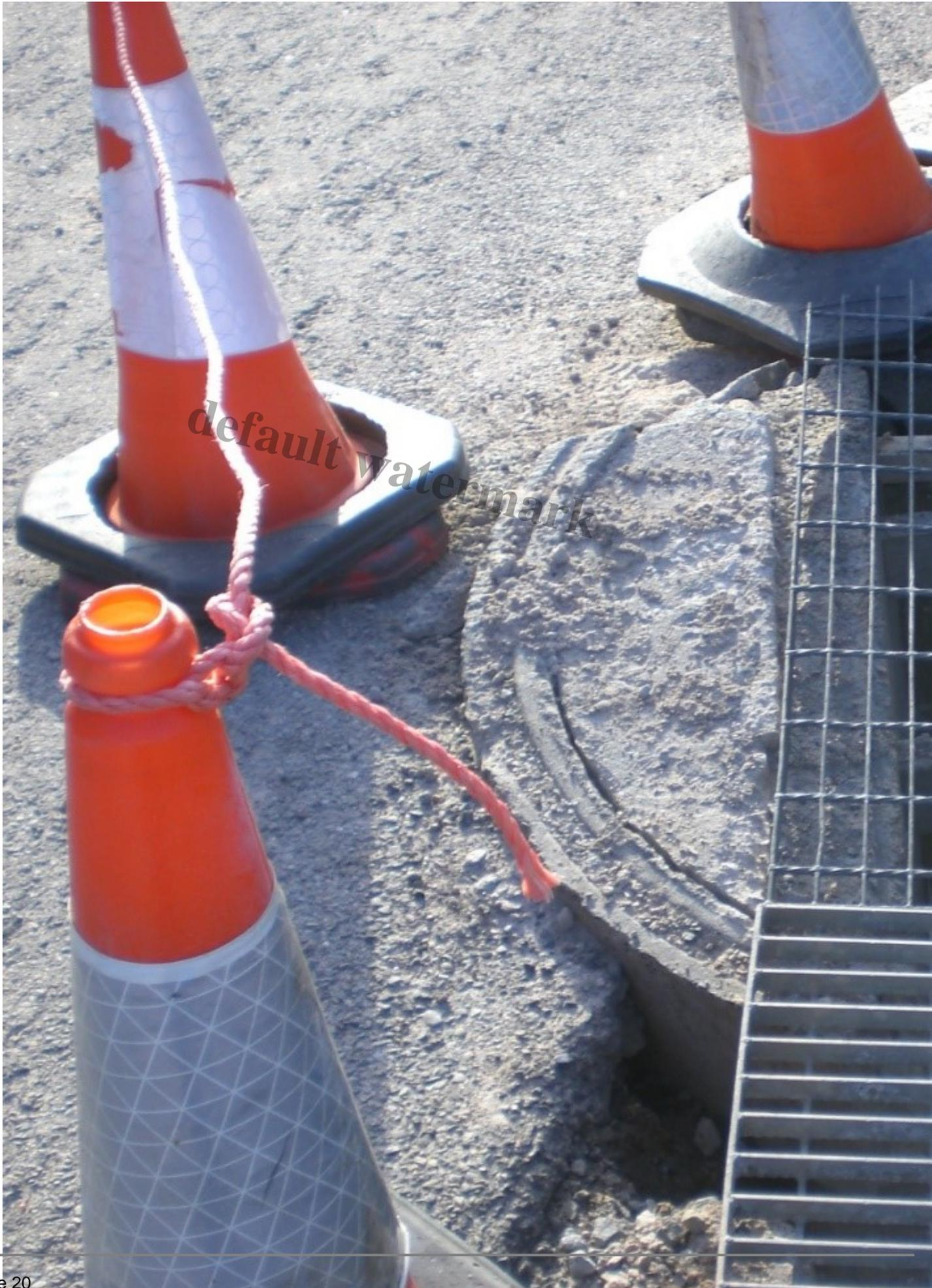
Broken drain between the Daylodge and the Funicular Station
