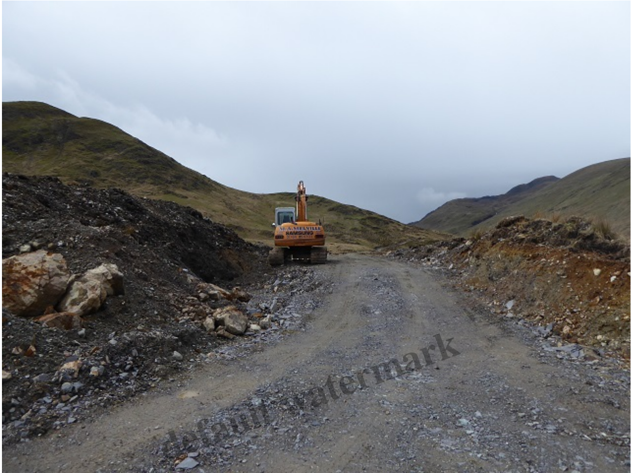
The new road starts with a cutting
