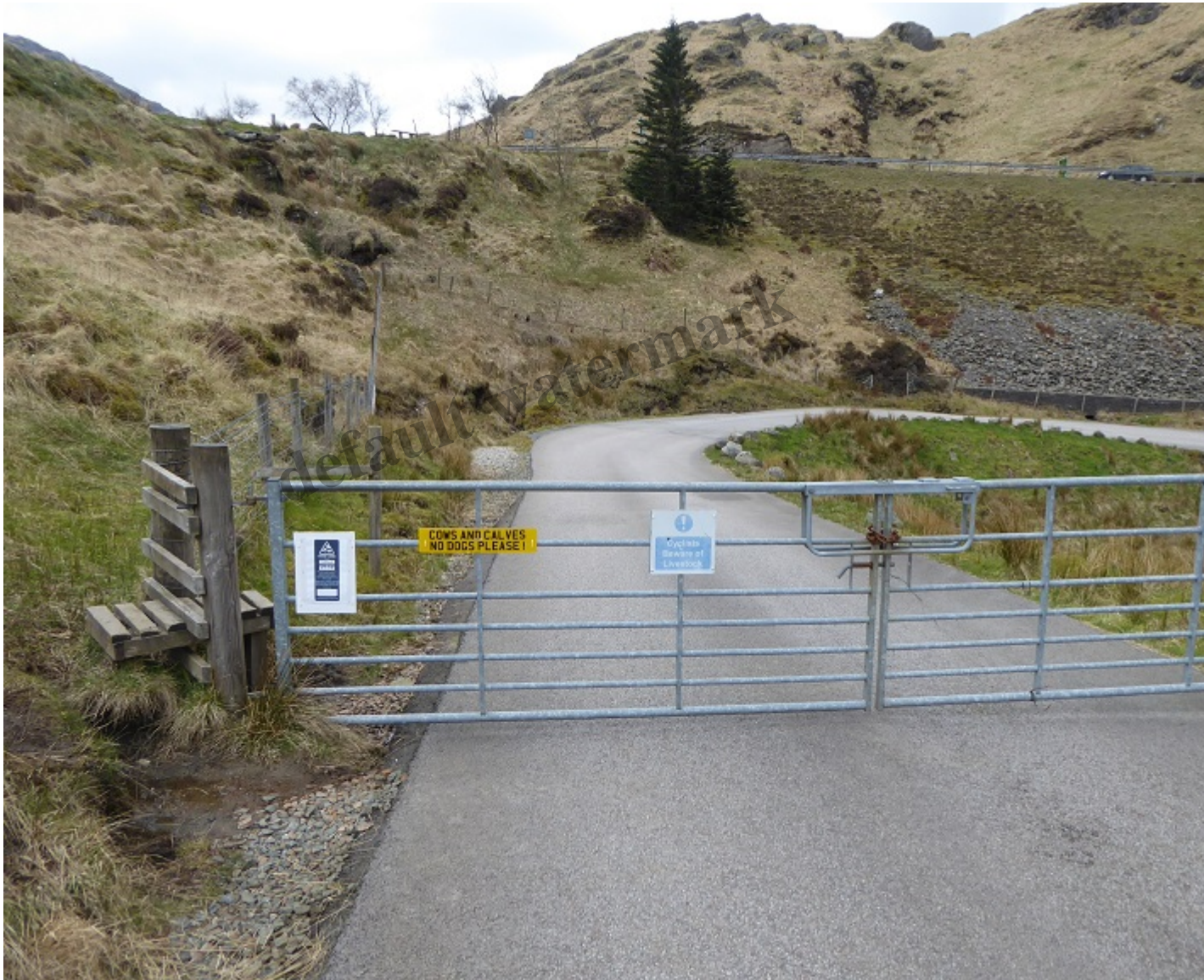
Locked gate on former military road just below the Rest and Be Thankful with the A83 visible above
