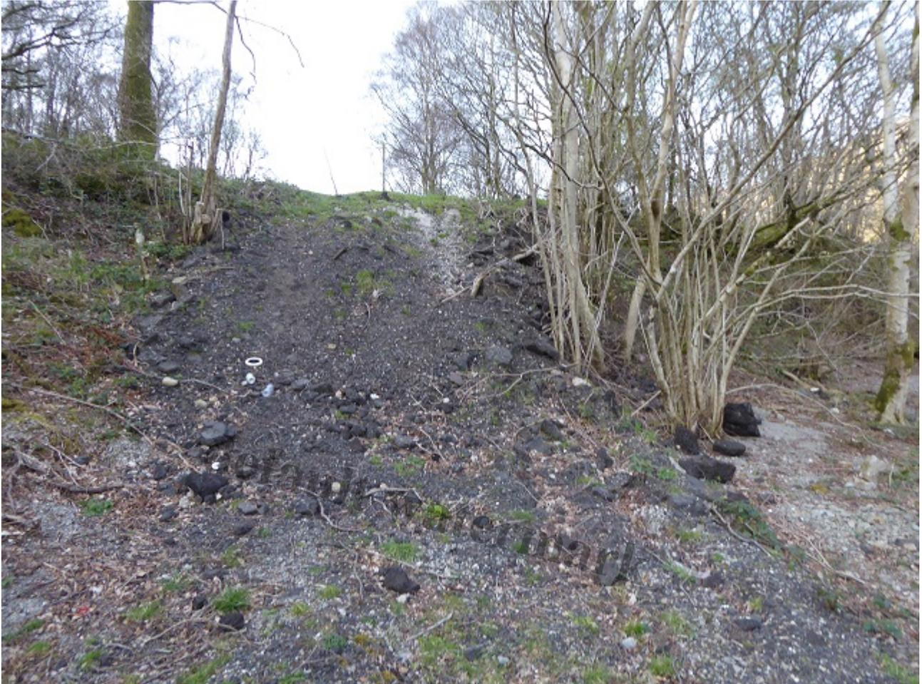
Old tarmac has been used to create a vehicle ramp down to the Loch shore to facilitate the creation of the new embankment
