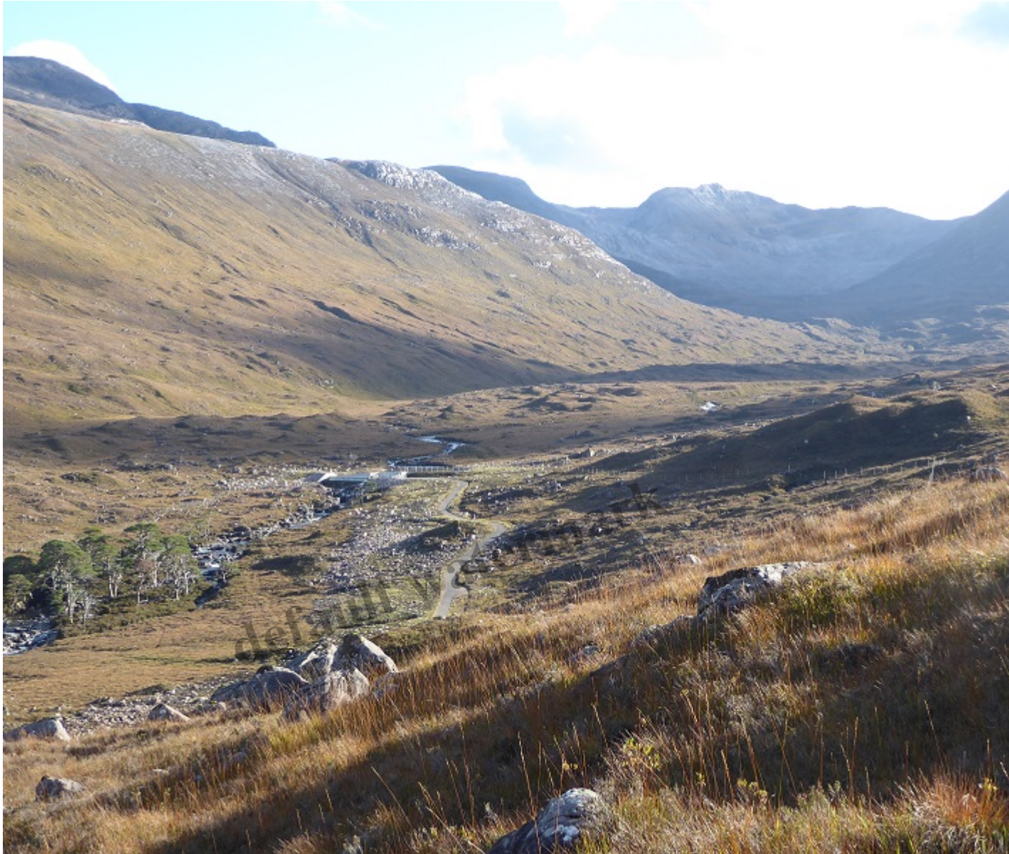
Intake on the Glen Grudie hydro scheme, Torridon. Even if there was no track here and the pipeline better restored the intake would still be visible from afar
